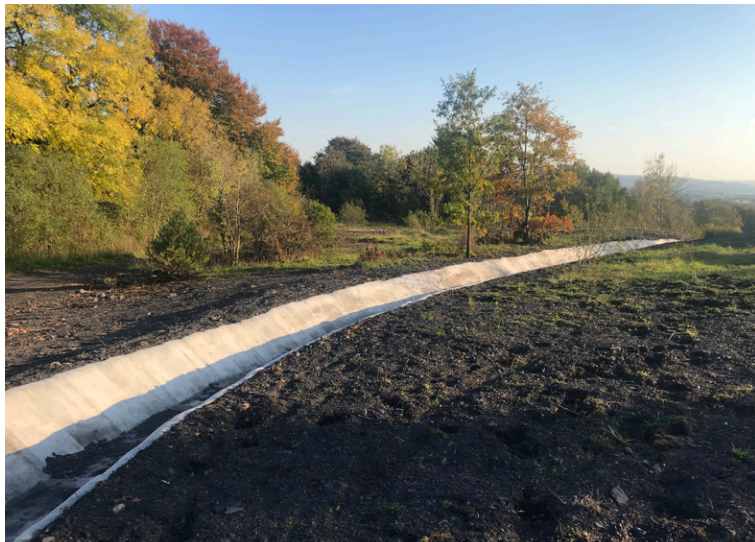
Anchor trenches were backfilled following hydration of CC
