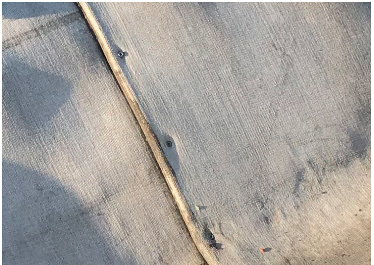
CC jointed using screws
