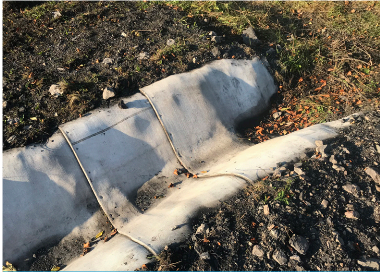
Material termination at source of natural water channel
