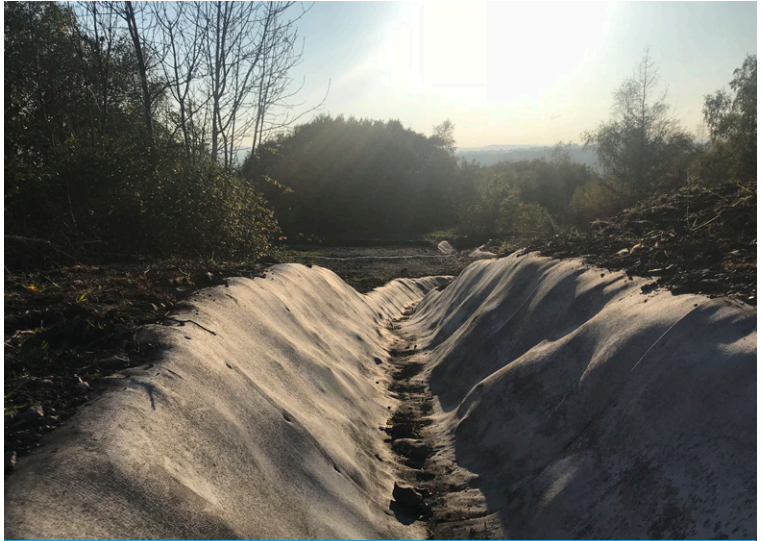
CC allowed installation with minimal groundwork & conforms to channel profile
