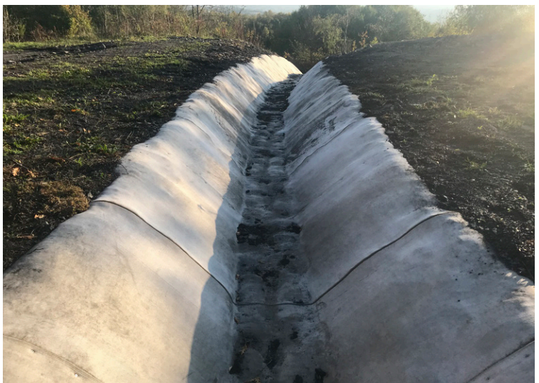
Section of channel lined using transverse layout
