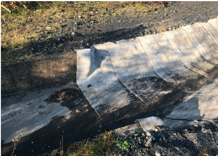
Termination of CC lined channels into existing concrete channel
