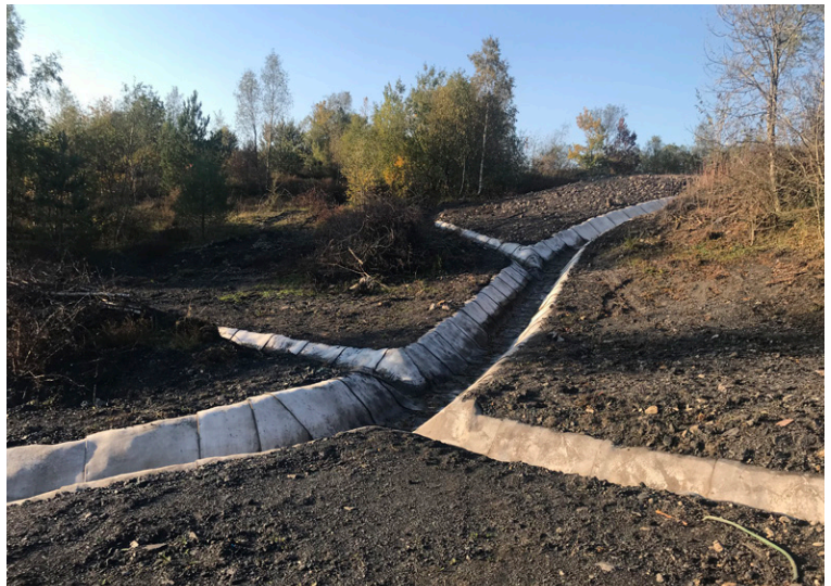
Section of drainage channel system created and lined for water management
