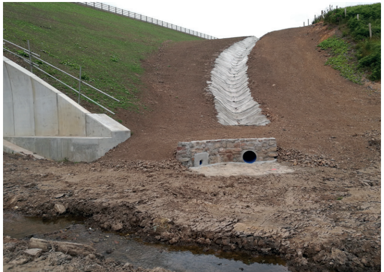
CC terminated into culvert headwall behind diversion channel
