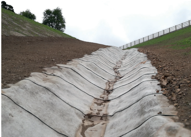
CC installed on steep slope
