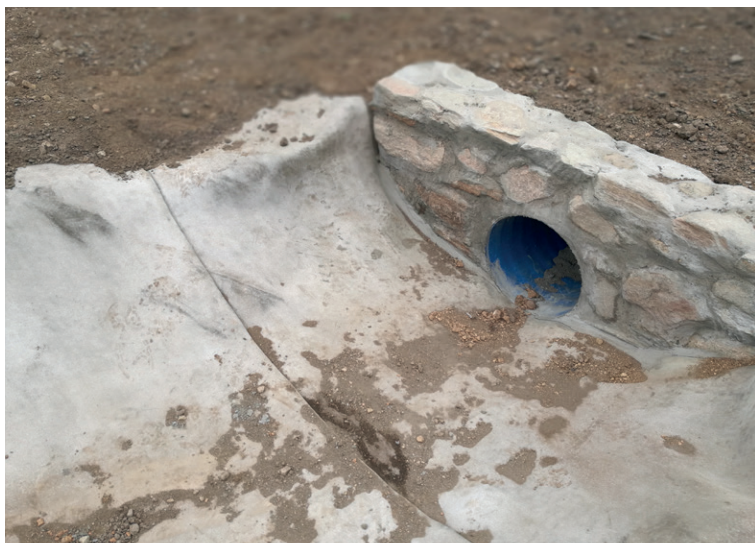
CC installed around headwall
