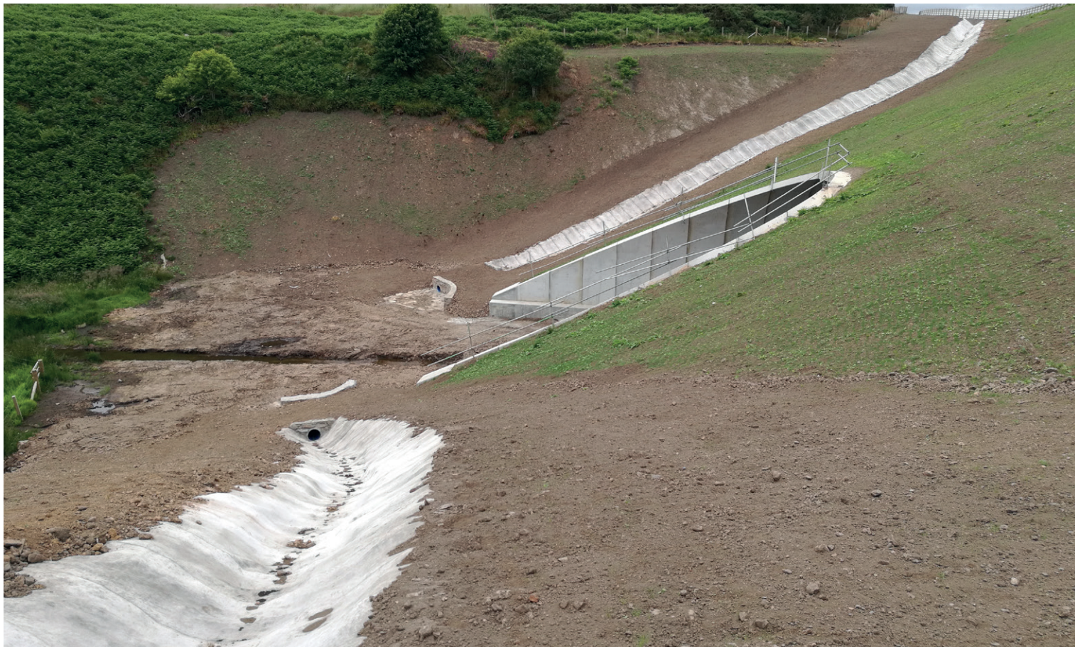
Completed CC lined drainage channels
