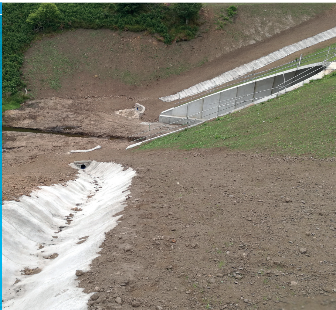
Completed channel lining installation in the AWPR-BT Fastlink Section
