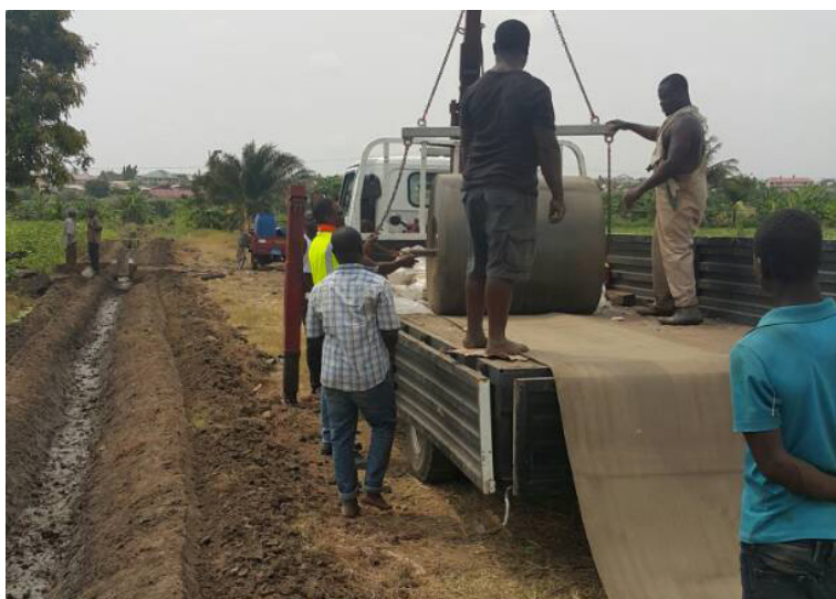
The CC was delivered on a bulk roll, unrolled and cut to length
