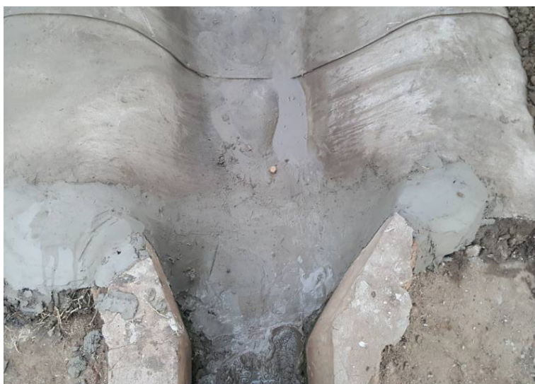
Grout was used to seal the ends of the CC at gates transitions
