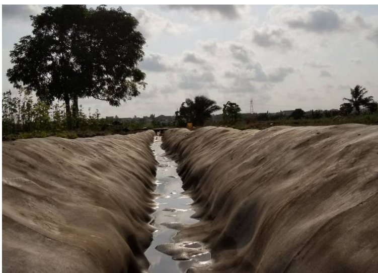
Completed transverse section post-hydration
