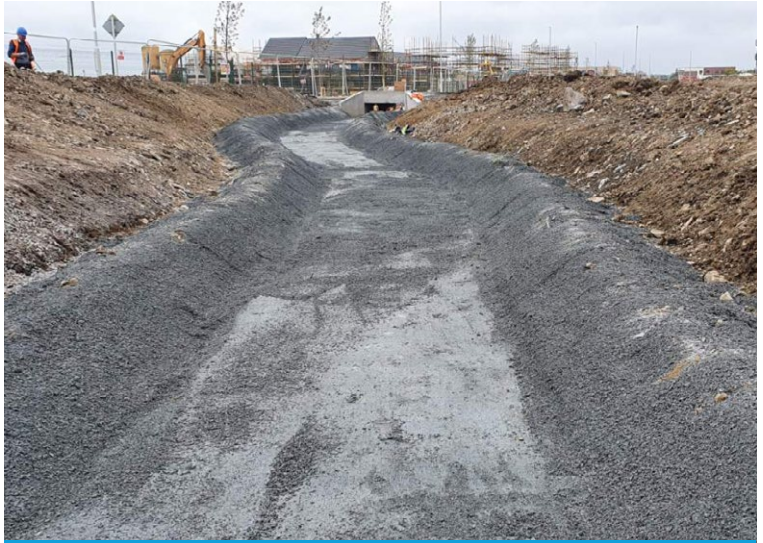
Crushed aggregate compacted for smooth substrate
