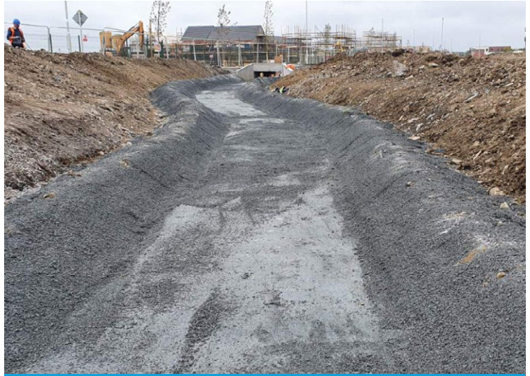
Crushed aggregate compacted for smooth substrate
