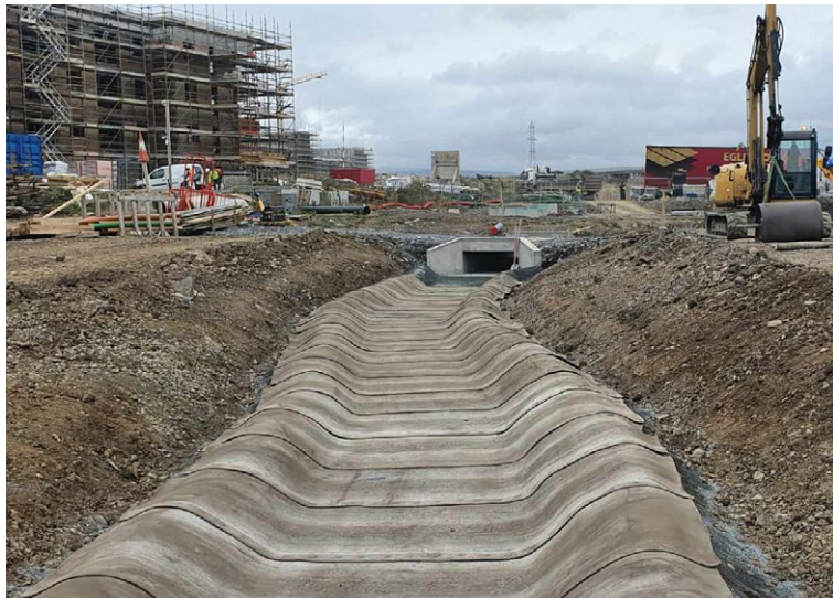
CCT2™ laid transversely across channel
