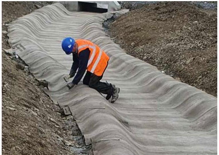
Leading edges terminated into anchor trenches with J-pegs
