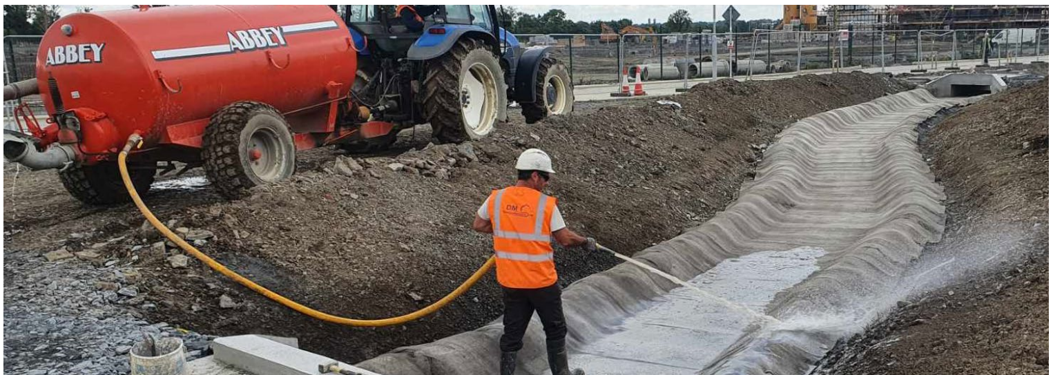
CCT2™ hydrated using hose and water bowser
