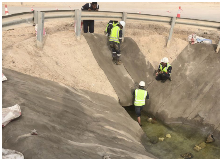
Vertical lengths of CC installed at the end of the channel
