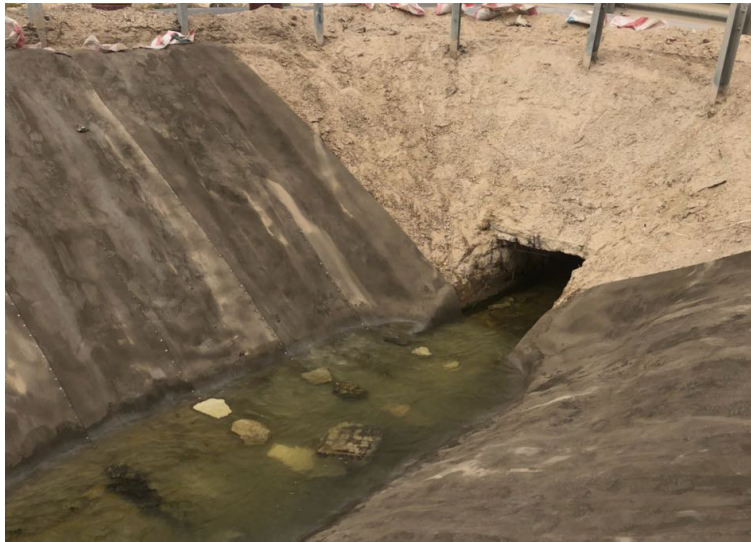
CC lengths were laid transversely across channel profile
