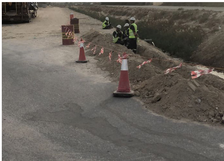
Anchor trenches were prepared using shovels where required
