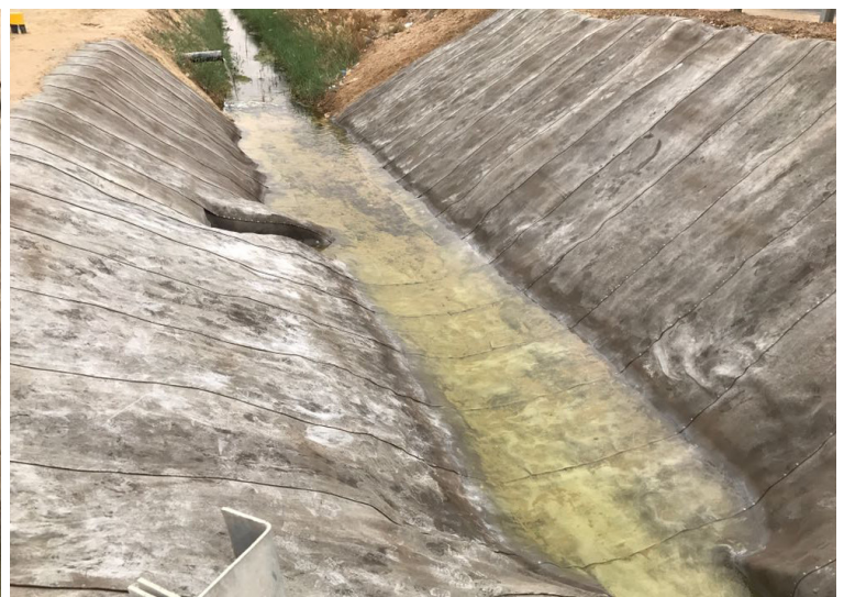
Completed CC lined channel section following hydration
