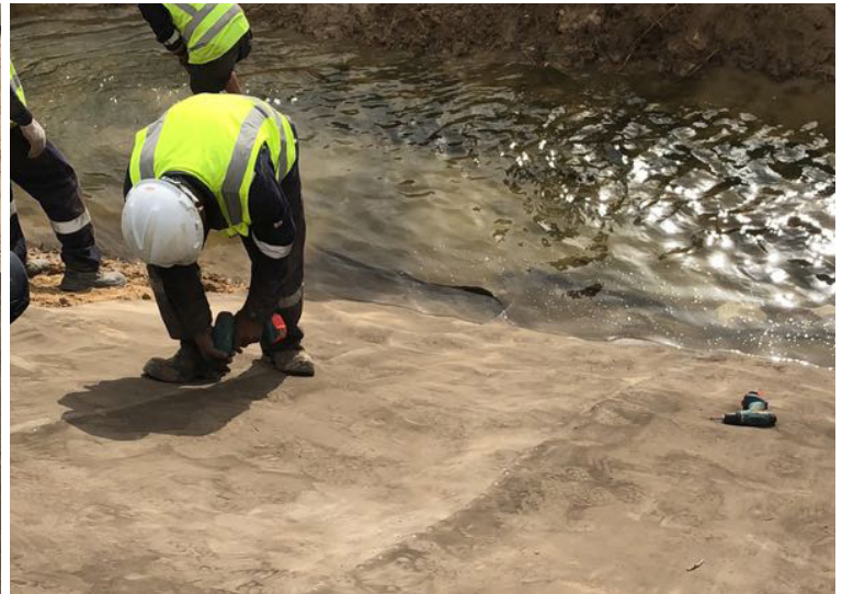
Overlapping joints were jointed with stainless steel screws
