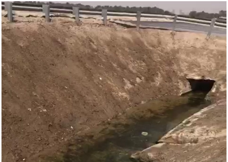
The channel was excavated and regraded prior to installation
