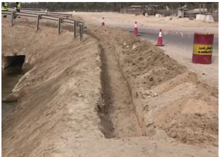
Prepared anchor trenches
