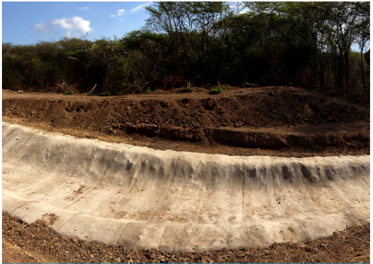
CC8 laid transversely and anchor trenched
