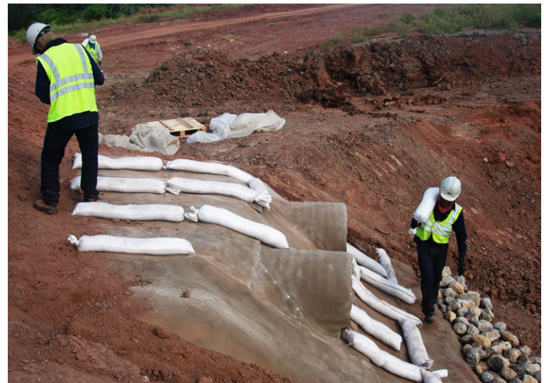
Sandbags were used to provide compression during setting
