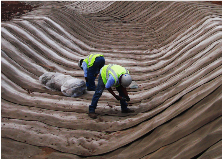
The overlaps were sealed and screwed
