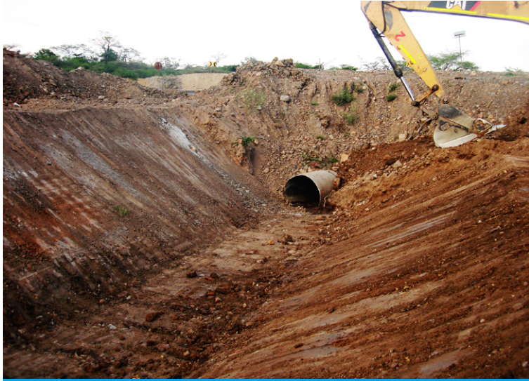
The ditches were cleared of debris and graded
