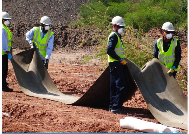
CC8 was cut to length and then positioned
