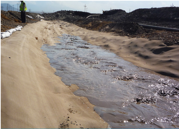
CC8 laid longitudinally
