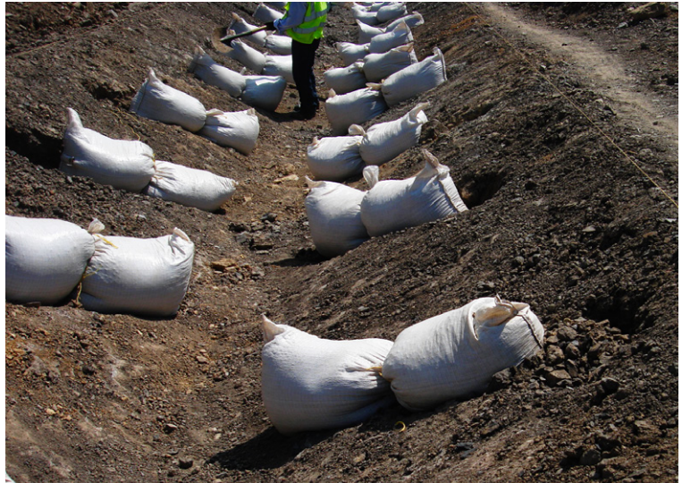
Placement was at 2m intervals (offset) to create a meandering route
