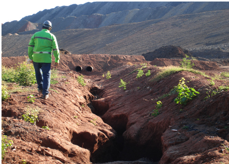
Severe vertical erosion and vegetation growth
