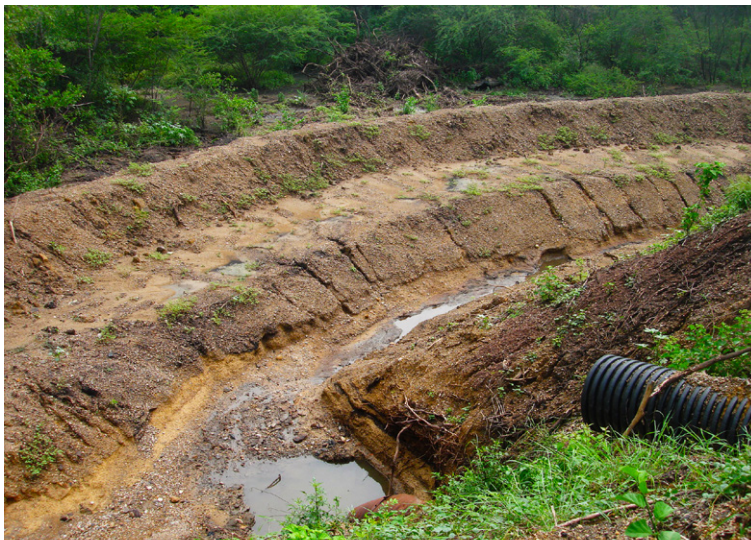
Slope and ditch erosion, cracking and vegetation
