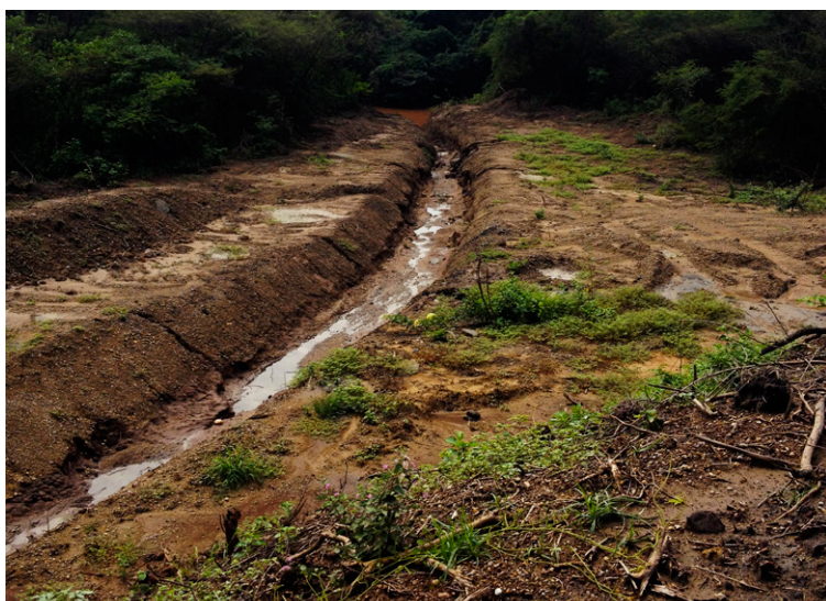
Cracking and undercutting of ditch walls
