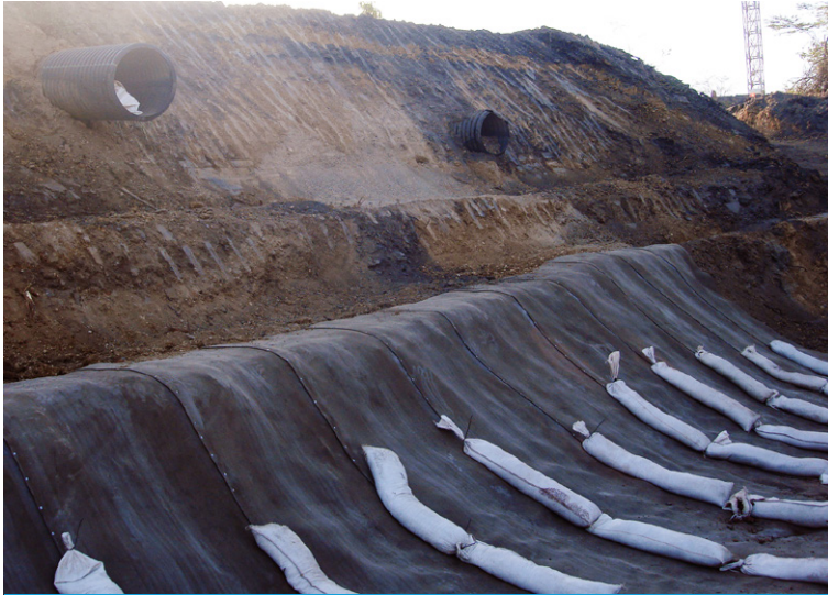
The ditch below the slope was lined with CC8
