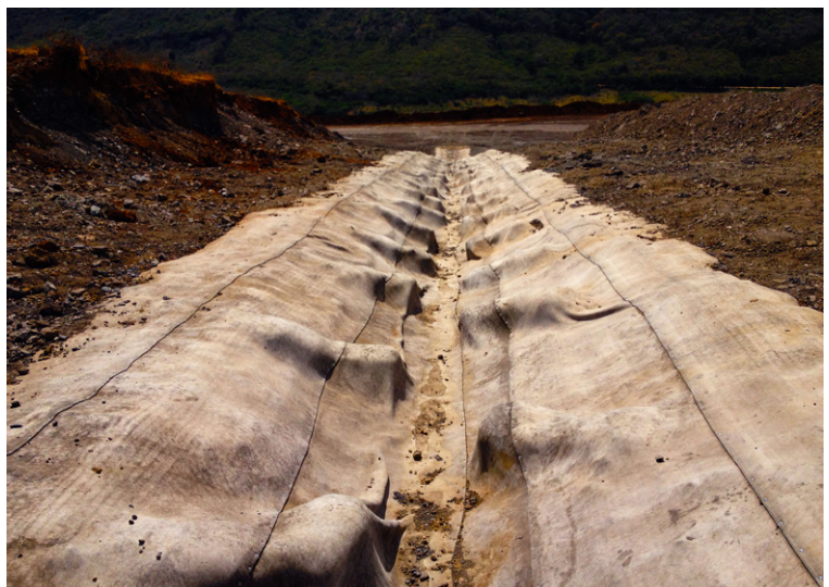
The finished ditch with baffling
