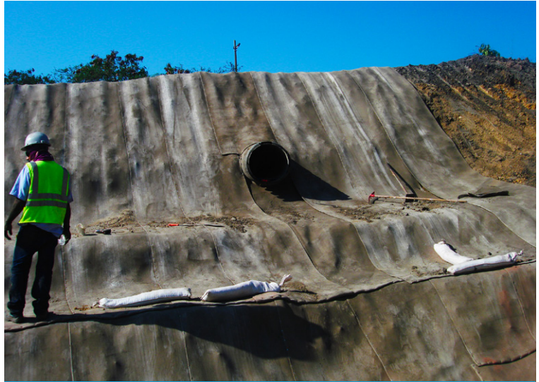
This was then overlapped with the CC8 being used for slope protection
