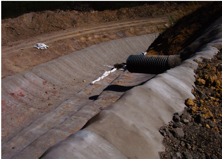
The CC8 was anchor trenched at the top of the slope
