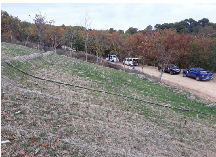
Biodegradable net installed on harvested slope
