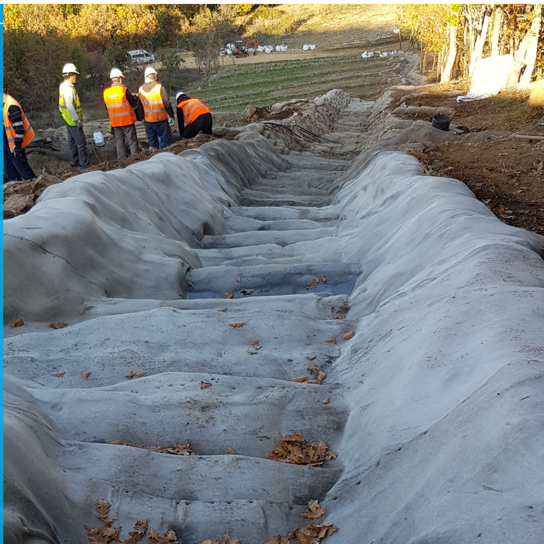
Completed section of CC channel lining installation
