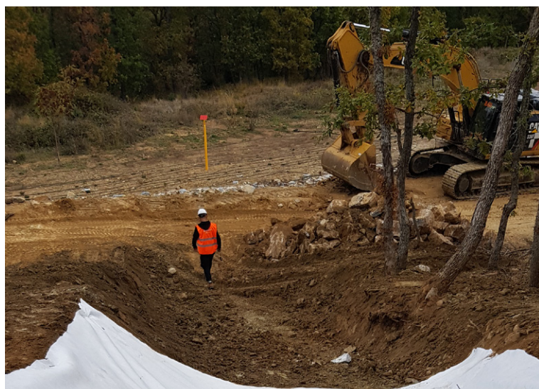
Excavating the channel
