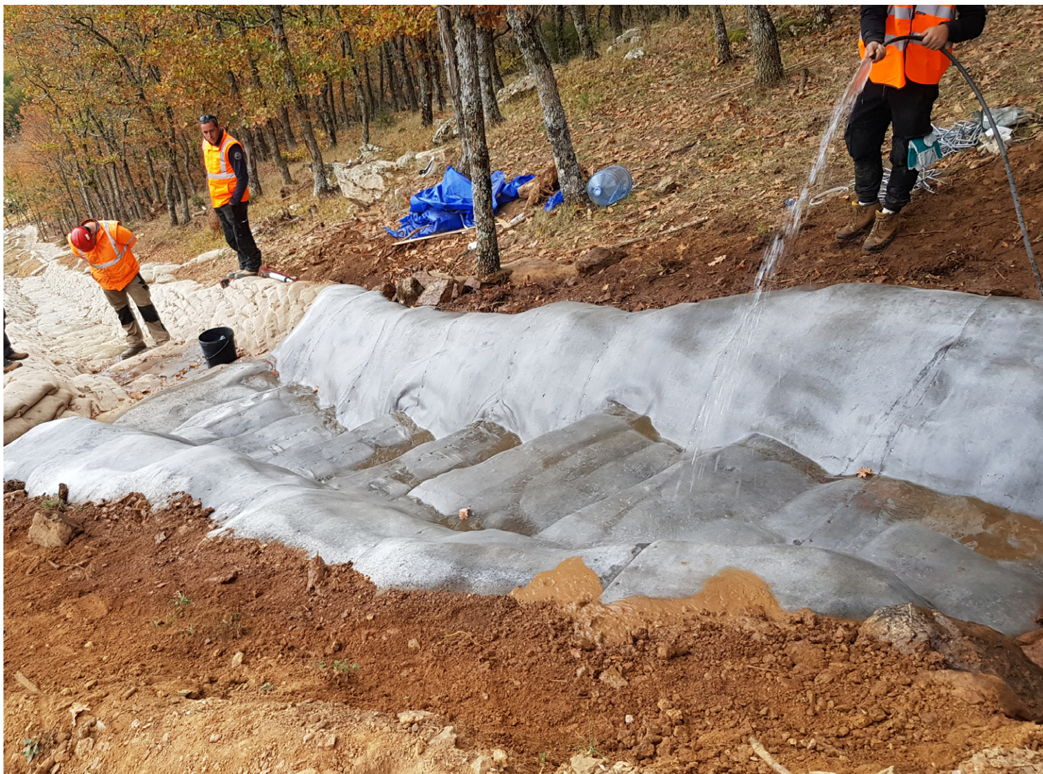
Completed section of CC installation
