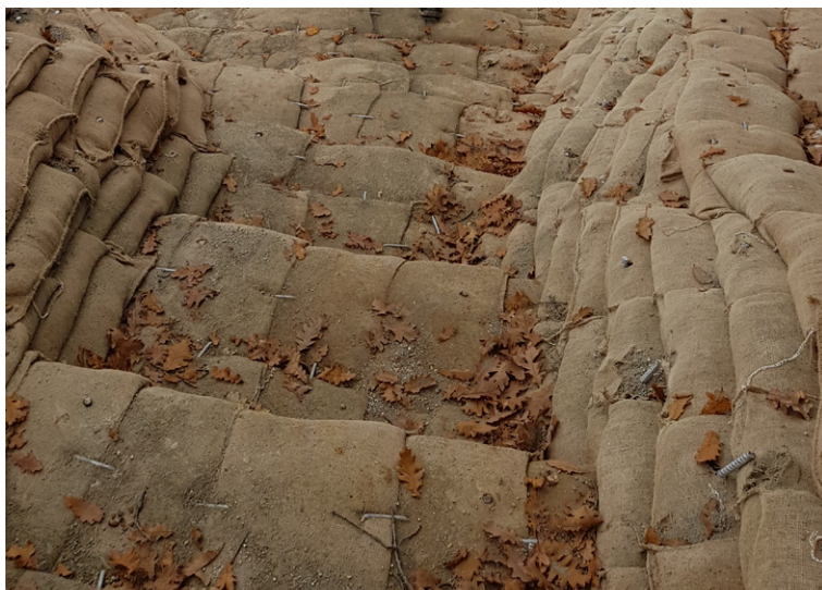
Sandbags jointed and fixed to substrate using anchors
