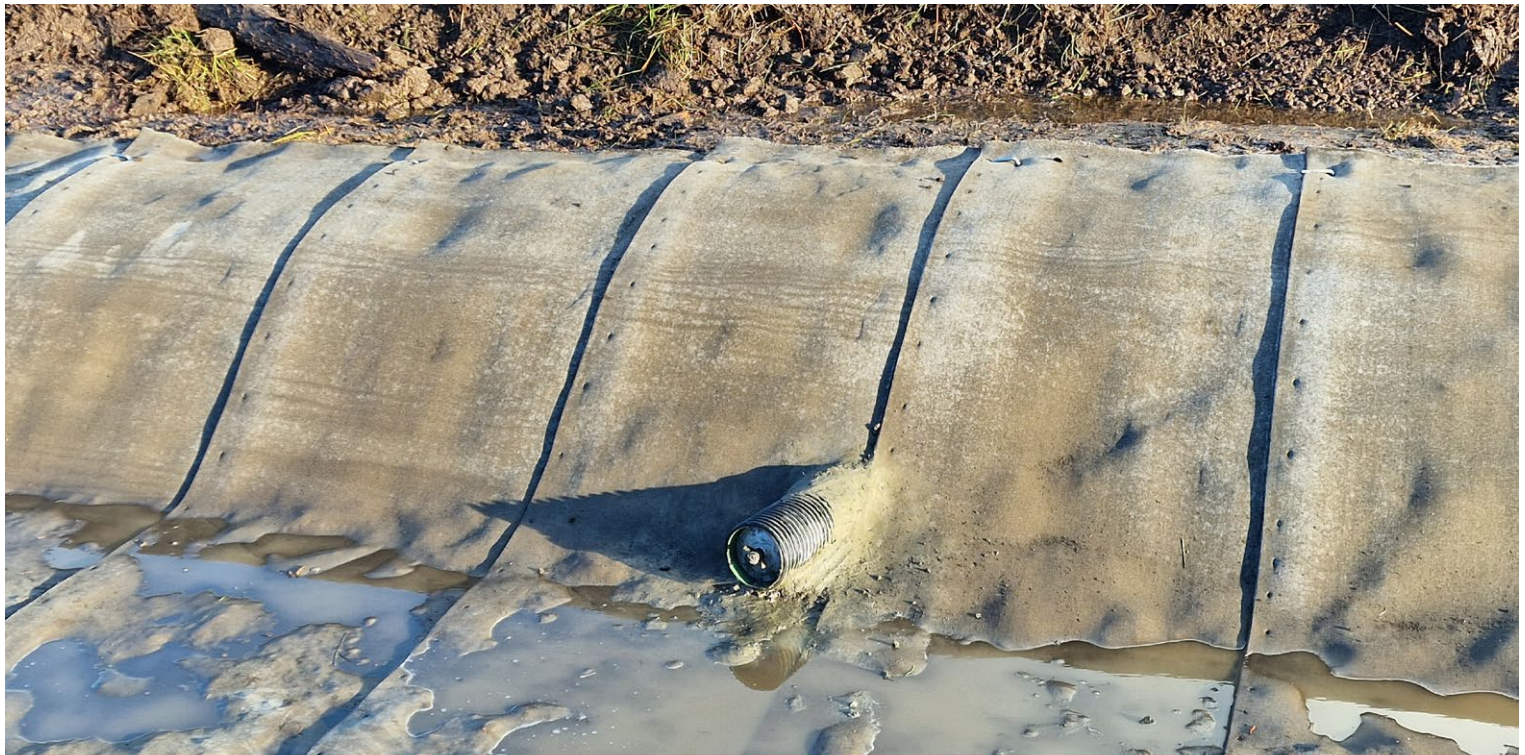
CCT3™ easily accomodated existing pipes within the channel
