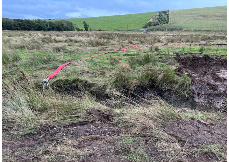
Water overpumped during the installation
