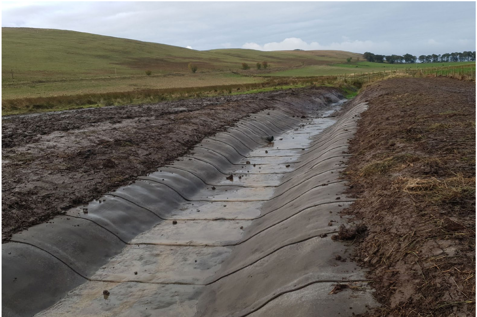
Anchor trenches backfilled
