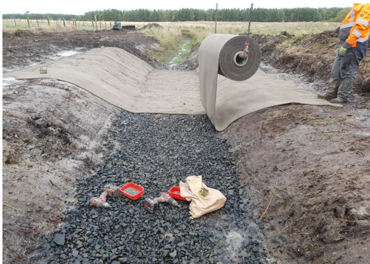
CCT3™ material laid transversely across channel
