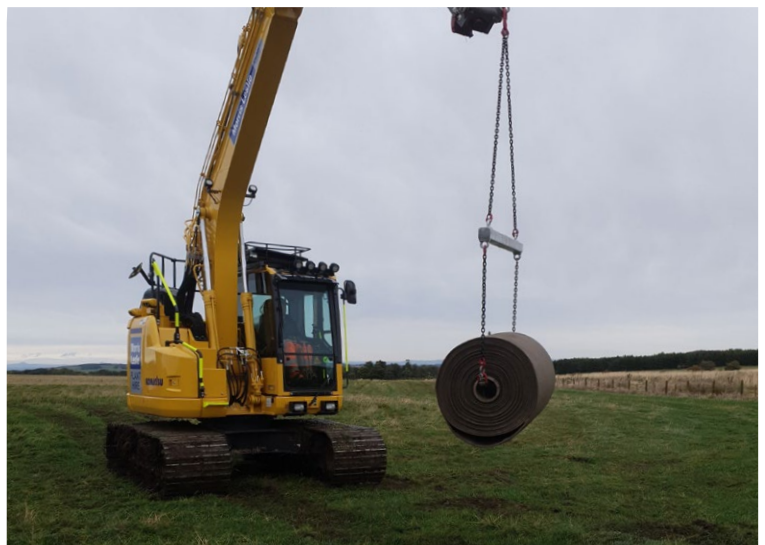
CCT3™ Bulk Rolls deployed using spreader beam
