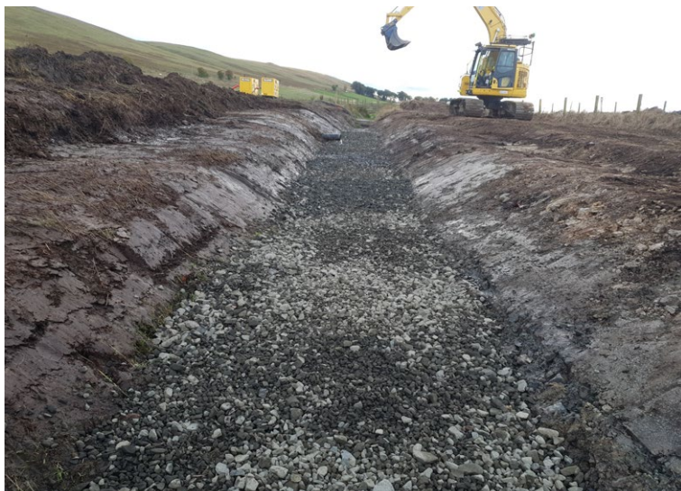
Channel excavated & rock placed in invert
