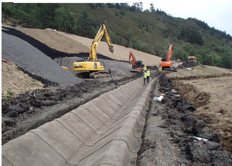
CC laid out prior to hydration
