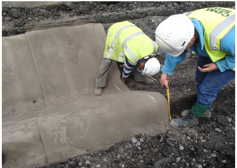
Marking the 100mm overlaps in chalk & measuring 250mm anchor trench
