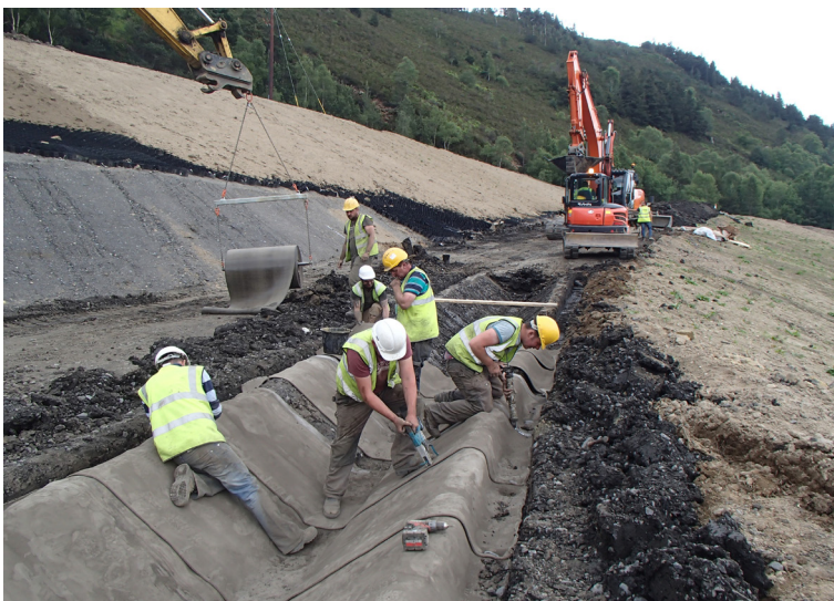
Sealing overlaps with Clearfix sealant & securing with screws at 200mm intervals
