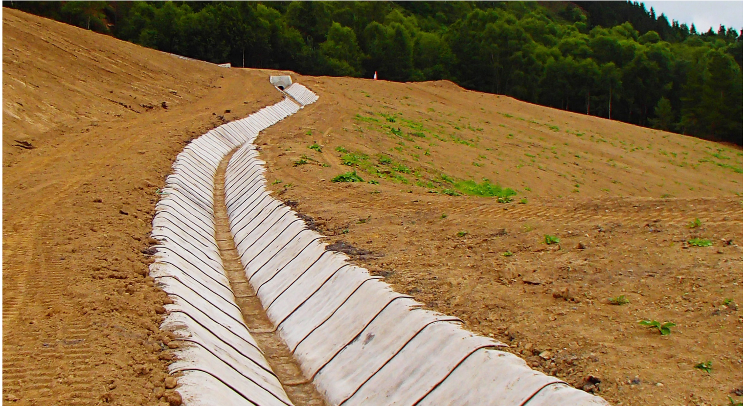
Lined channel immediately after installation
