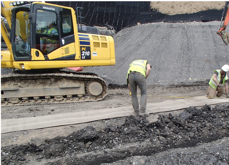
Measuring the CC prior to cutting to match channel width
