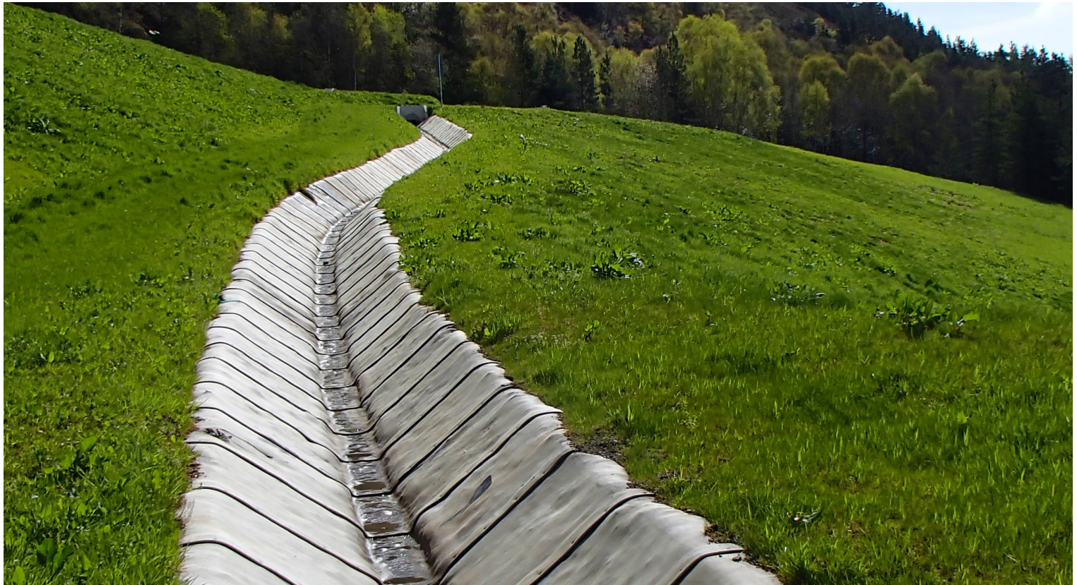
Lined channel, 1 year after installation
