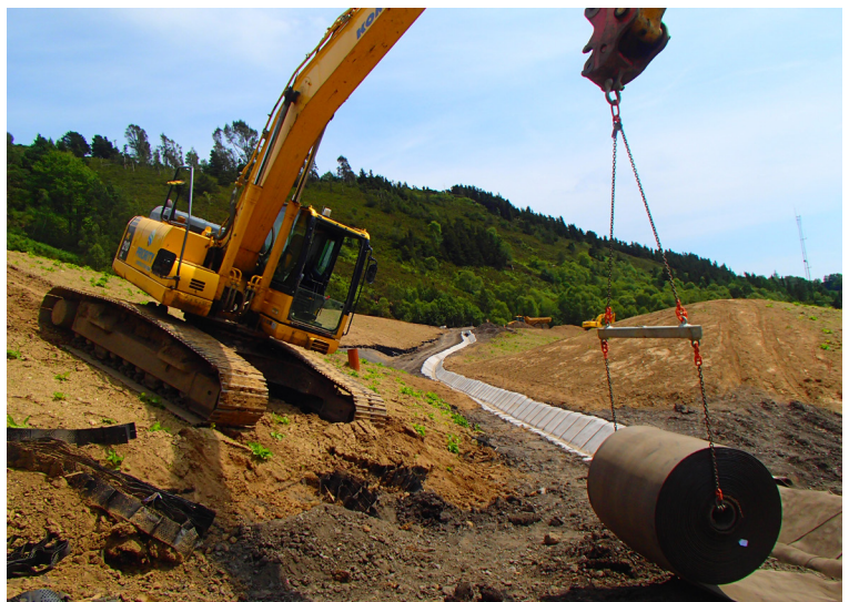
CC13™ was delivered in Bulk Rolls and deployed from a spreader beam
