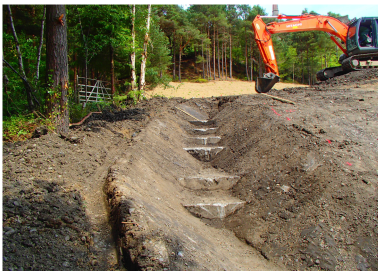
Spillway steps produced, prior to installation
