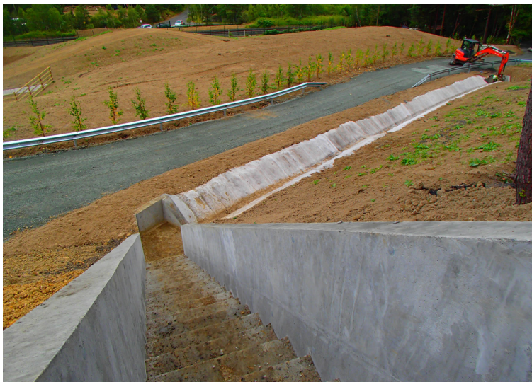
Poured concrete spillway leading into CC™ channel
