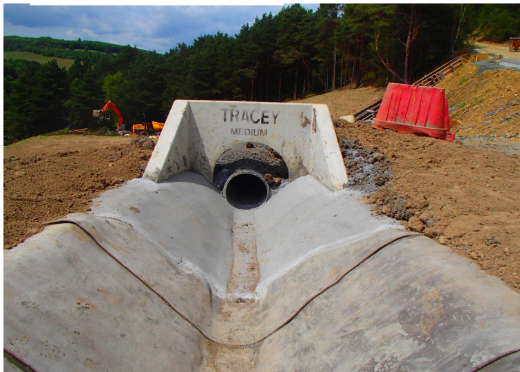
Headwall detail on upstream side
