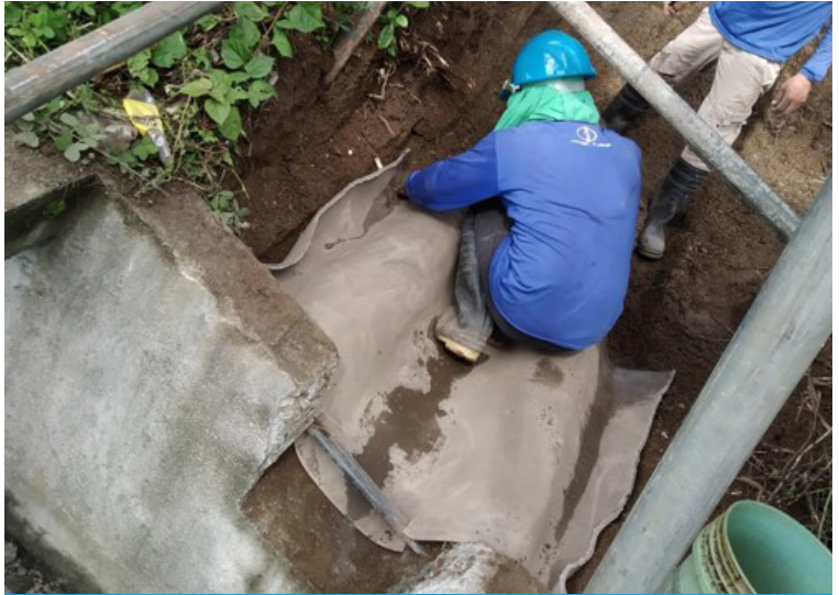
Installing CC at the outfall at toe of slope
