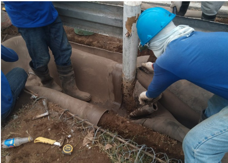
CC was easily installed around existing infrastructure
