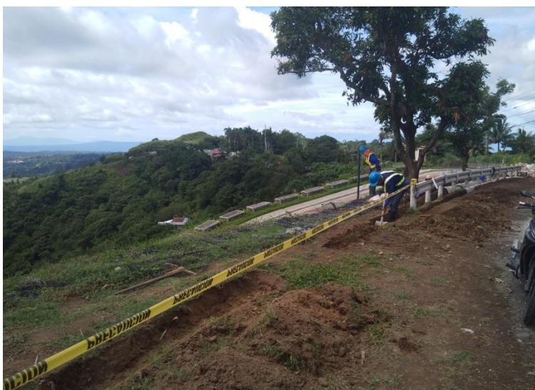
Excavating roadside drainage channel using shovels
