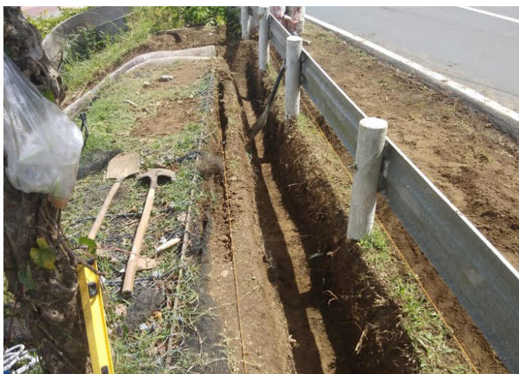
Roadside channel aims to divert surface runoff
