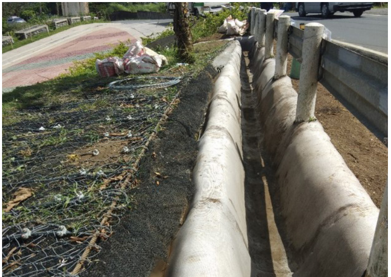
Completed section of roadside channel
