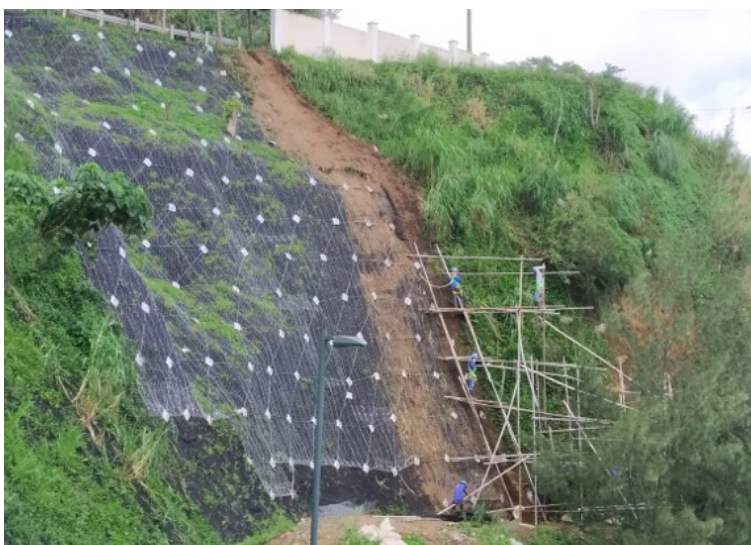
Preparing channel down slope face
