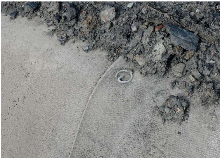
Fixing pins were used to secure material in anchor trenches
