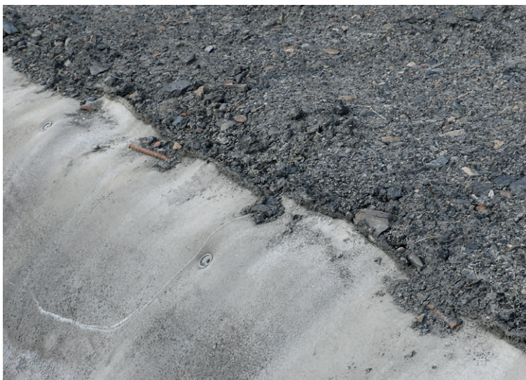
Backfilled anchor trenches
