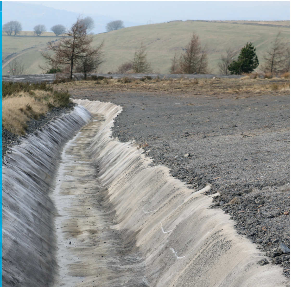
Completed CC lined drainage channel
