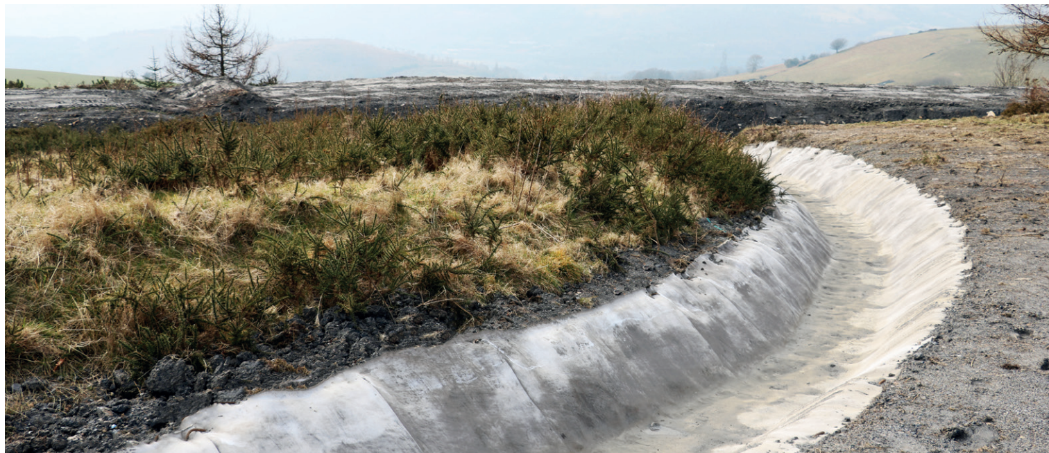
CC's flexibility allowed for easy accomodation of bends and corners
