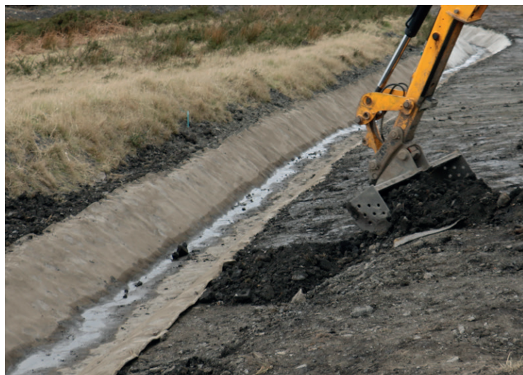
Anchor trenches were backfilled using diggers
