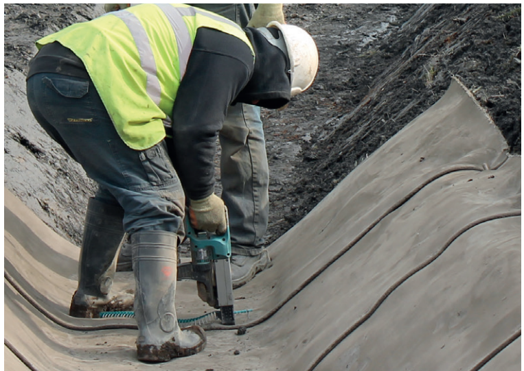
Screws were used to joint overlaps
