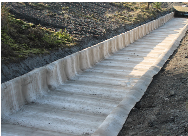
CC was laid transversely
