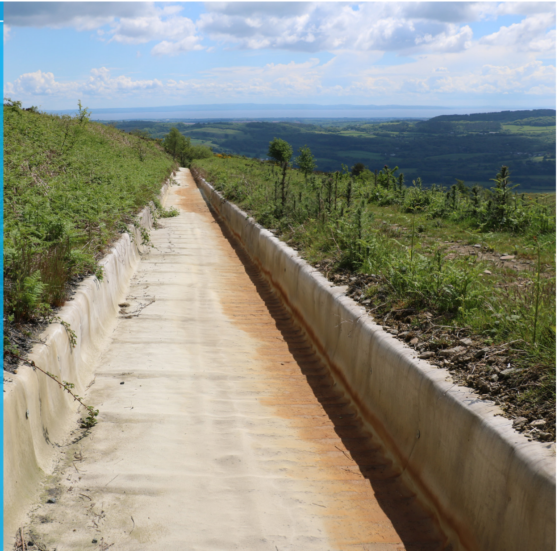
Completed section of CC lined drainage channel at Bedwas Colliery
