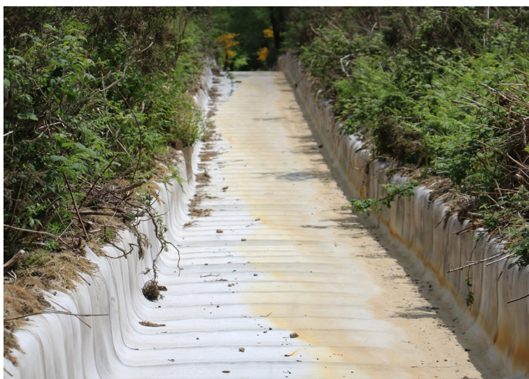
CC fixed to invert using shot-fired nails
