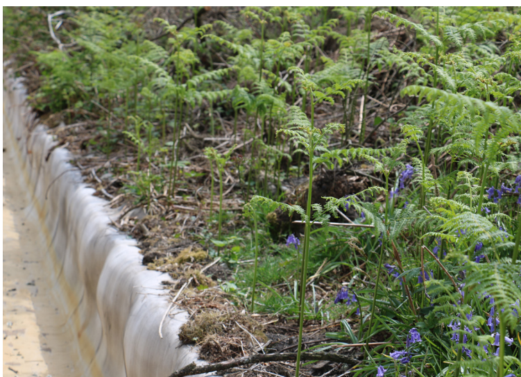
Back filled anchor trenched edge detail filled
