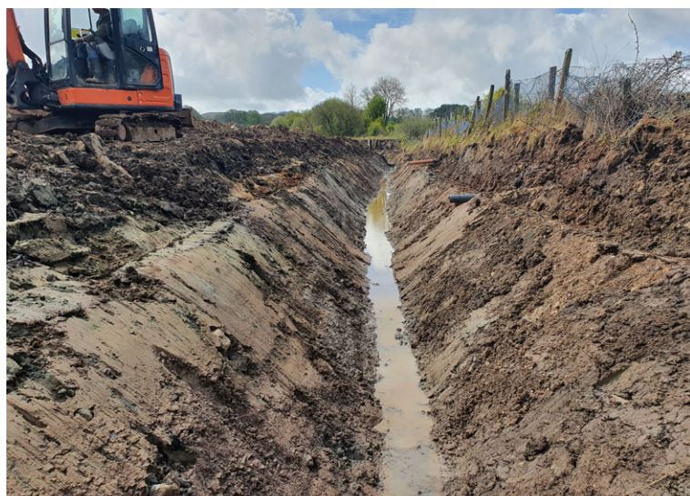
Channel excavated and inlet pipes installed
