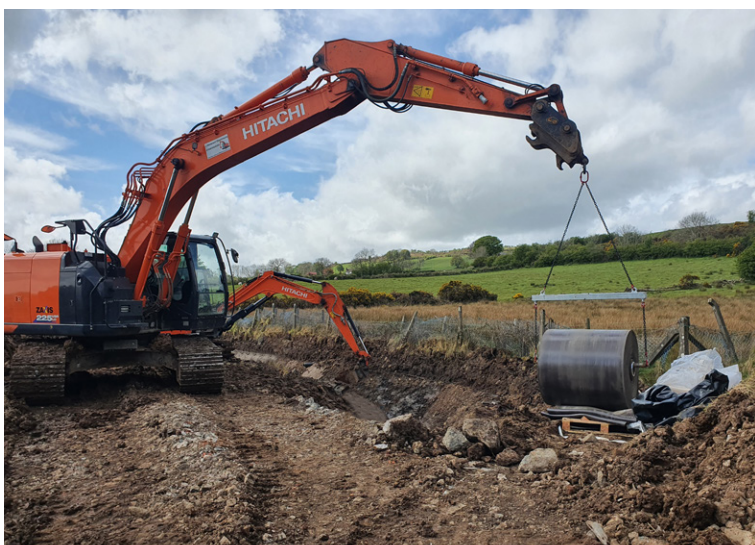
CC Bulk Roll dispensed from excavator mounted spreader beam
