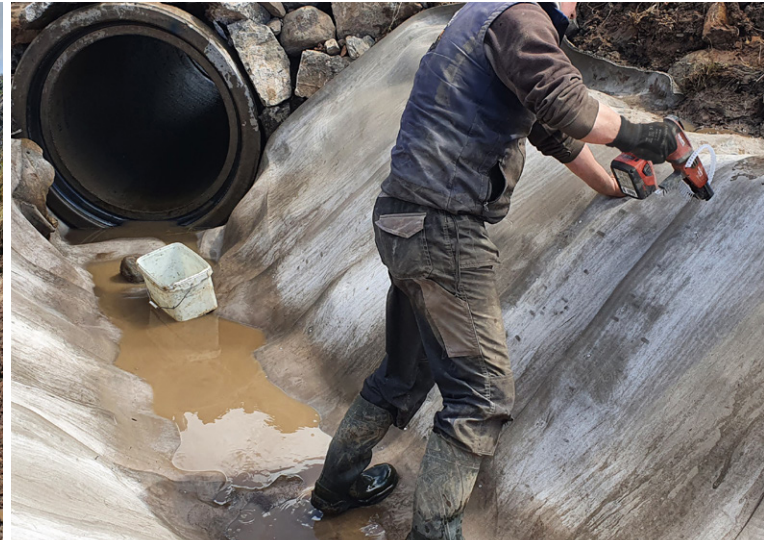
CC layers screwed using auto-fed screw gun
