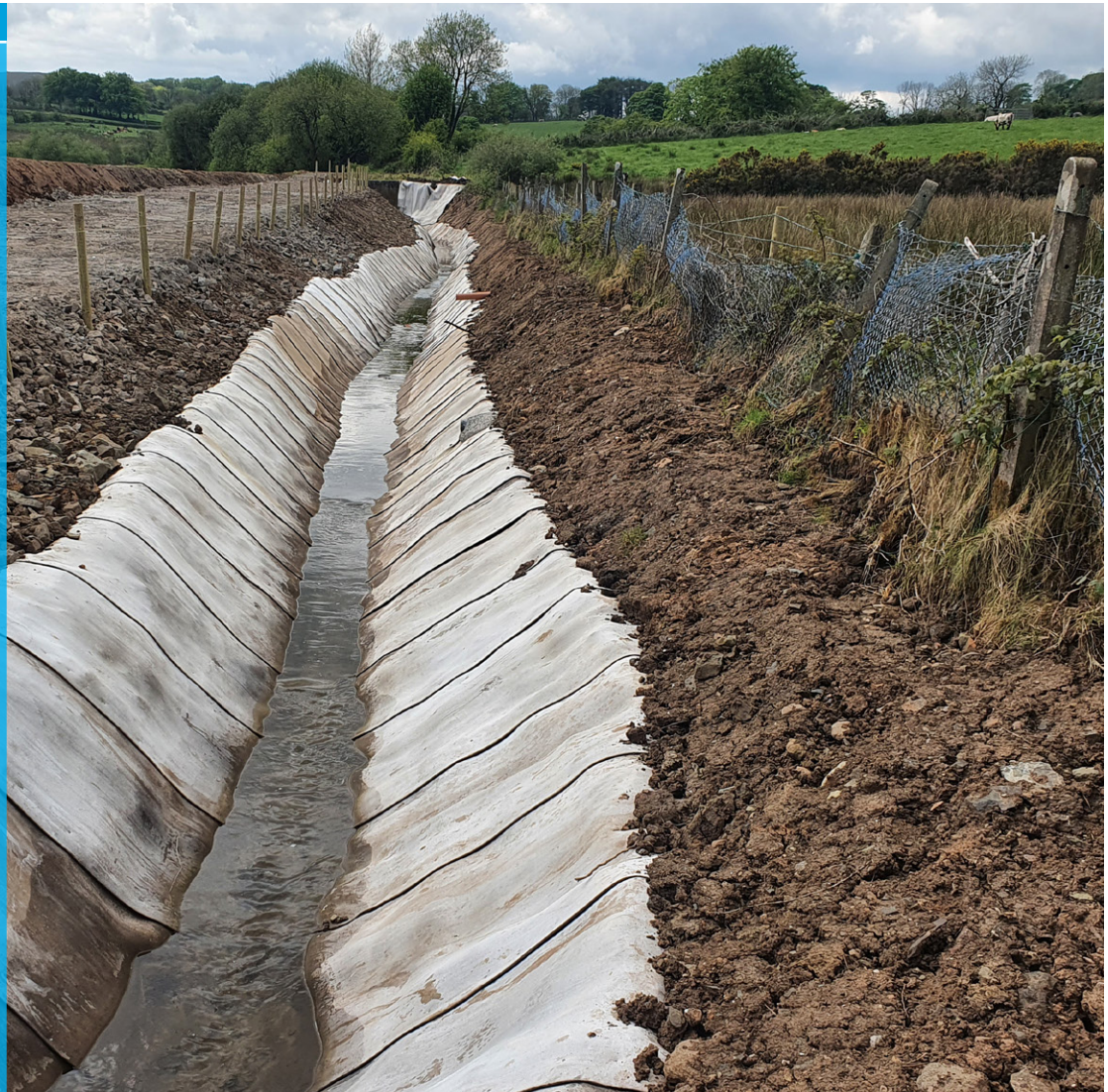
Completed CC lined channel at Boghill Dam in Northern Ireland
