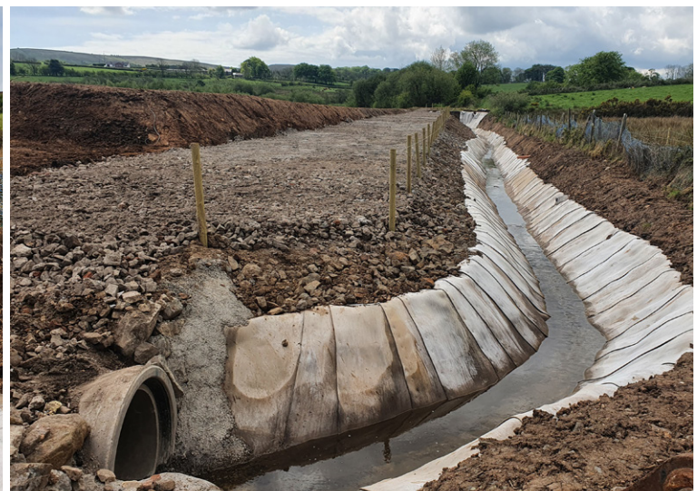
Headwall and corner detail
