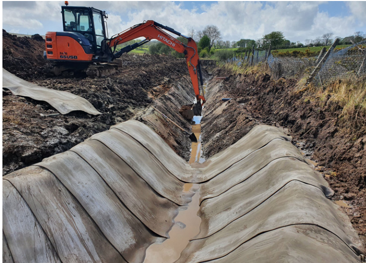
CC laid transversely across the channel
