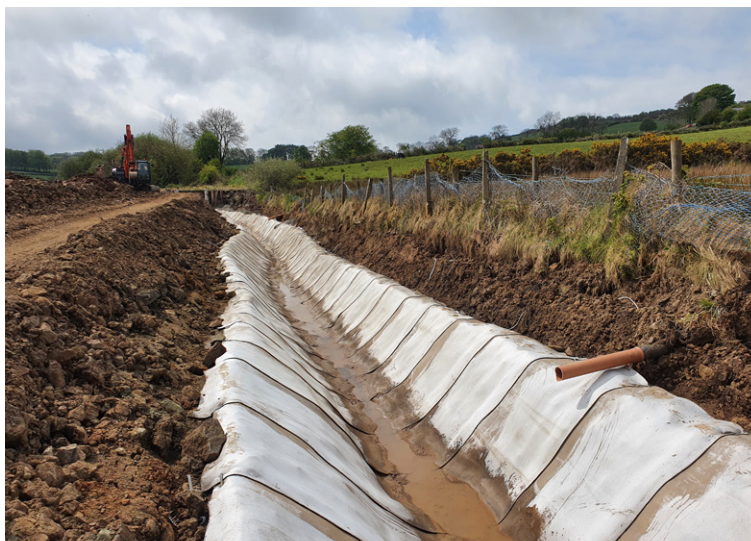
Inlet pipes installed to relieve hydrostatic pressure from the embankment
