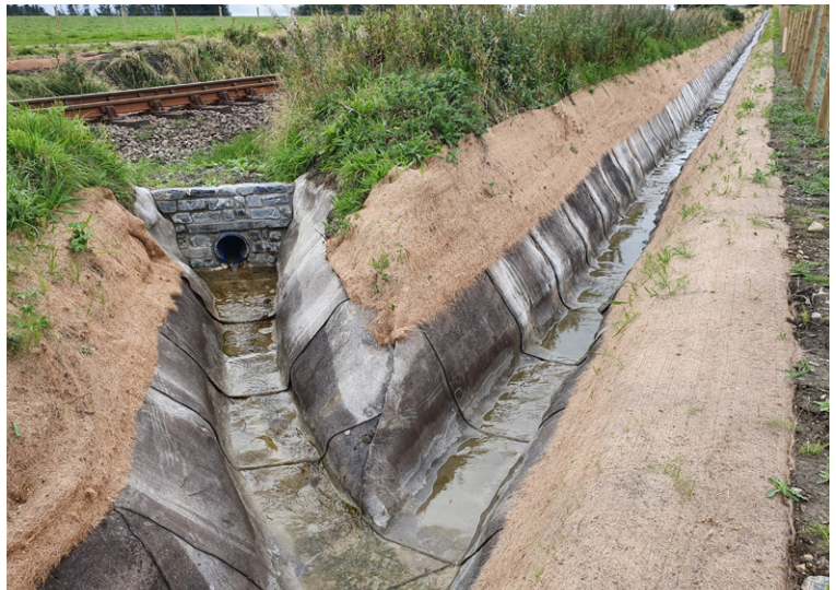
CC lined arterial drainage channel
