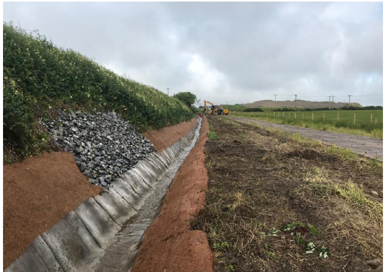
Erosion mat installed on field side
