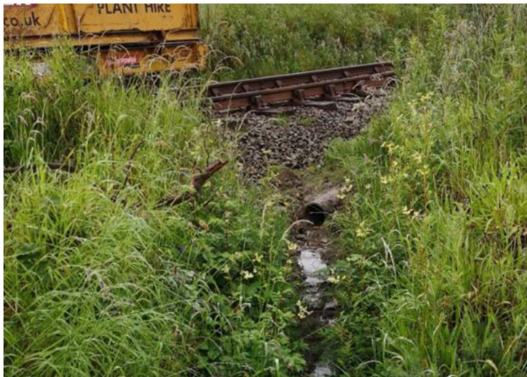
Unlined arterial drainage channel
