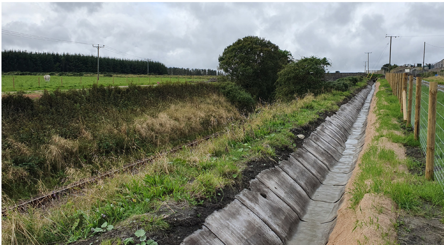
Completed CC lined crest drainage channel
