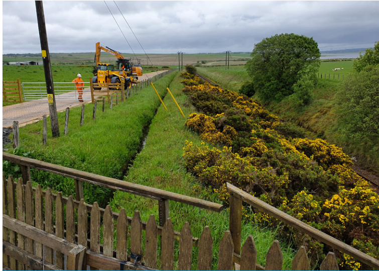
Unlined crest drainage channel
