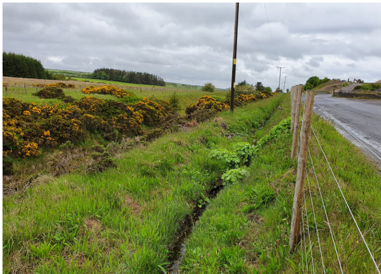
Unlined channel showing scour
