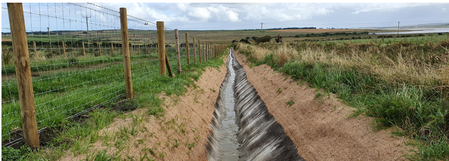
Completed CC lined channel
