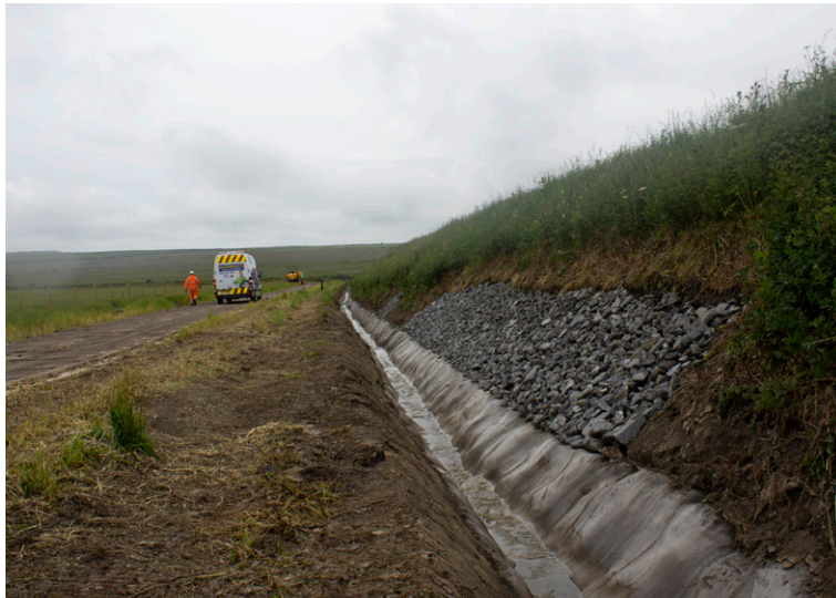
CC installed prior to erosion mat
