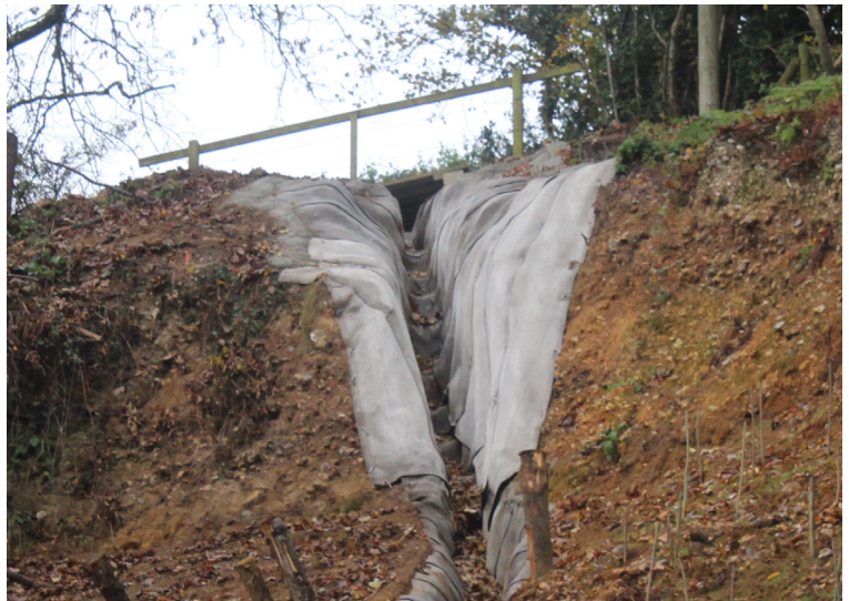
CC5™ was installed to provide slope protection at the steepest point
