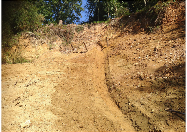
Vegetation was removed and the channel was dug by hand
