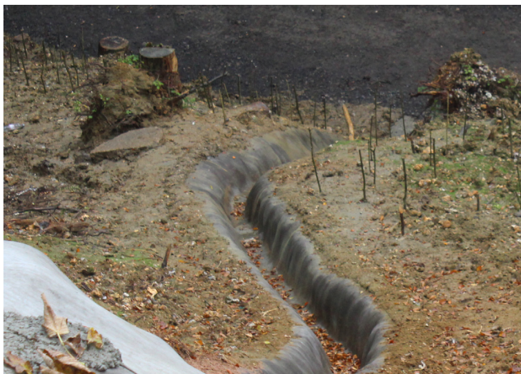
CC grouted into existing channel
