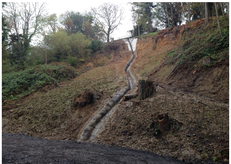
Channel connected to pipe under trackway
