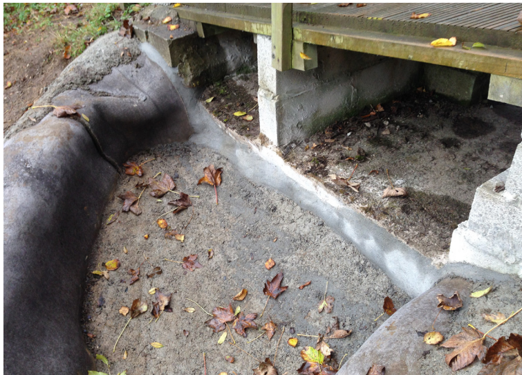
CC grouted into existing channel
