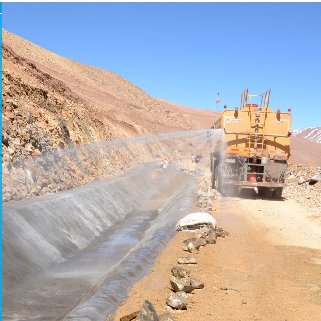
Section of CC-lined ditch undergoing hydration
