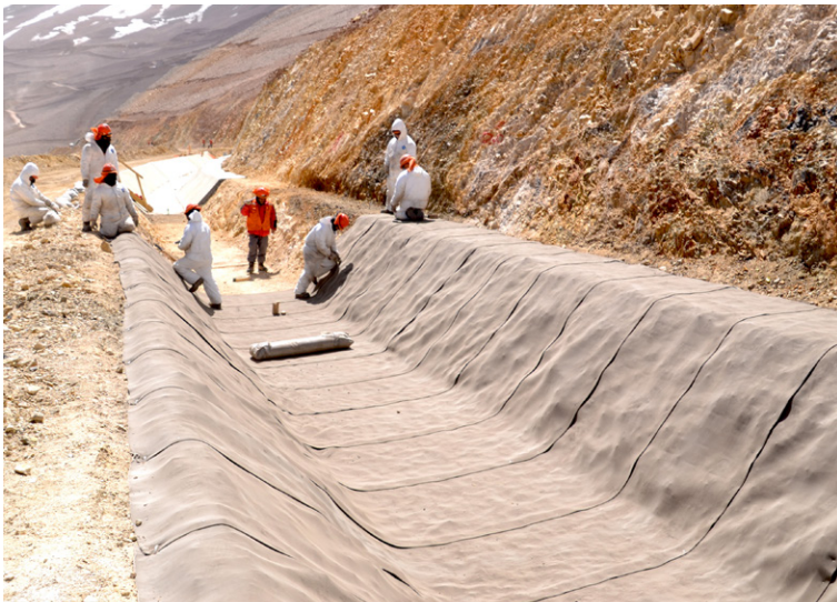
CC edges pegged and buried in anchor trenches
