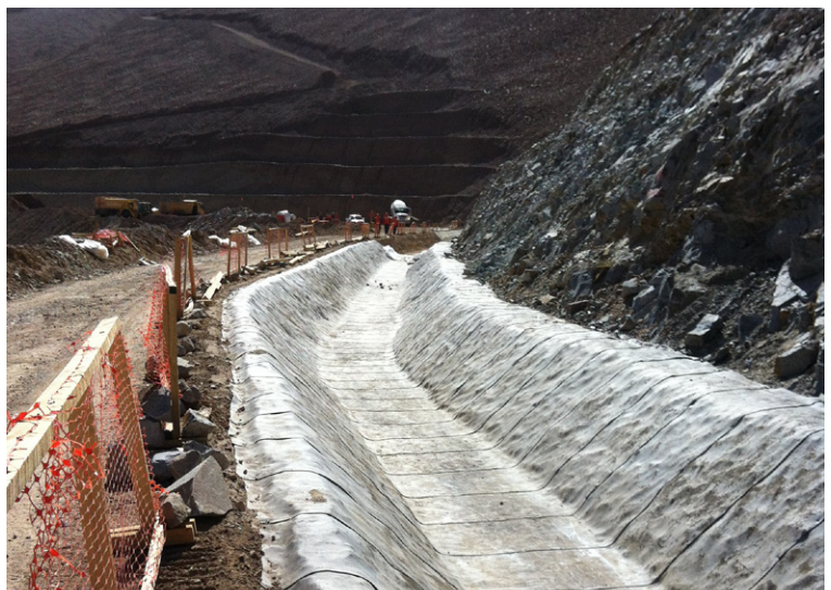
Completed CC-lined section of ditch
