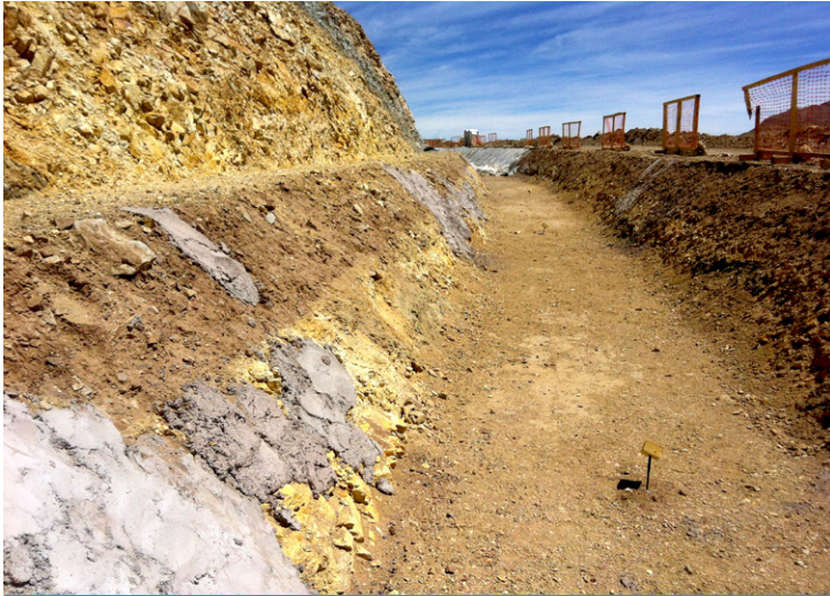
The ditch was graded and cleared of rocks and debris prior to installation
