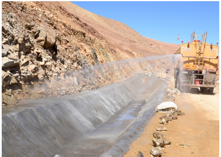
CC hydrated via water tanker
