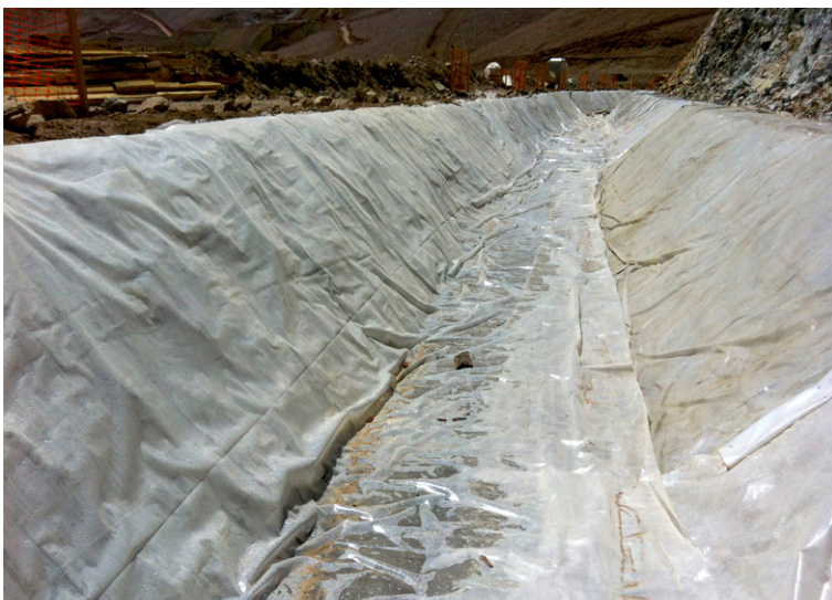
CC covered with plastic sheeting to protect it from low temperatures
