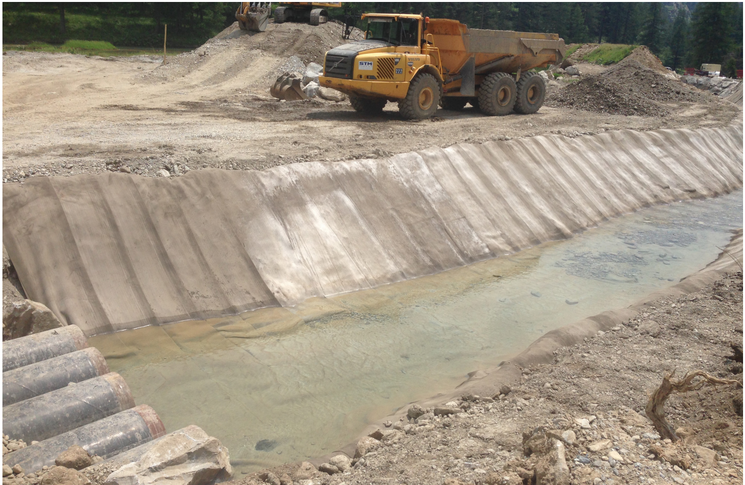
The complete diversion channel showing back-filled anchor trenches
