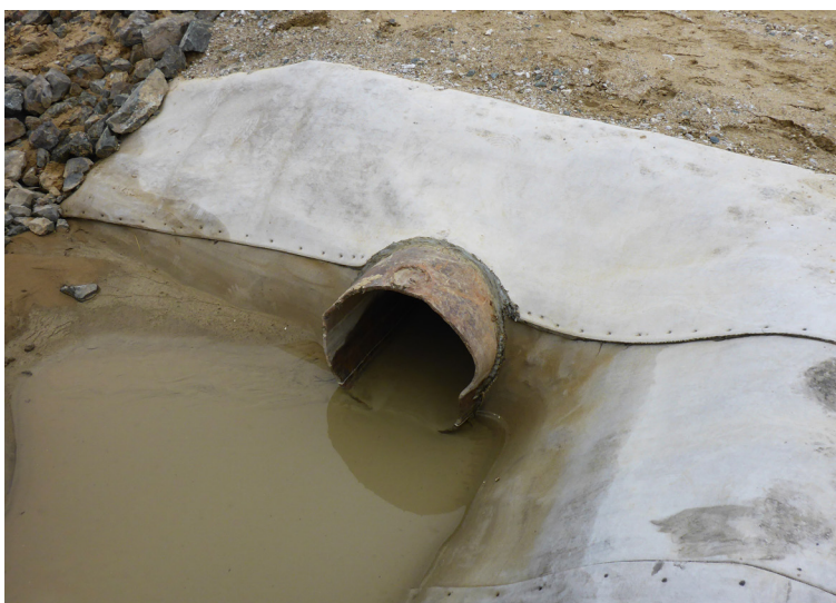
Pipe protrusion
