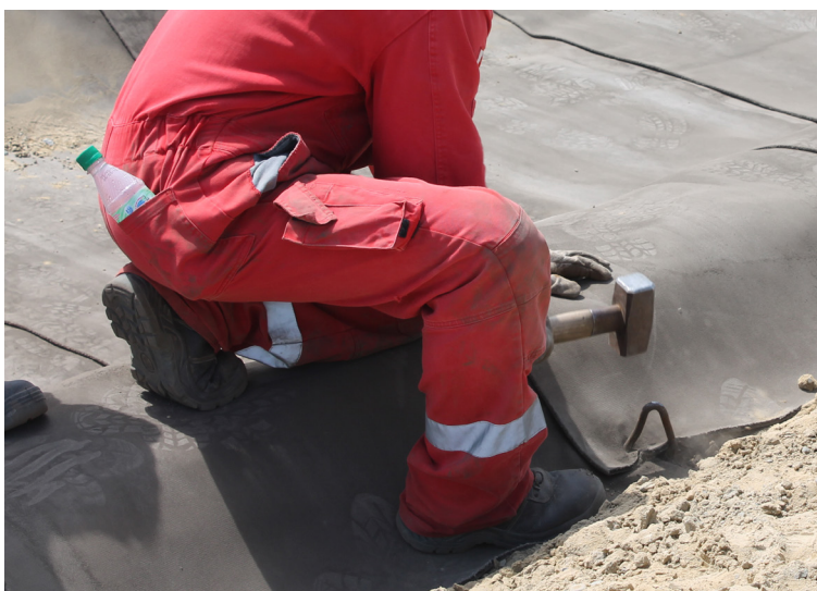
Pegging CC into anchor trench
