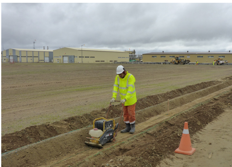
Substrate compaction
