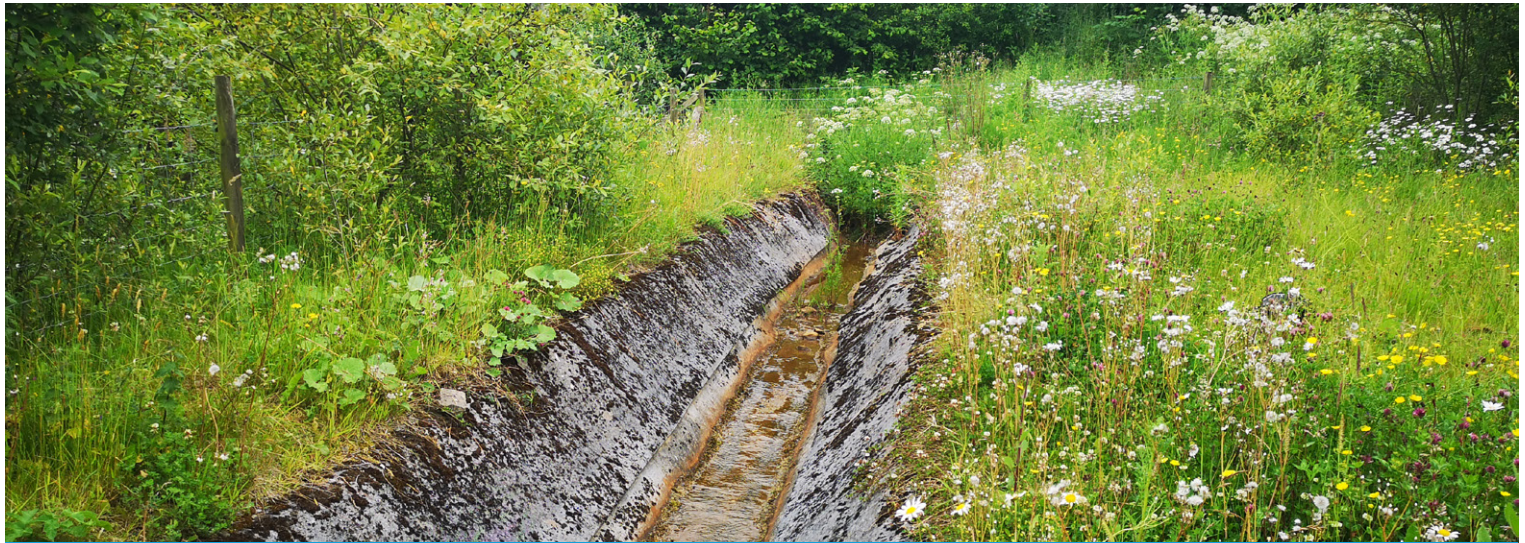
Despite significant weed and vegetation growth around the channel, the CC is performing as expected and providing weed suppression within the channel itself
