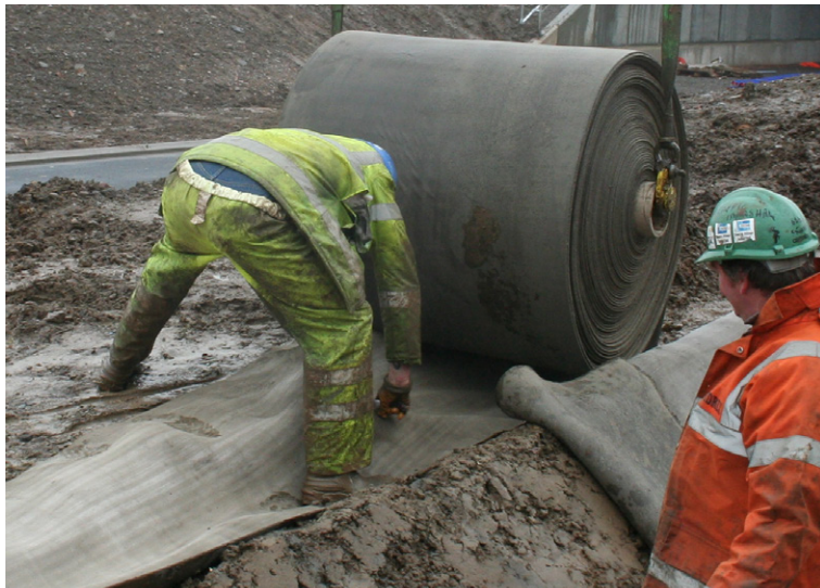
Cutting CC to required length using hand tools
