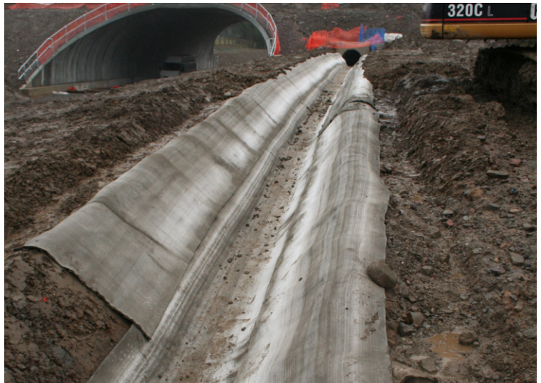
CC was laid in three longitudinal sections
