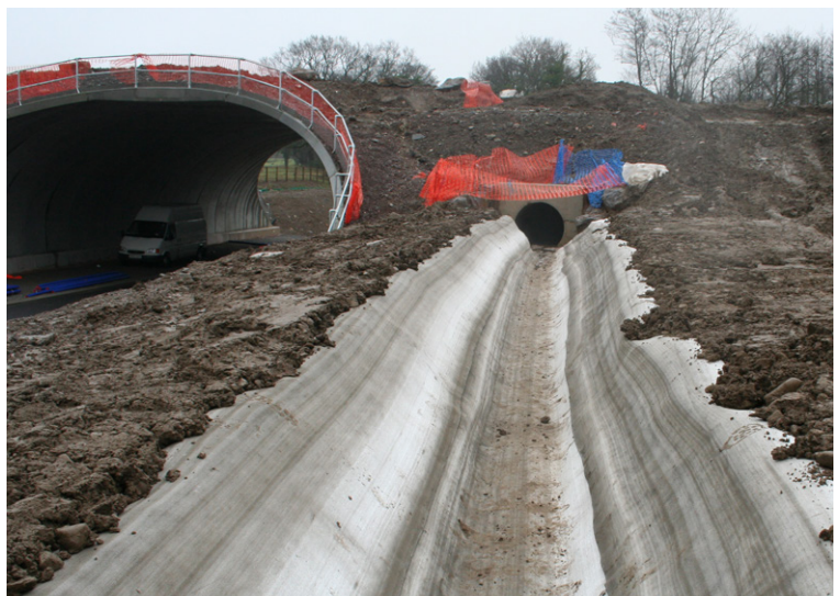
Anchor trenches were backfilled to prevent ingress
