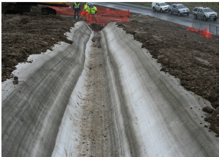
CC edges were captured in anchor trenches following installation
