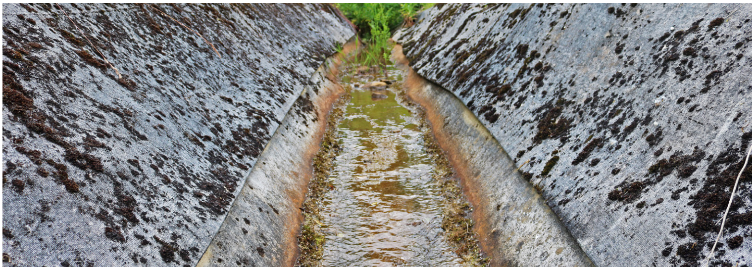
Algae and moss growth established on the fibrous top surface of the CC material
