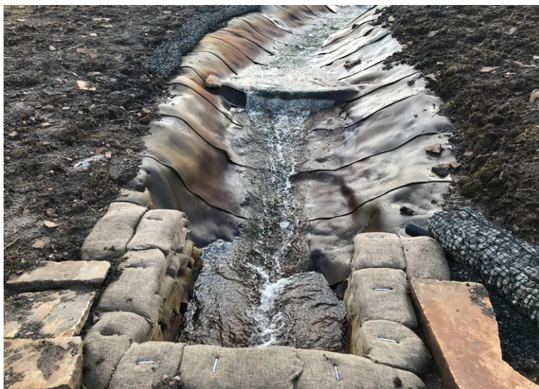
Channel terminating into downstream sandbag headwall
