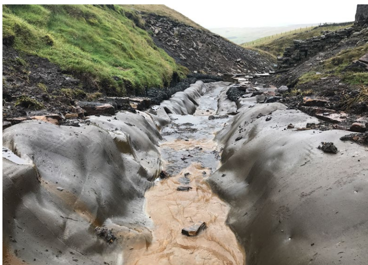
Upstream view of channel - CC able to conform to varying channel profile
