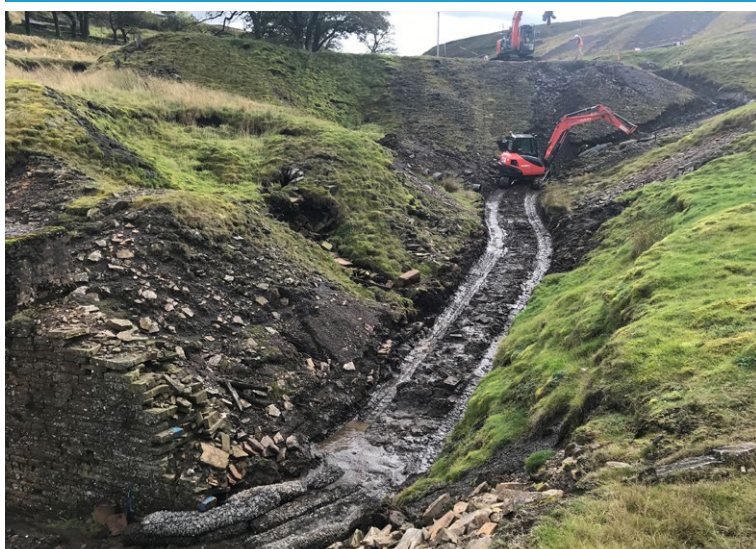
Small excavator used to create the channel profile
