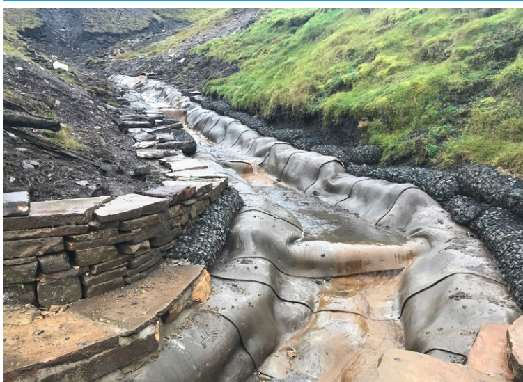
Installation began downstream, working up the channel
