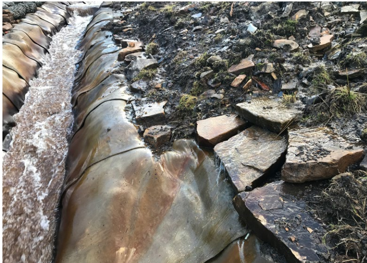
Where anchor trenches were not possible, rock rolls and stones were used
