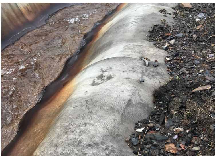
Anchor trenches used to capture CC edges where possible
