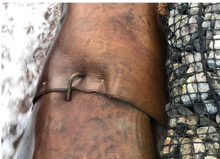
Ground pegs secured CC to substrate and screws used to joint overlaps
