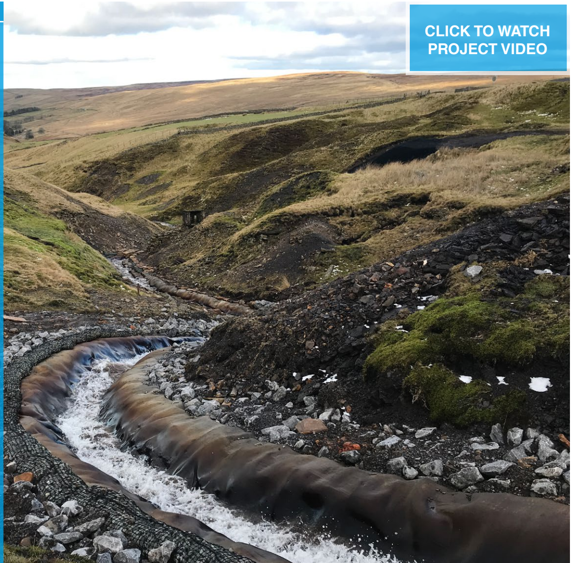
Upstream view of the completed CC lined channel
