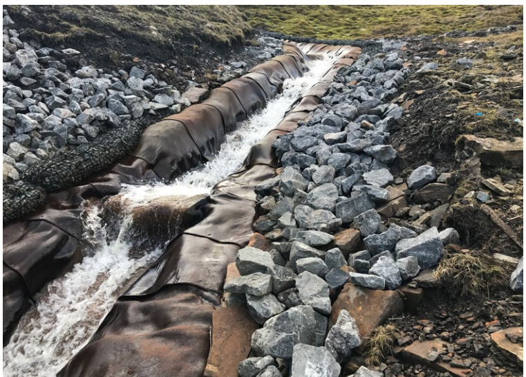
CC provides erosion control, particularly in high flow events
