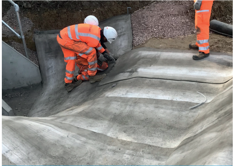
CC installed at headwall termination section
