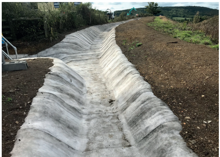
Completed junction section of CC installation
