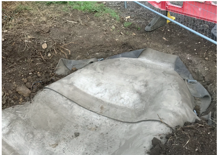
CC termination at end of channel prior to backfilling
