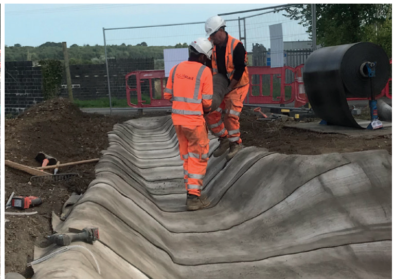
CC laid transversely and fixed in anchor trenches using ground pegs
