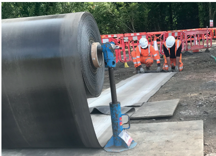
Batched material rolled and moved by hand
