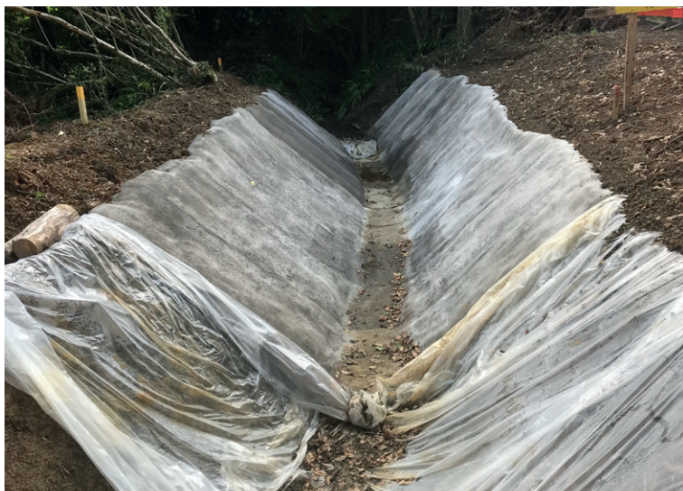
Edge of CC material covered with plastic sheeting overnight
