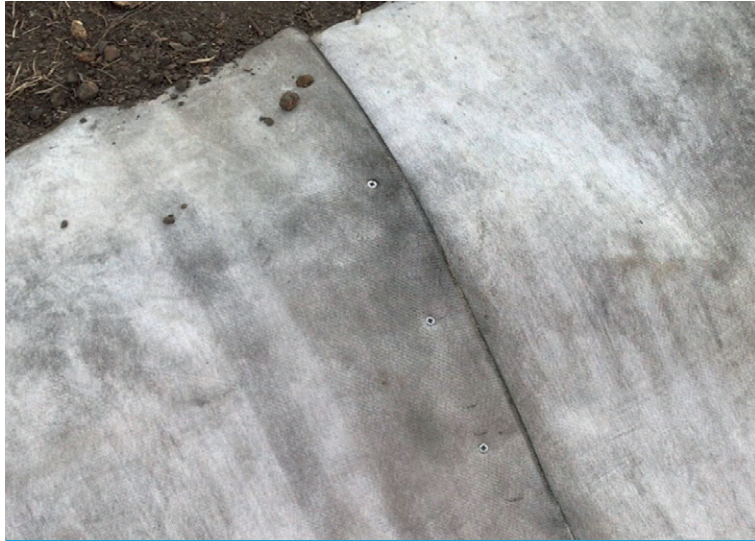
CC overlaps jointed with screws and sealant
