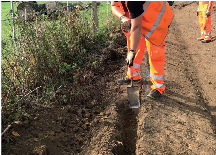
Anchor trenches dug by hand
