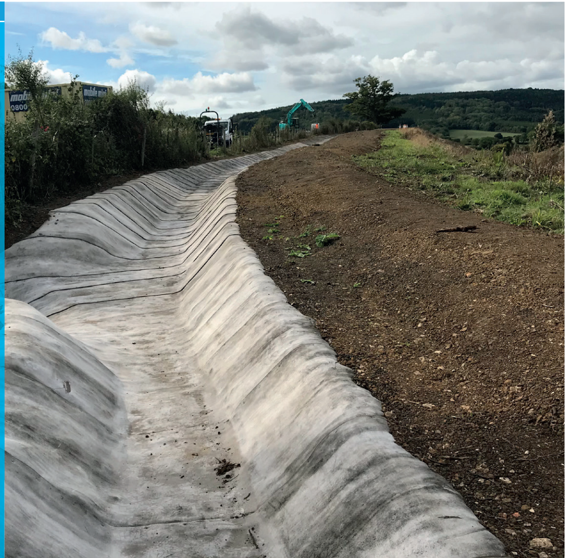
Completed CC lined drainage channel in Yeovil, UK
