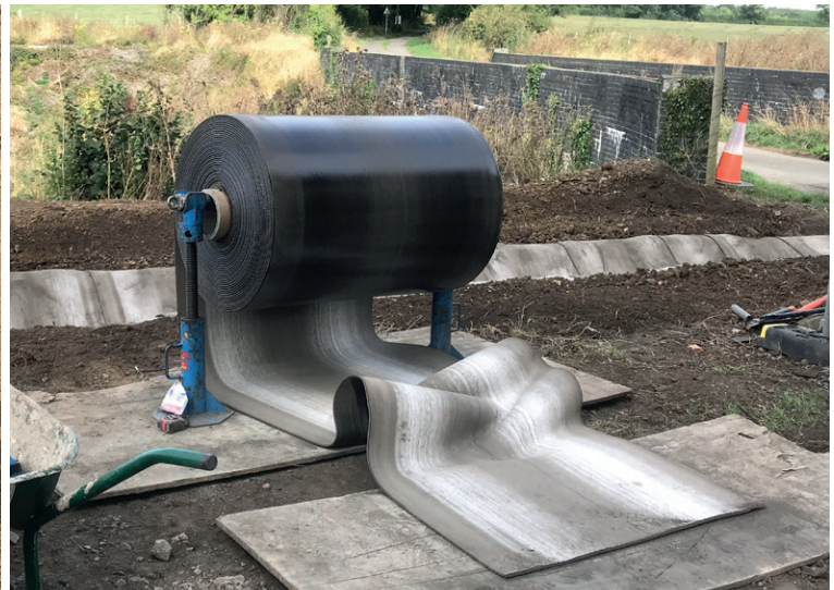
CC material cut to required length by batching on site
