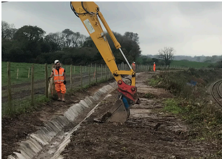
Backfilling the anchor trenches
