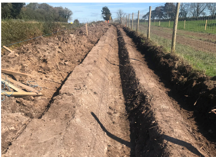
Channel following excavation
