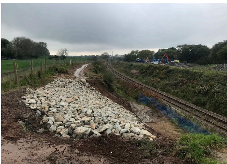
Rocks placed at channel end to protect slope
