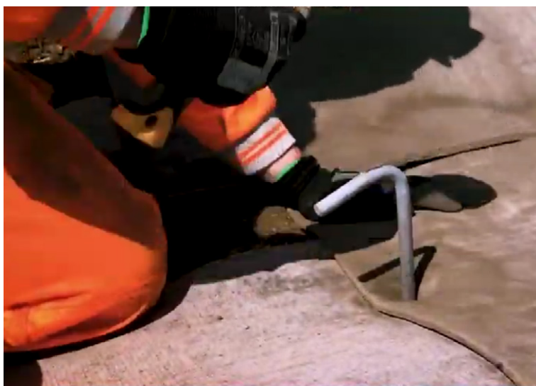
CC edges fixed within anchor trenches using ground pegs
