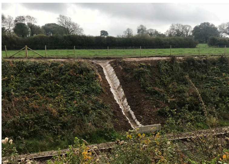
Completed outfall channel section leading to headwall
