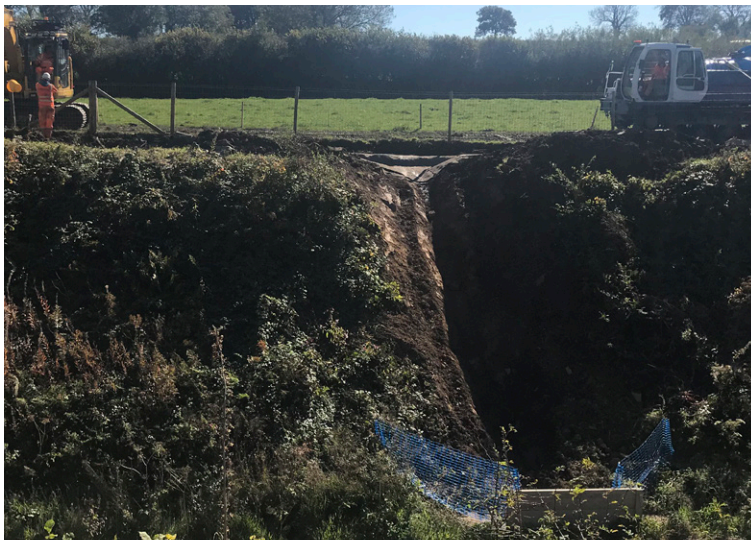
Outfall channel leading to headwall following excavation
