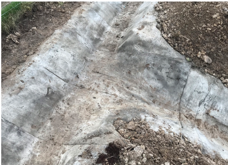
Corner detailing from main channel to outfall
