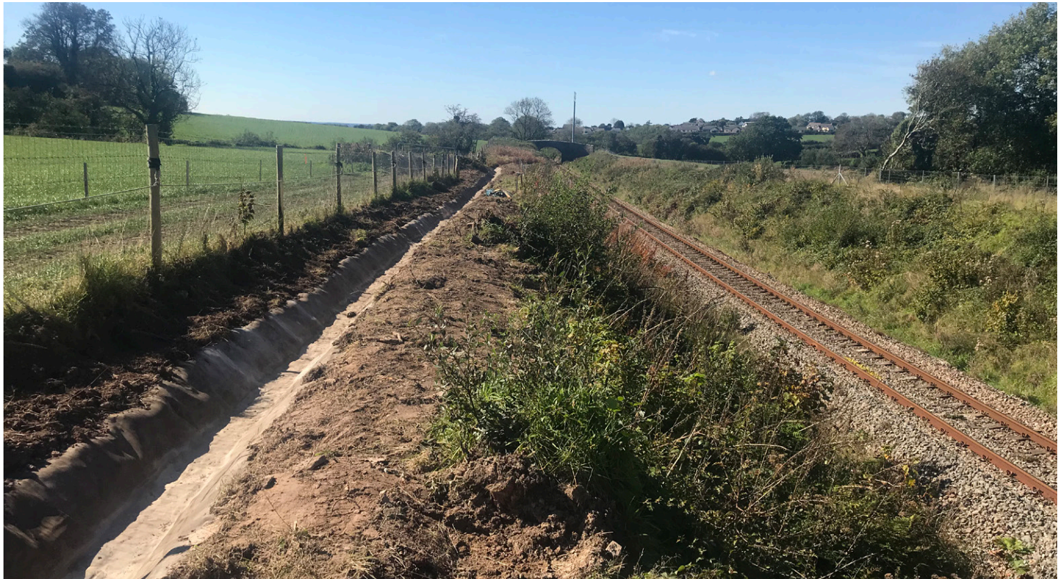
Completed crest drainage channel running adjacent to rail line
