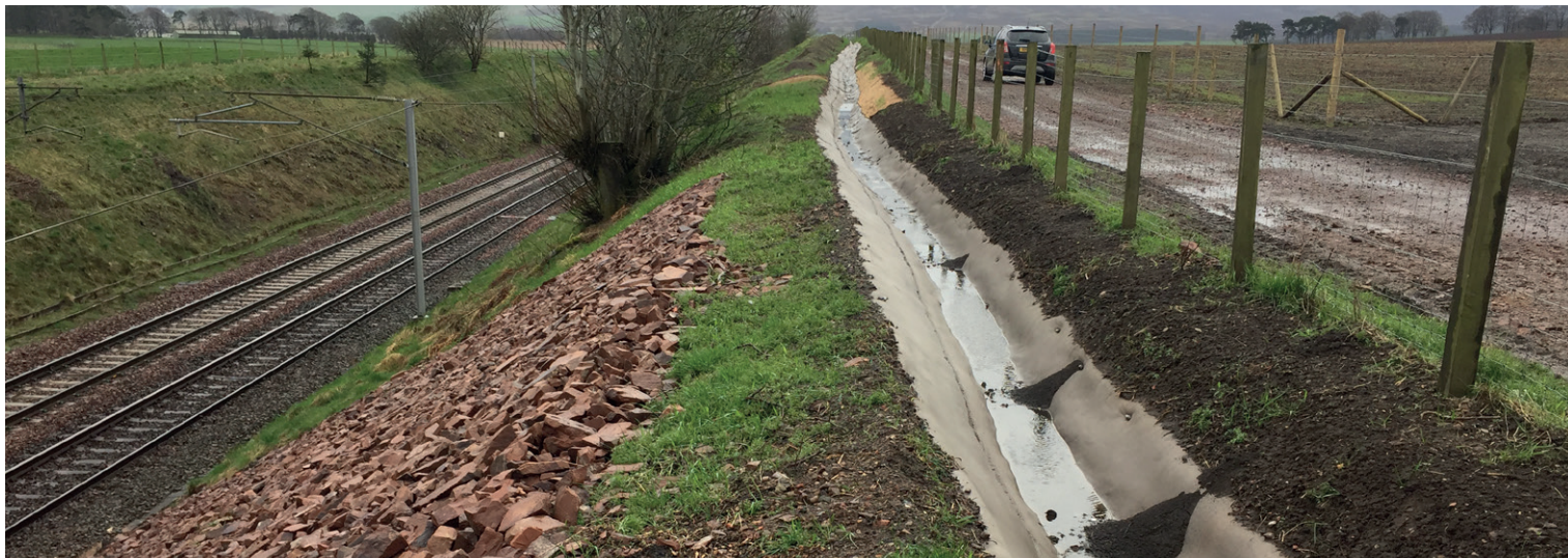
CC channel protecting rail cutting from saturation following previous landslip
