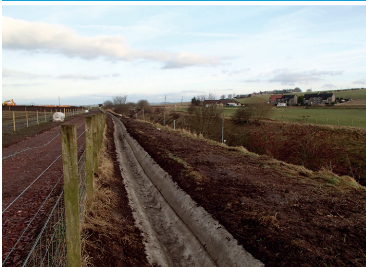
Two CC layers laid longitudinally and pinned into anchor trenches
