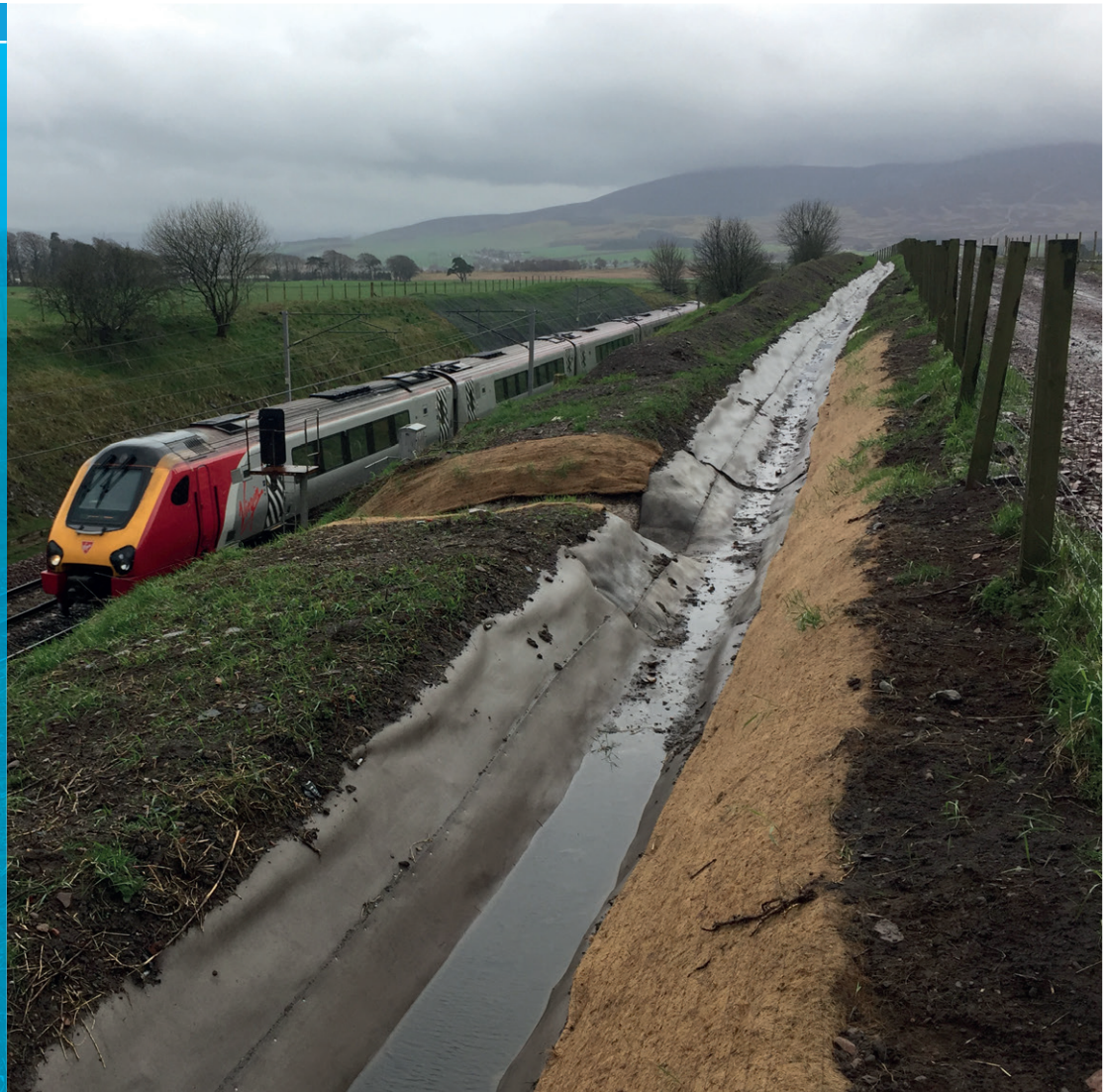
Completed channel lining installation in Scotland
