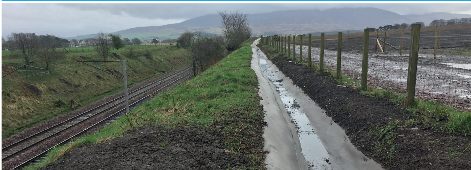
Completed CC lined channel
