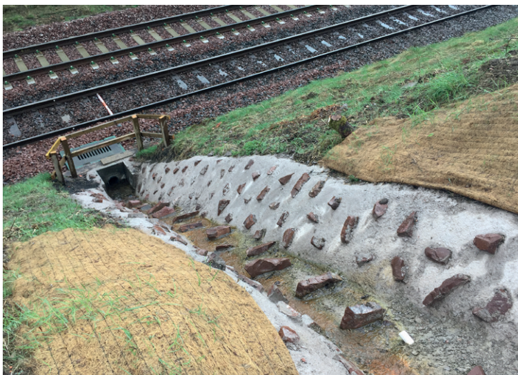
Concrete outfall diverting water into culvert underneath railway line
