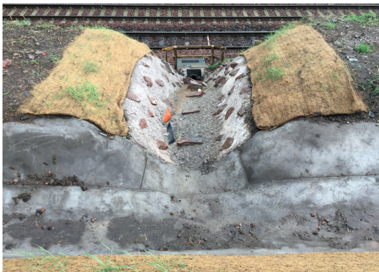
CC termination at concrete outfall
