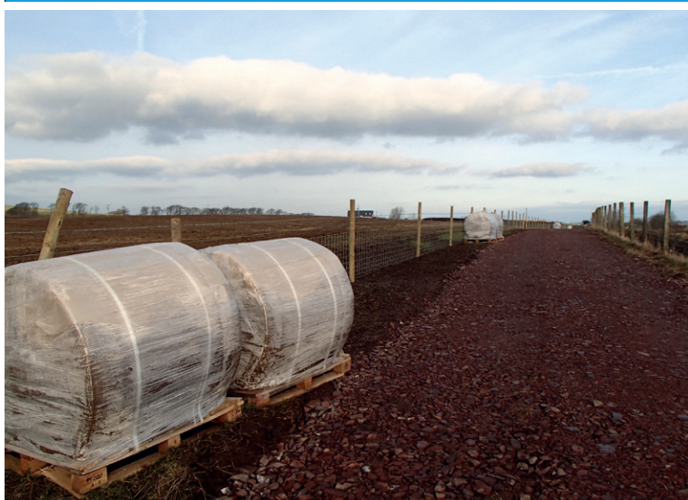
CC8™ bulk rolls placed strategically at intervals along channel
