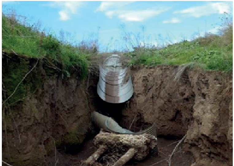
Heavy rainfall had resulted in severe undercutting
