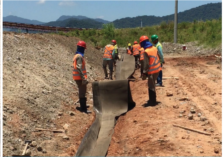
The CC being walked into place from the mounted Bulk Roll
