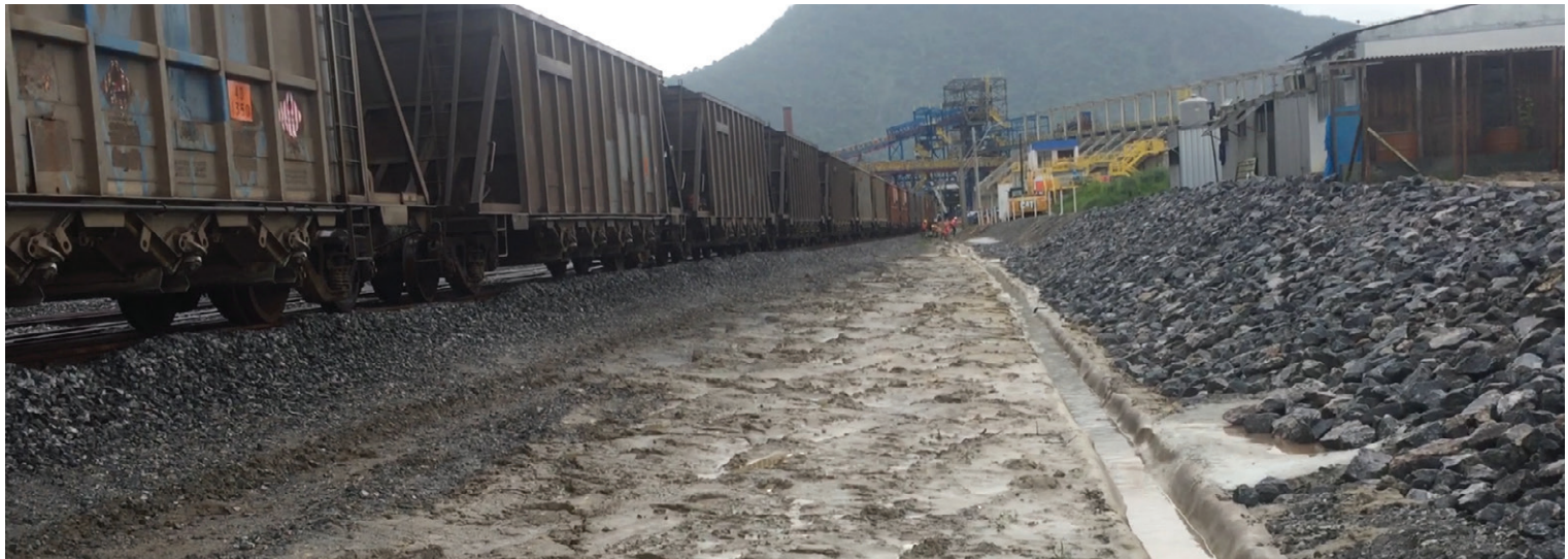
The completed channel
