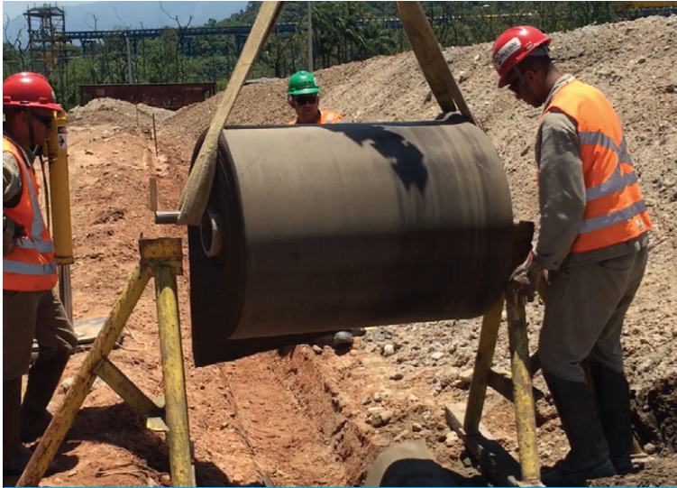
The CC being mounted onto a static spreader beam
