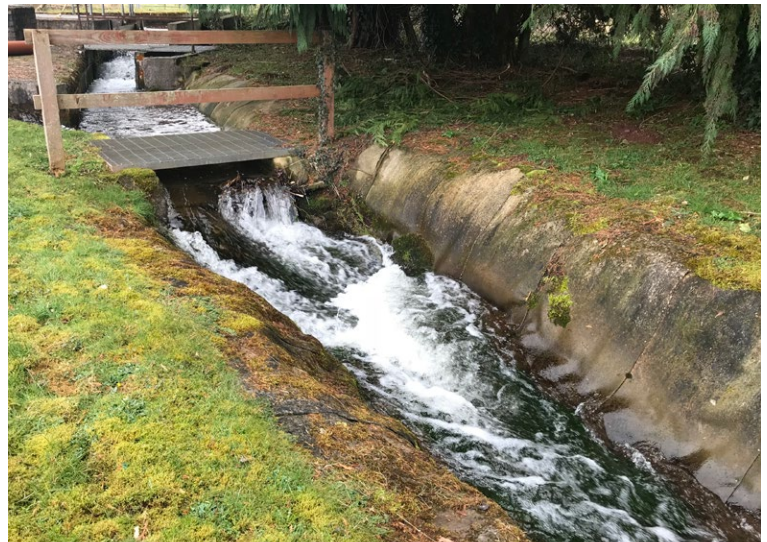
CC is providing durable erosion control, successfully coping with varying flows
