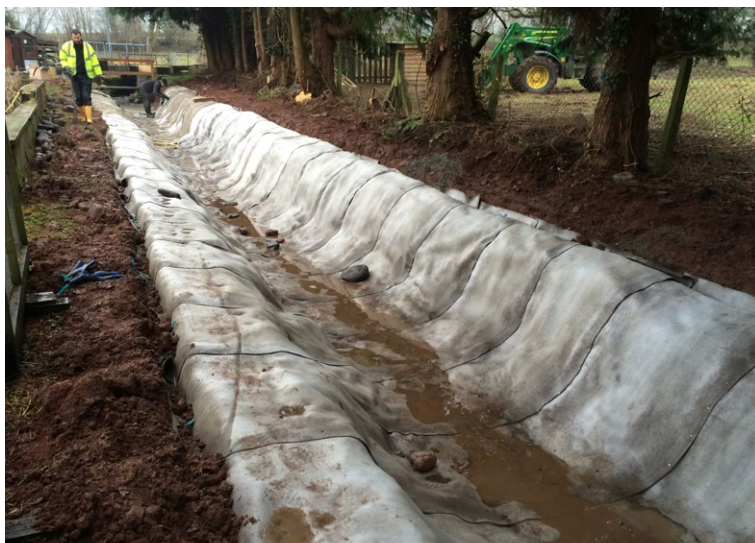
CC5™ was captured within anchor trenches and hydrated
