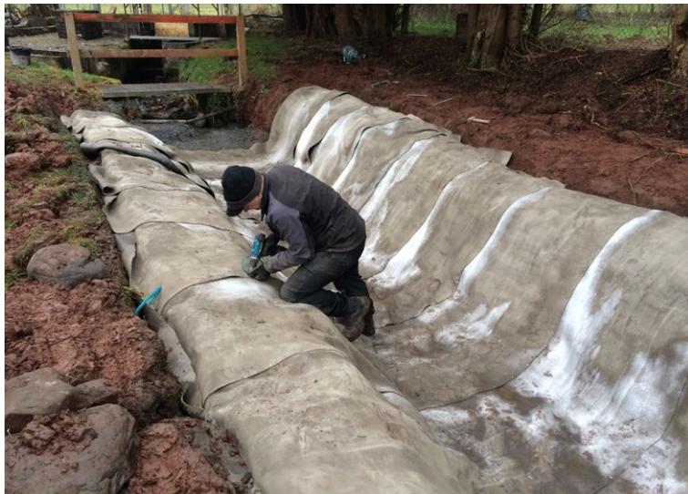
CC5™ was applied in transverse layers with a 100mm overlaps
