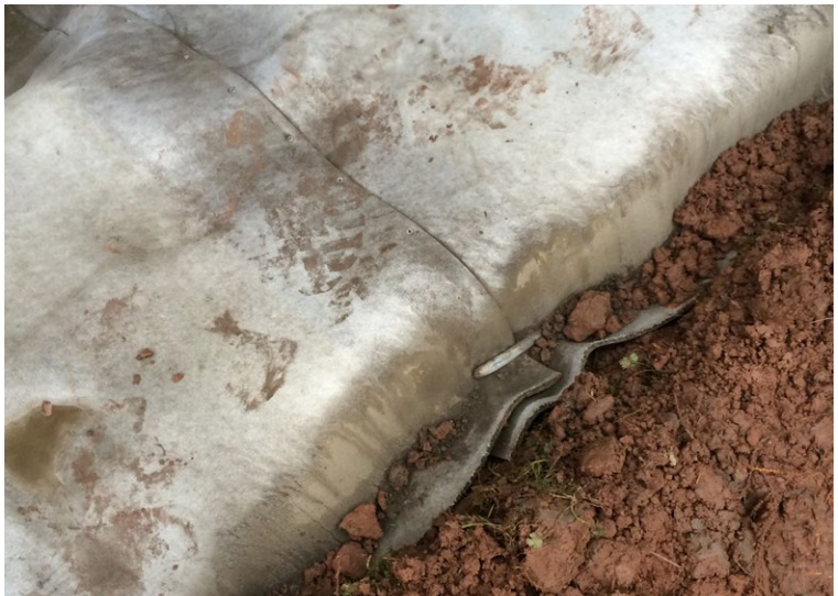
CC was fixed using steel ground pegs and concrete masonry fixings
