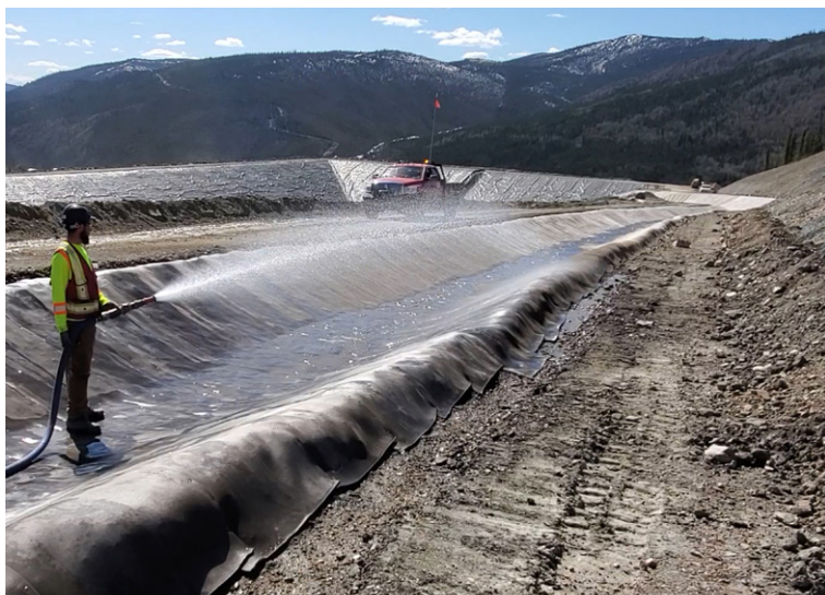
Hydration of the lined channel
