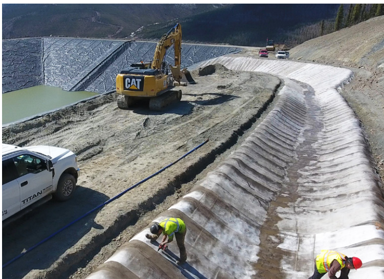
Joints were sealed and screwed for increased impermeability
