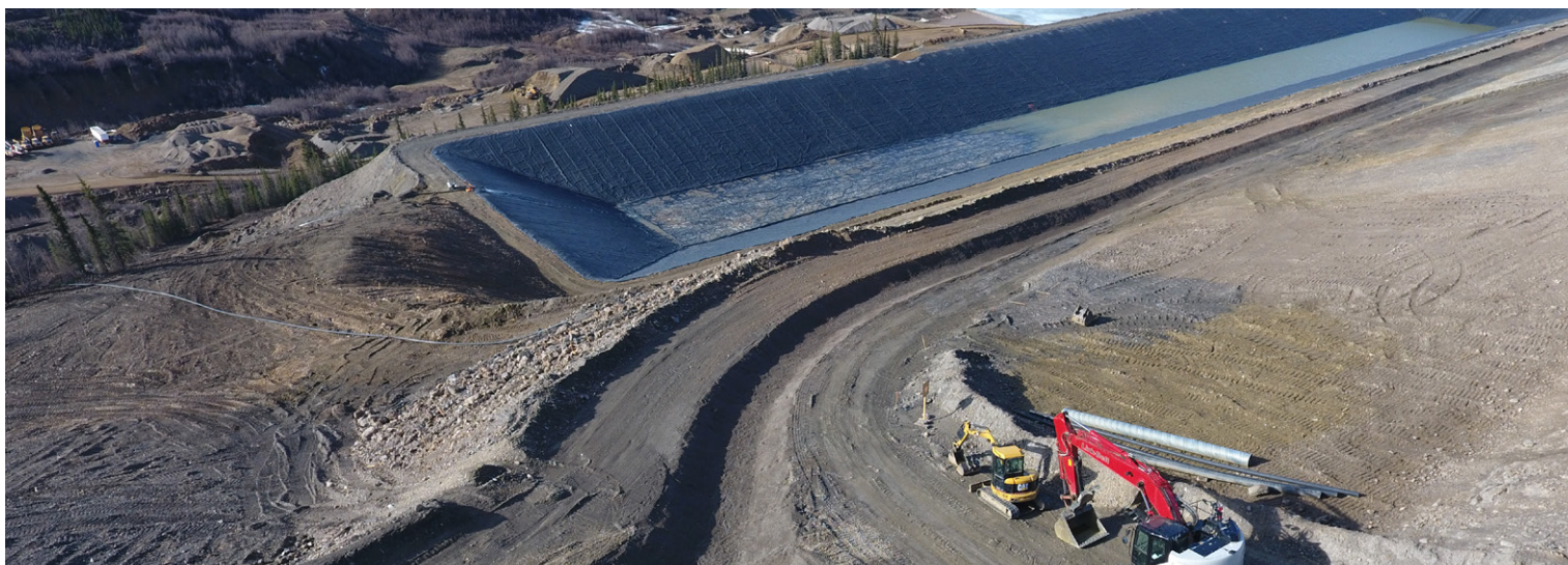
Main spillway channel to be lined with CC
