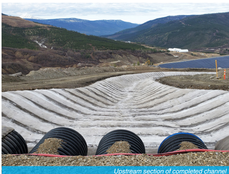
Hydration of the lined channel
