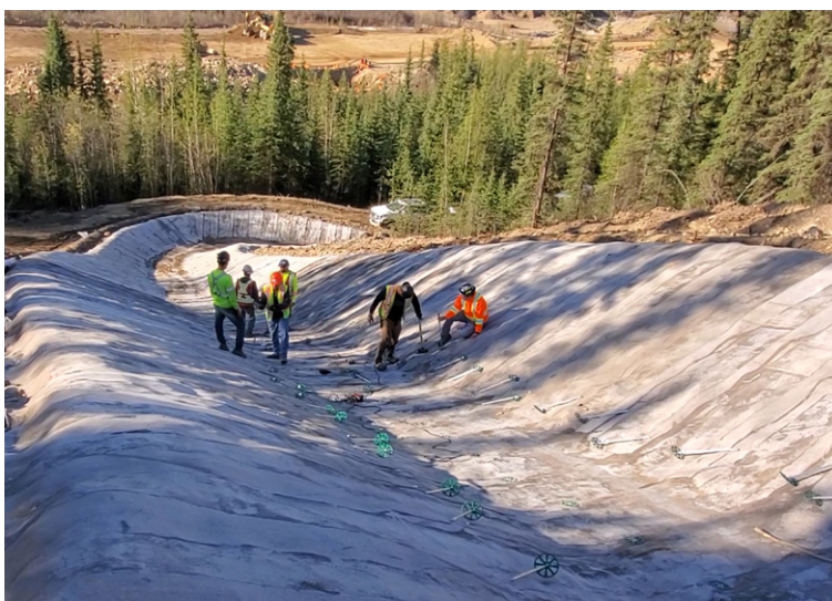
Installation of percussion anchors on emergency spillway section
