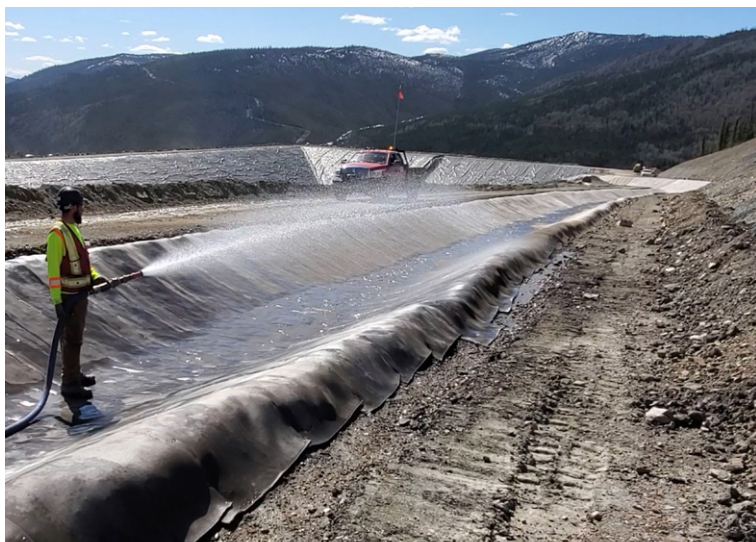
Hydration of the lined channel
