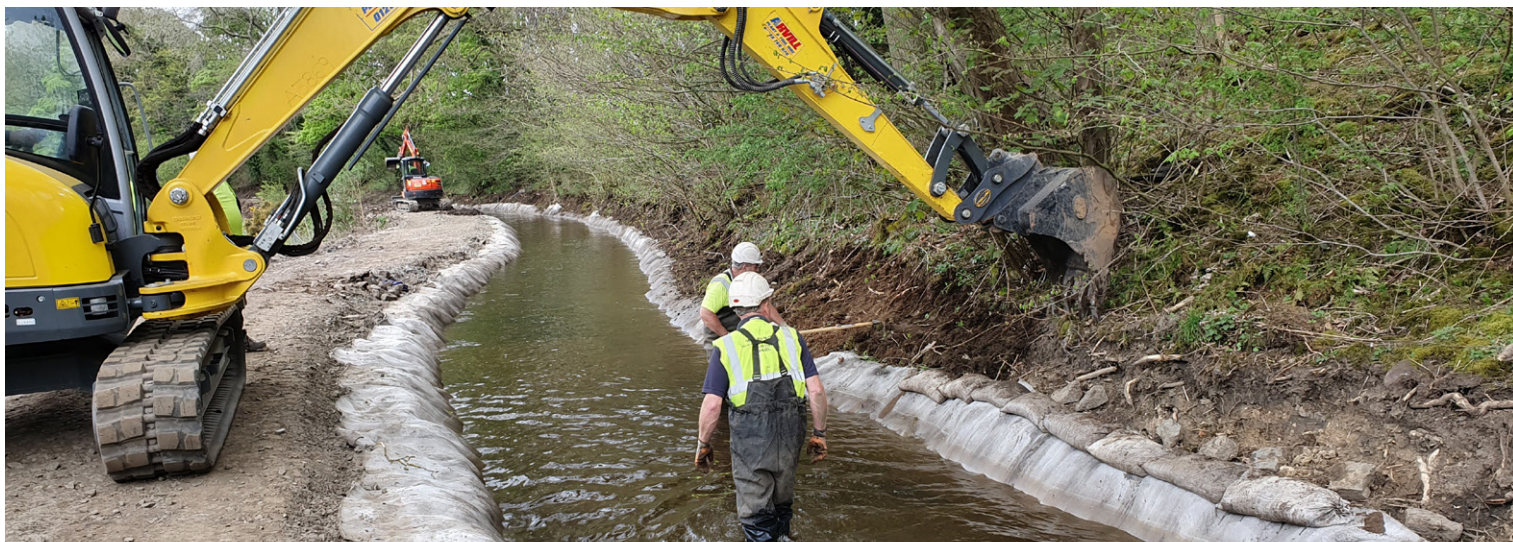
Backfilling anchor trenches
