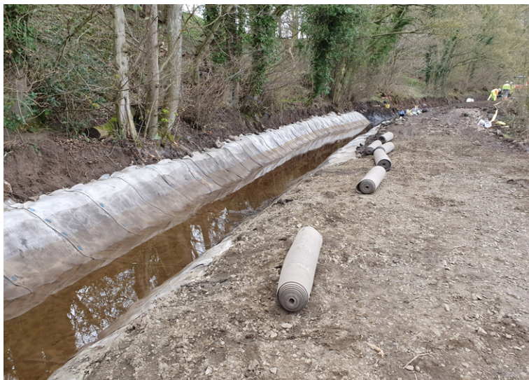
CC8 cut to length and staggered along the channel
