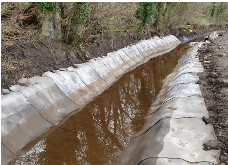
CC laid transversely and benched on either side
