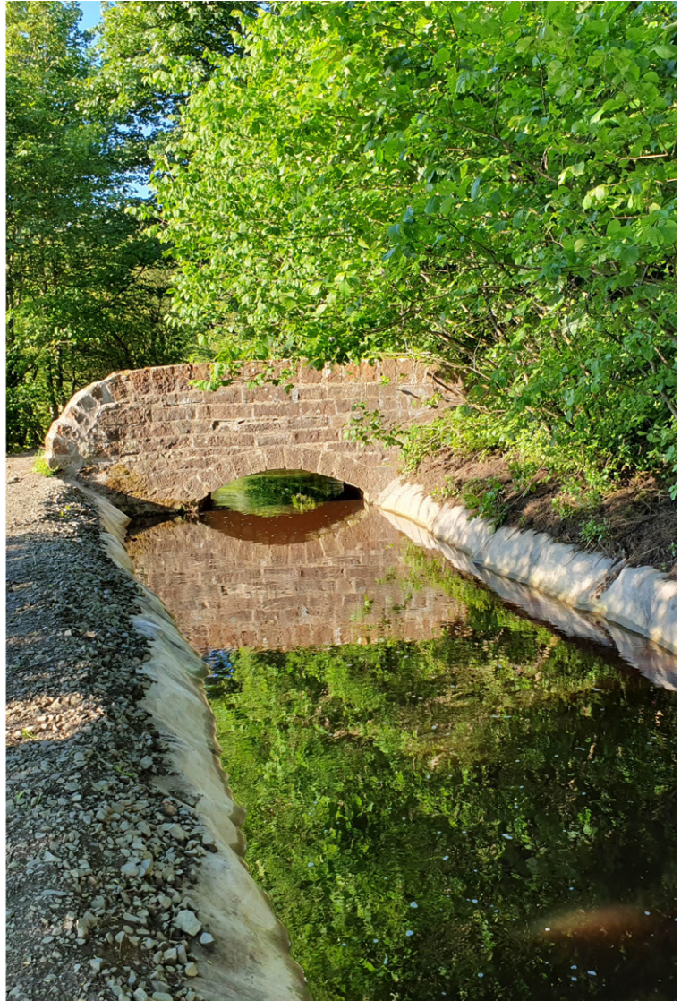
Left: Before - overgrown channel leading to masonry bridge / Right: After - CC lined channel leading into masonry bridge
