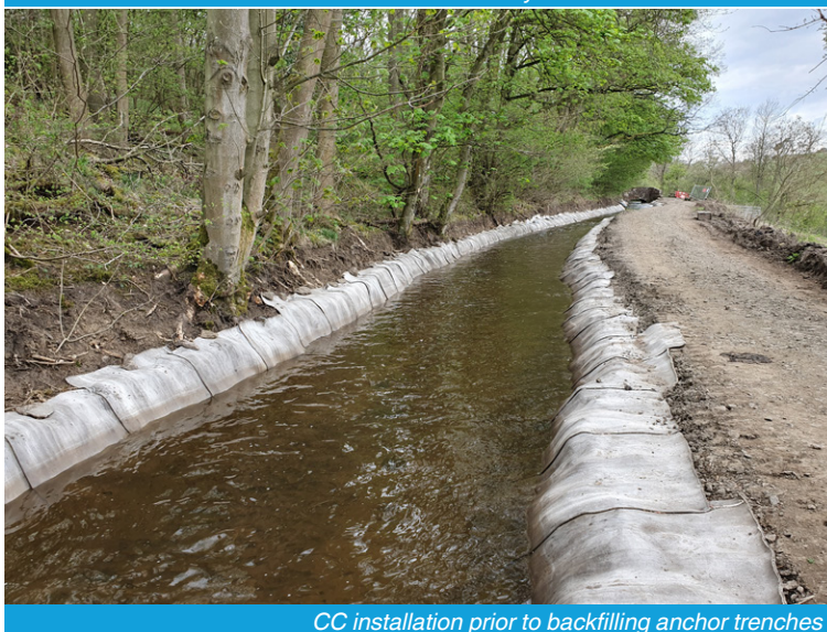
CC laid transversely and benched on either side
