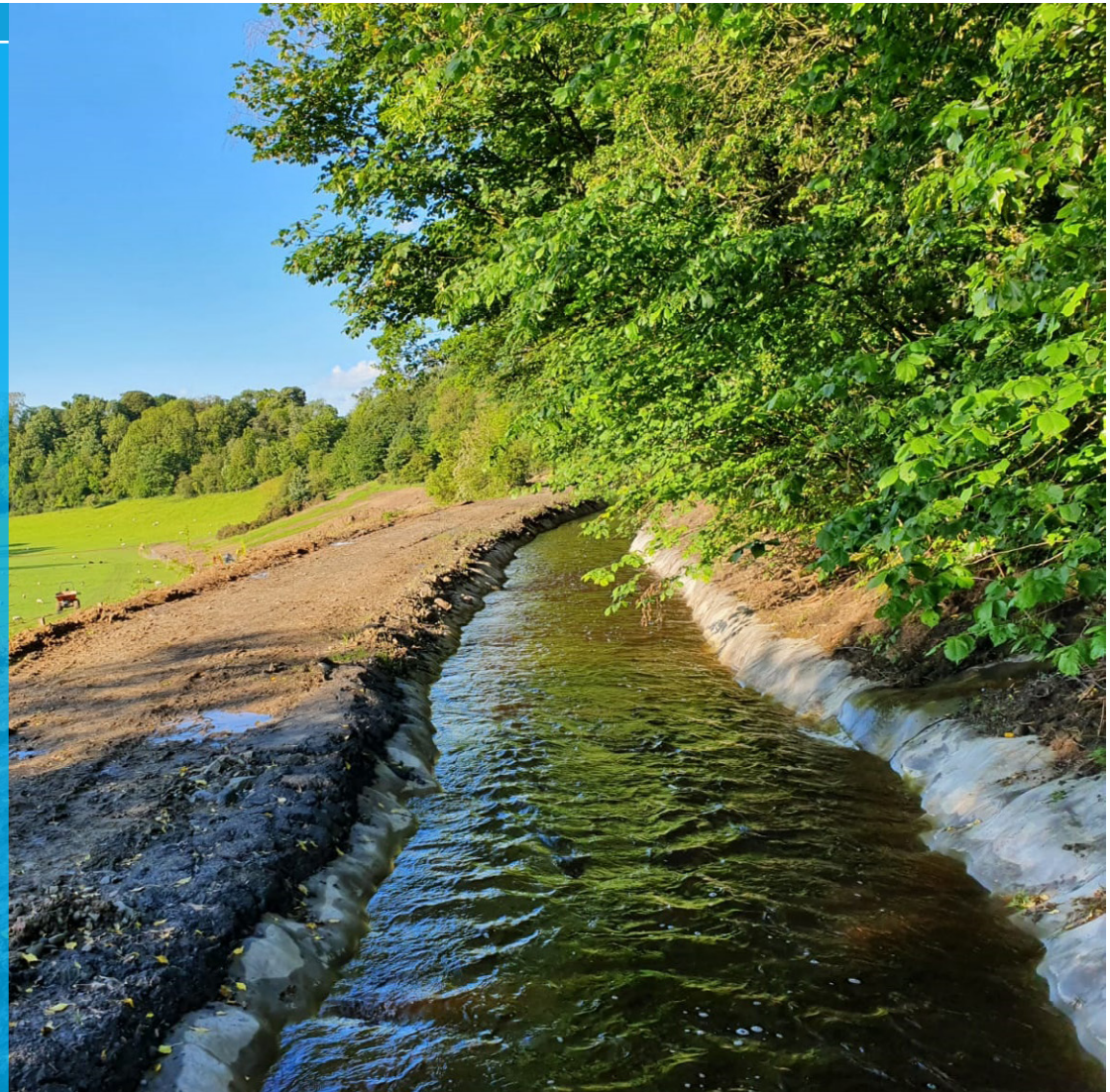
Completed CC installation at the Scottish Canals Almond Feeder
