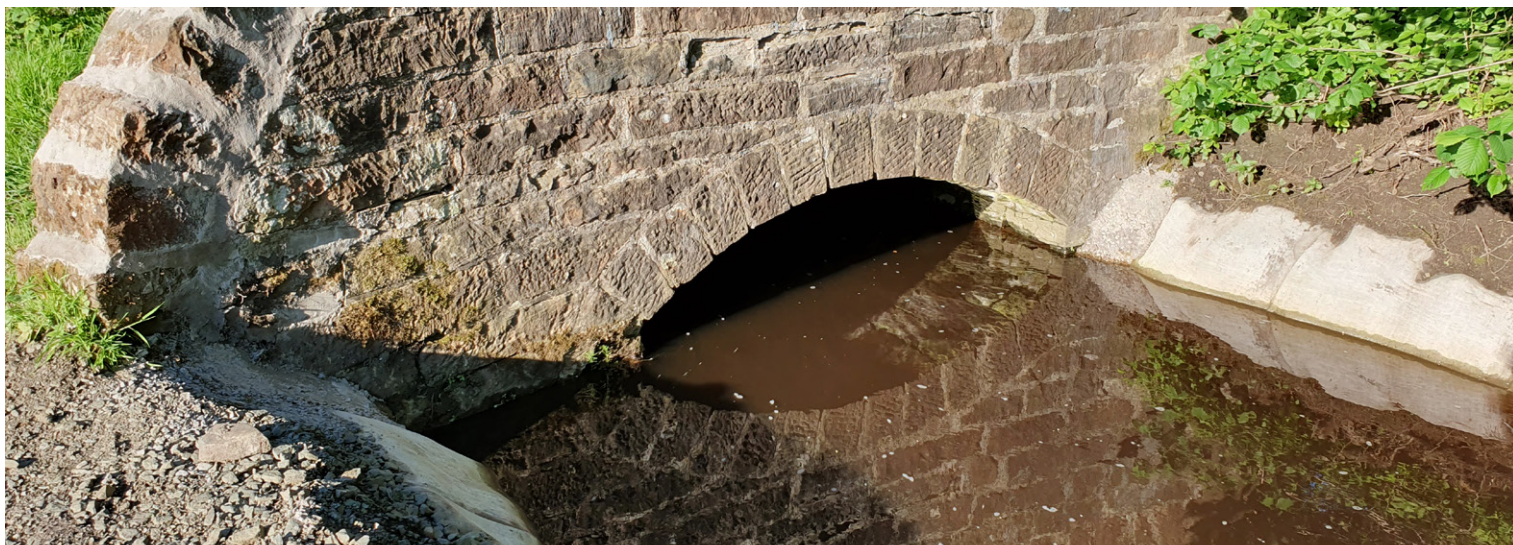
CC termination at masonry arch
