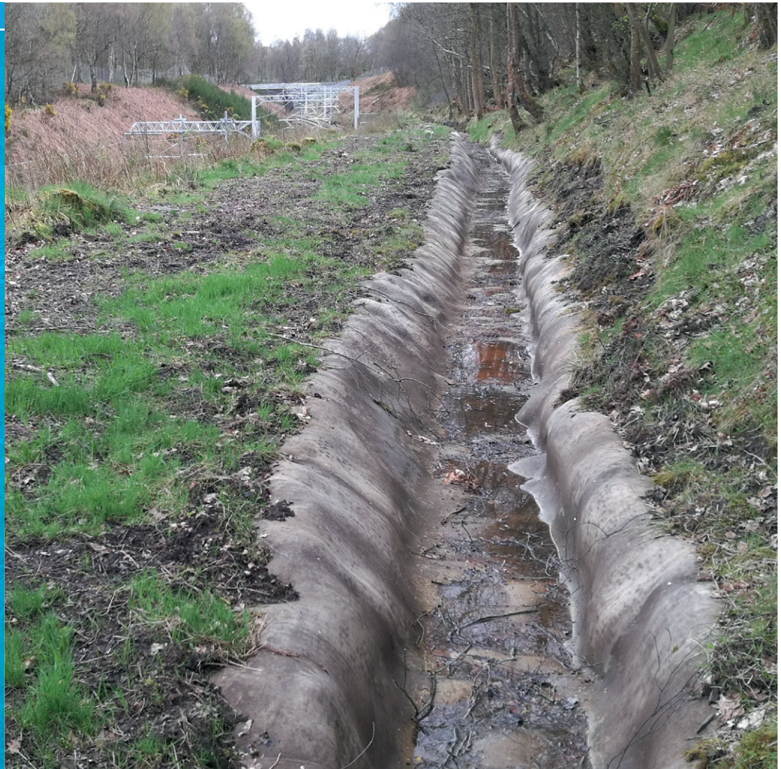
Completed CC lined channel in Falkirk, Scotland
