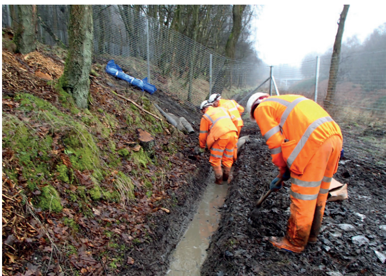
Anchor trenches excavated with hand shovels
