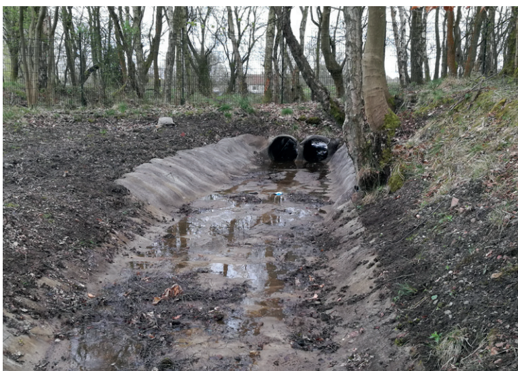
CC lined channel diverted water into two large culverts
