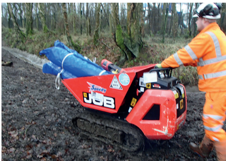
Batched rolls delivered using JCB tracked mini dumper
