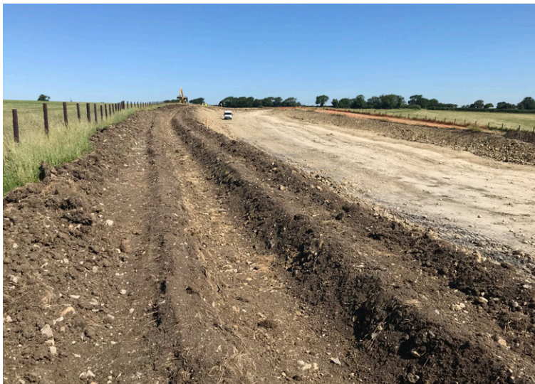
Channel profile following excavation
