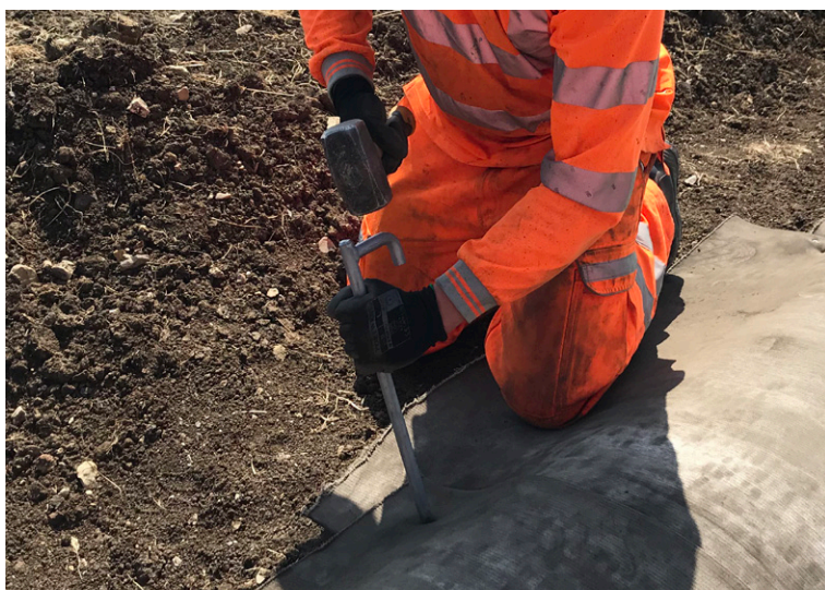
Edges of CC material secured using ground pegs
