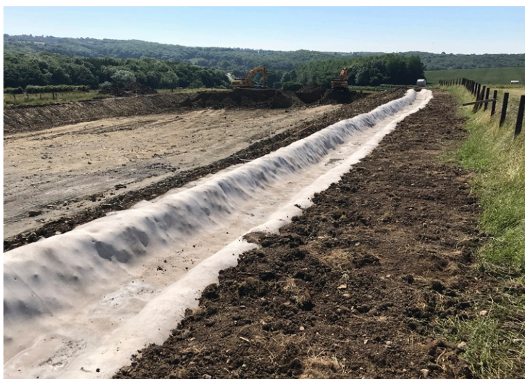
Anchor trenches backfilled for neat termination and to prevent ingress
