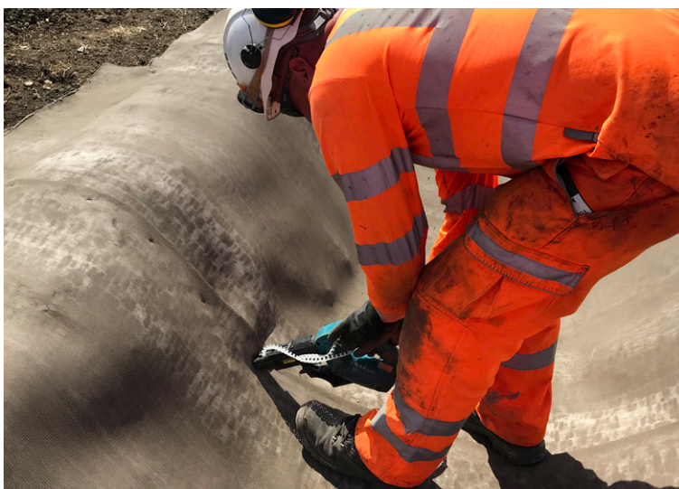
Stainless steel screws used to joint CC overlaps
