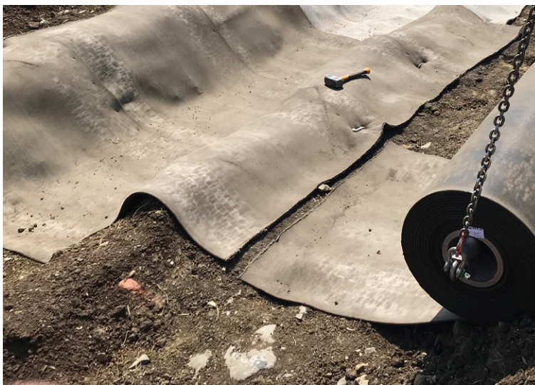
CC deployed from spreader beam, cut to required length
