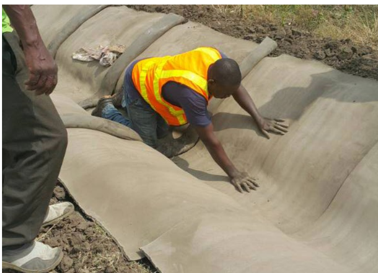
The CC™ was laid transversely
