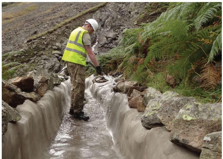
Hydration taking place via an army issue portable 10,000 ltr reservoir
