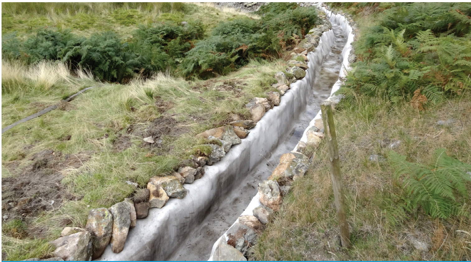
The completed lined channel at Glenridding, Ullswater
