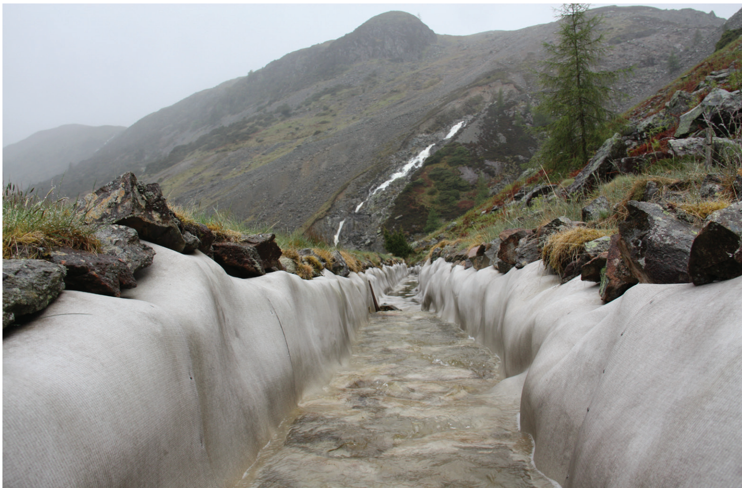
An aged image (May '17) of the completed lined channel at Glenridding, Ullswater
