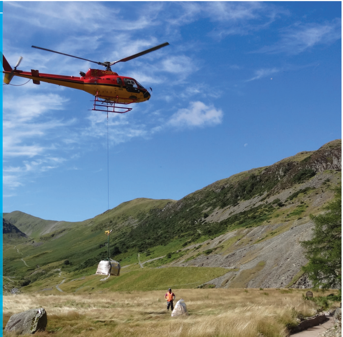
Batch & Bulk Rolls of CC being delivered via a commercial helicopter
