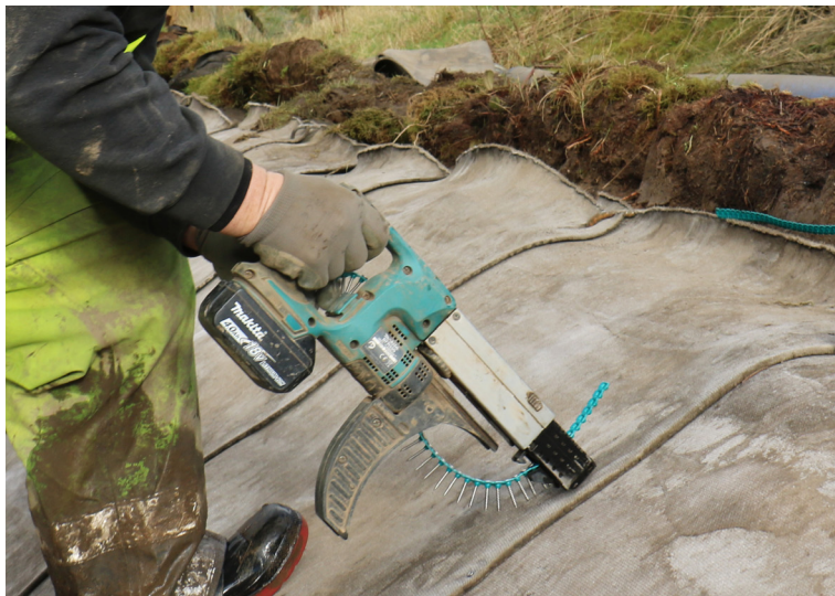
Joining adjacent layers of CC with an autofed screw driver
