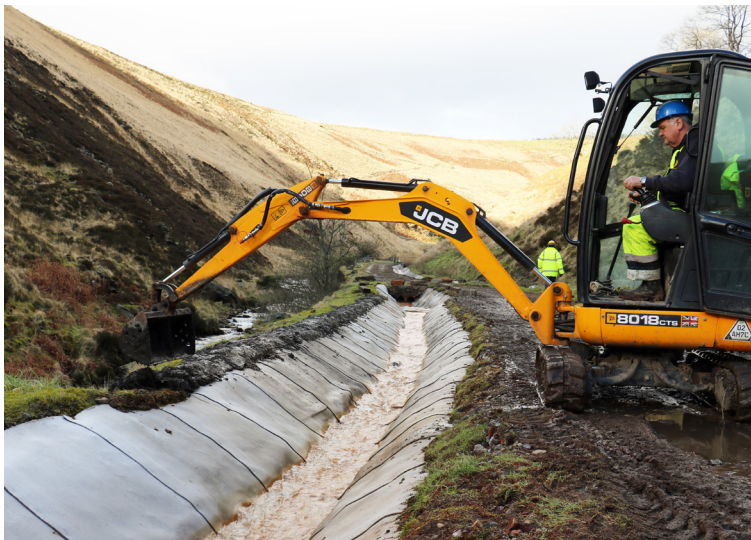
Backfilling anchor trenches after hydration of CC
