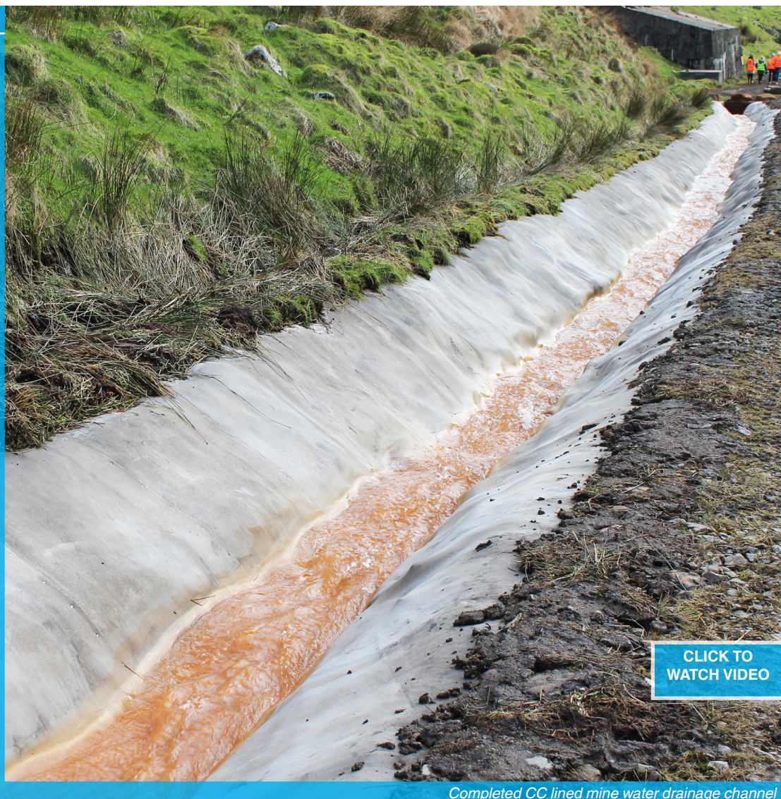
Completed CC lined mine water drainage channel
