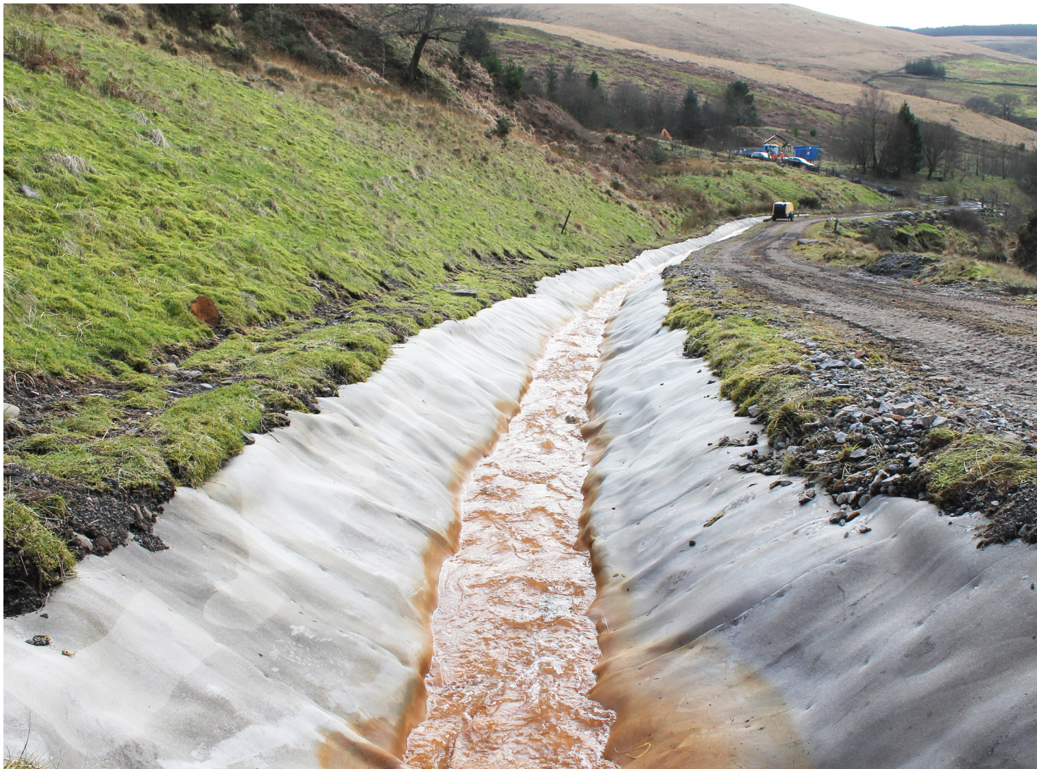
Completed CC lined mine water drainage channel
