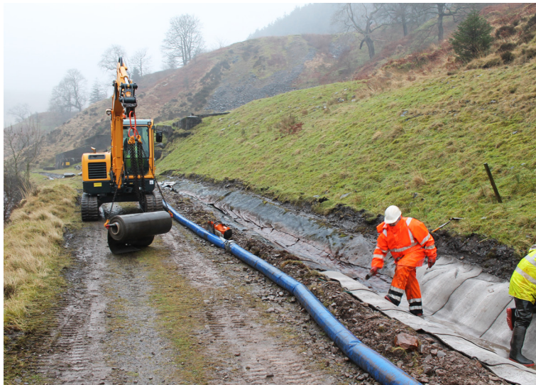
Deployment of CC8™ material in bulk rolls via spreader beam equipment
