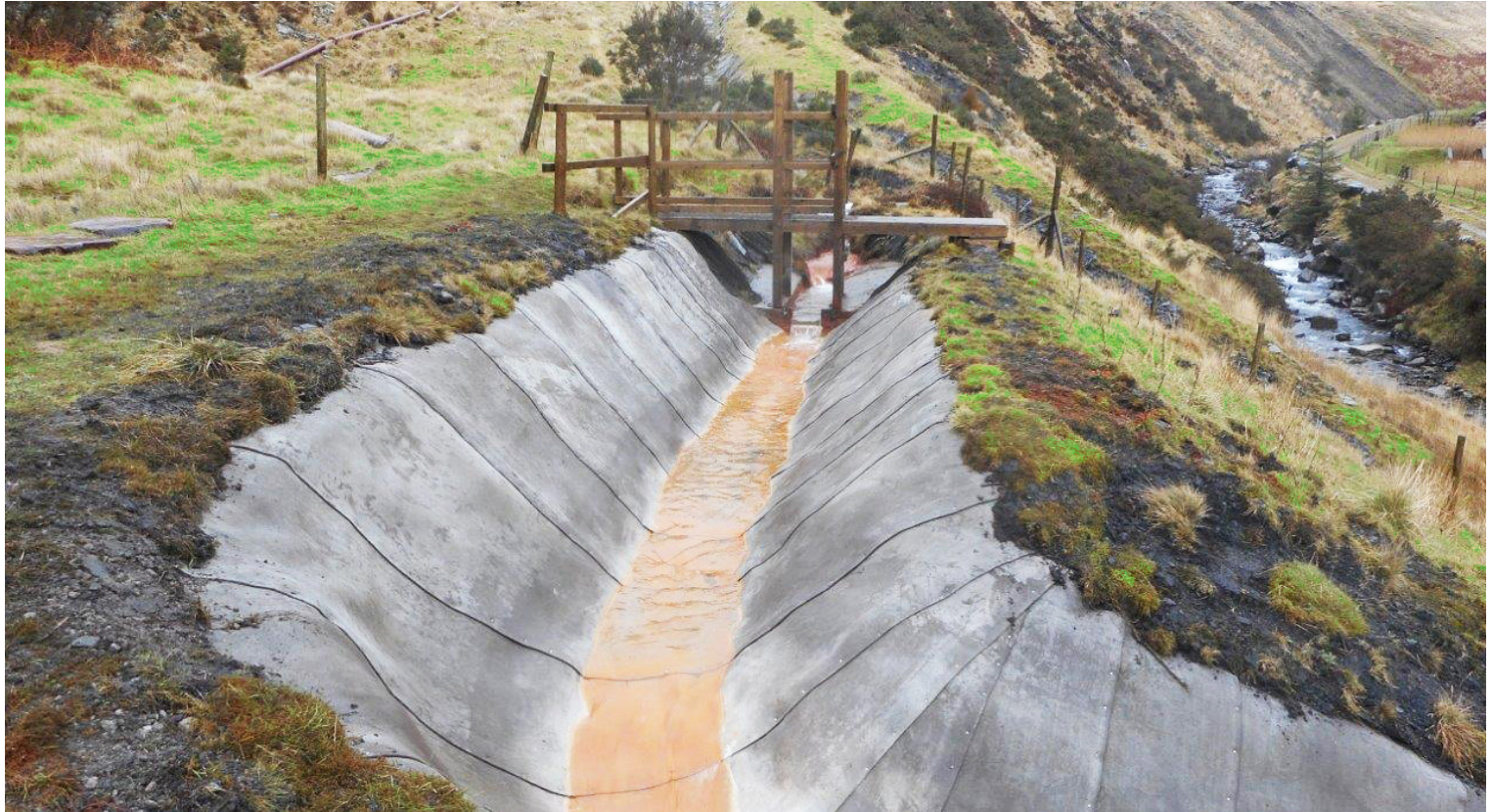
Section of channel inaccessible by plant which would have been impossible to line with conventional concrete methods
