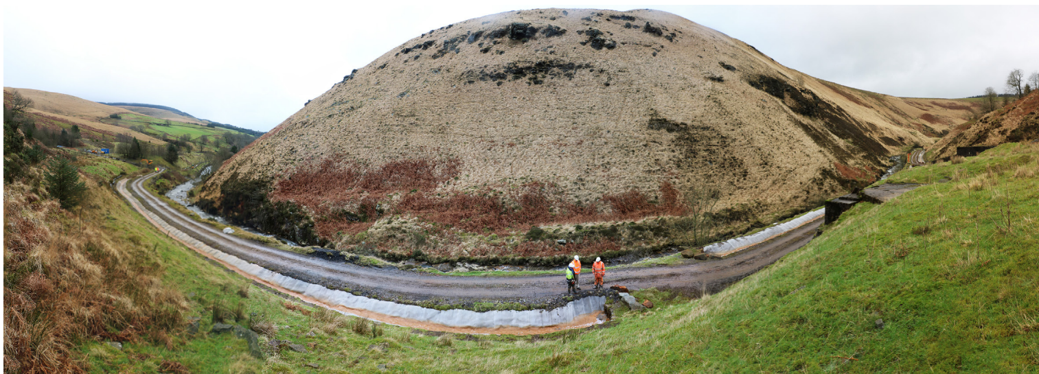
Completed north section of CC lined drainage channel network
