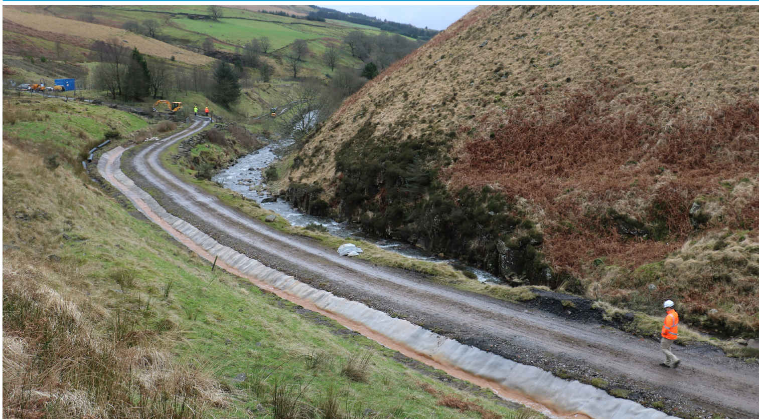
Completed section of CC lined mine water drainage channel
