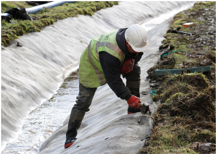
Fixing of CC layers within an anchor trench using steel ground pegs
