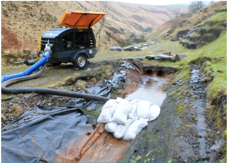
Temporary damming of channel sections prior to CC installation
