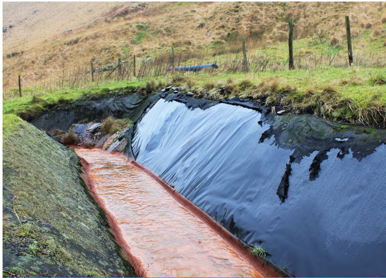
Ditch section showing deteriorated geotextile and LLDPE liner beneath
