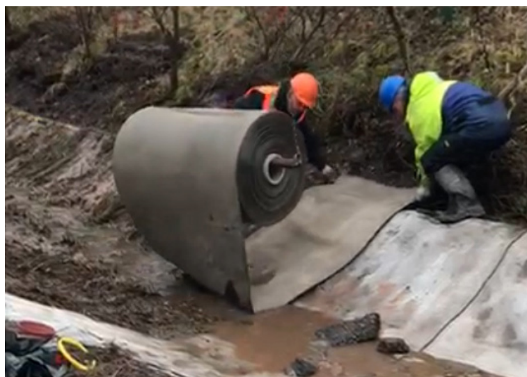
CC was laid transversely across the channel
