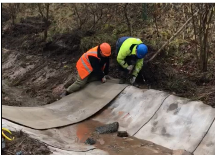
CC was fixed in anchor trenches using ground pegs
