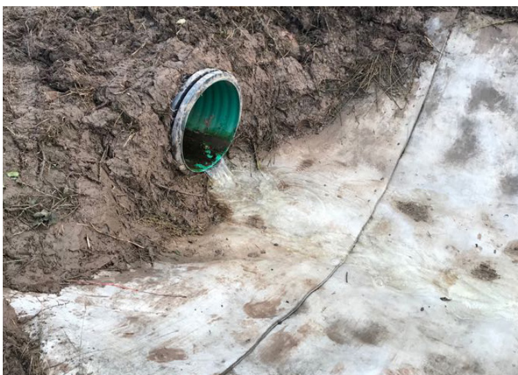
Channel termination detail
