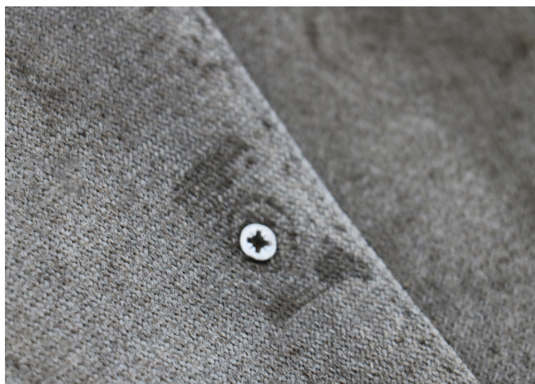
Screws were used to joint overlaps
