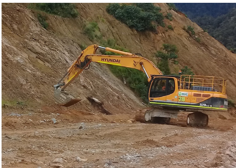
Excavator used to prepare channel
