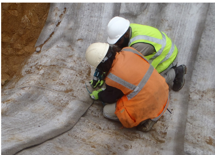
Joining CC overlaps
