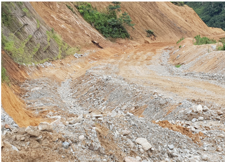
Channel profile cut from substrate
