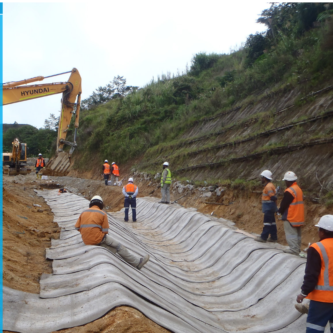
Installation of CC at Hidden Valley Gold Mine in Papua New Guinea
