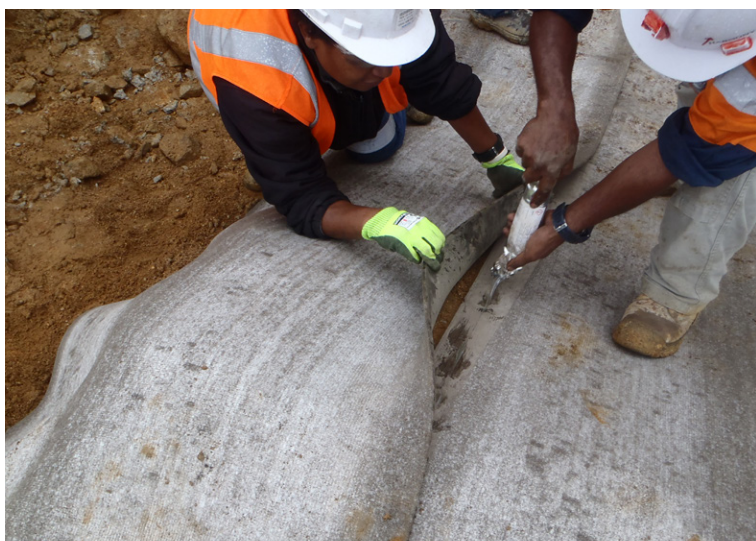
Applying sealant to CC overlaps
