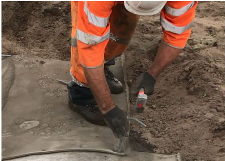
CC edges captured in anchor trenches using ground pegs
