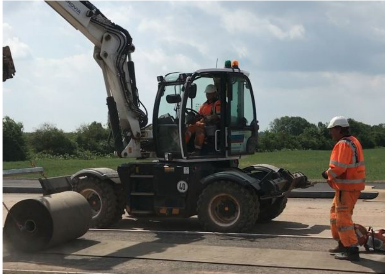
CC unrolled using spreader beam and excavator and batched road-side
