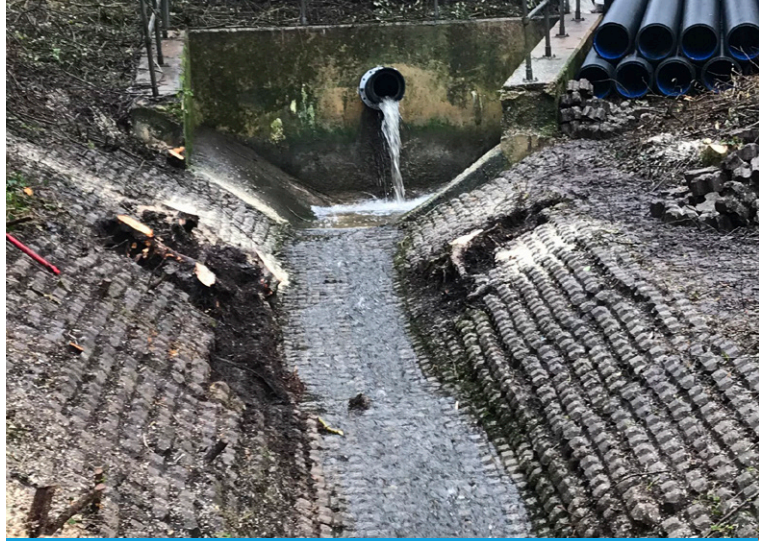
Trees cut out of concrete block channel
