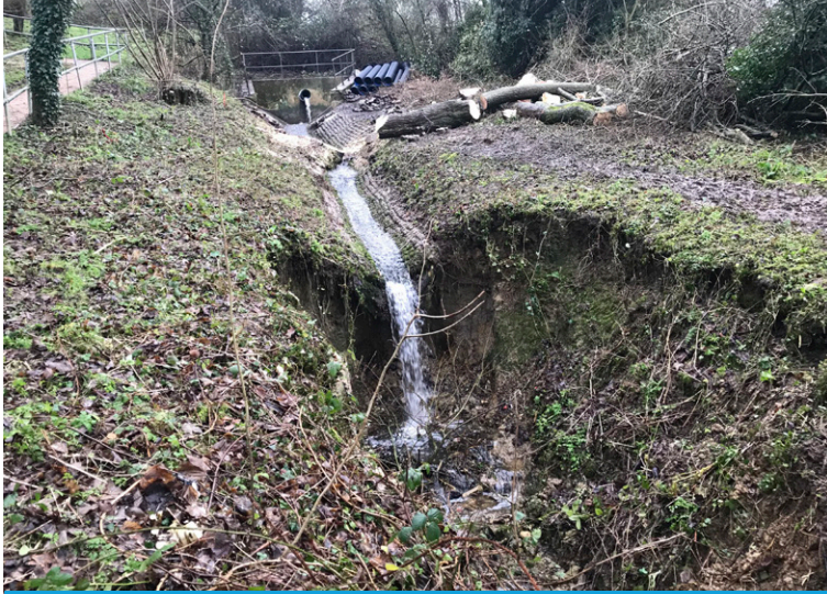
Scour hole created by undermining of concrete block system
