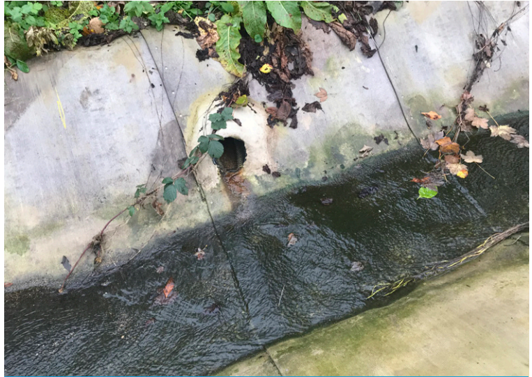
Grouted pipe detail
