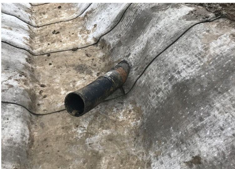
Section of channel installation prior to backfilling
