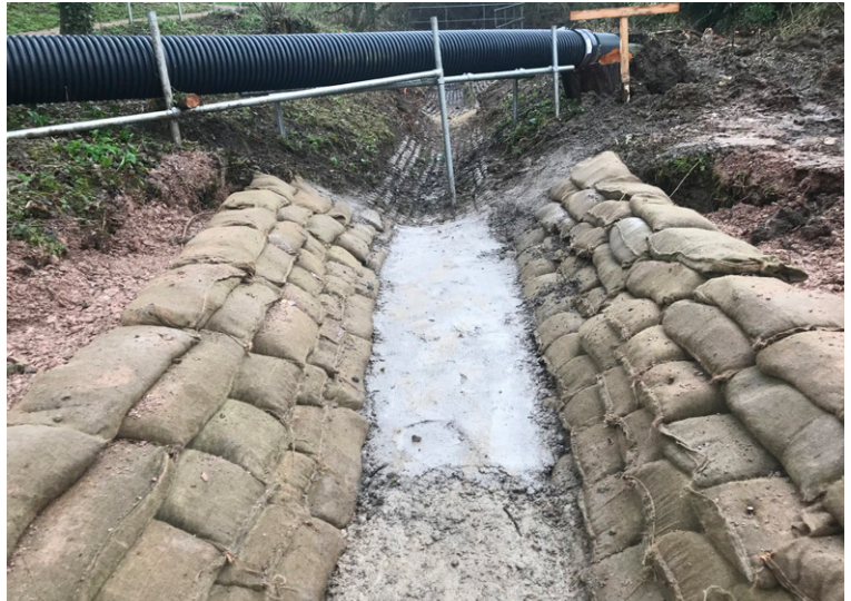
Scour filled with clay and channel formed using sandbags and concrete blinding
