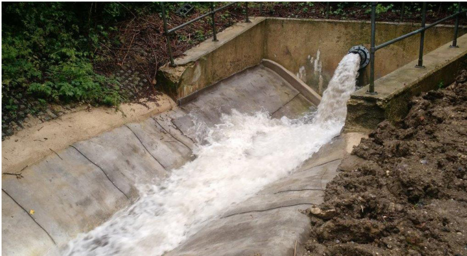
Channel in full flow with velocities up to 8ms -1
