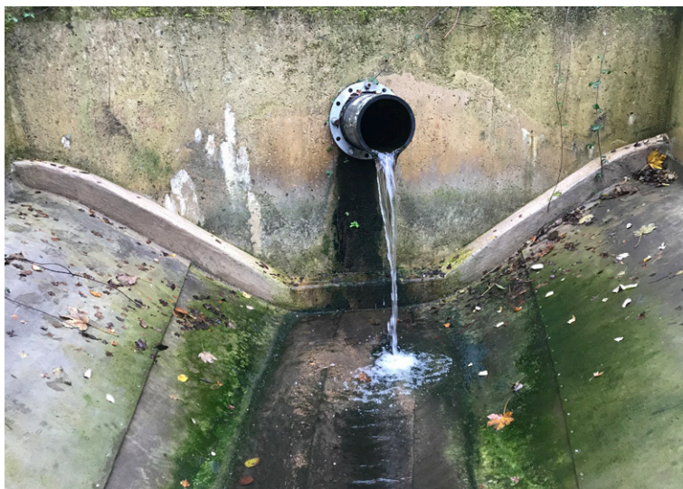
Poured concrete fillet at interface with headwall
