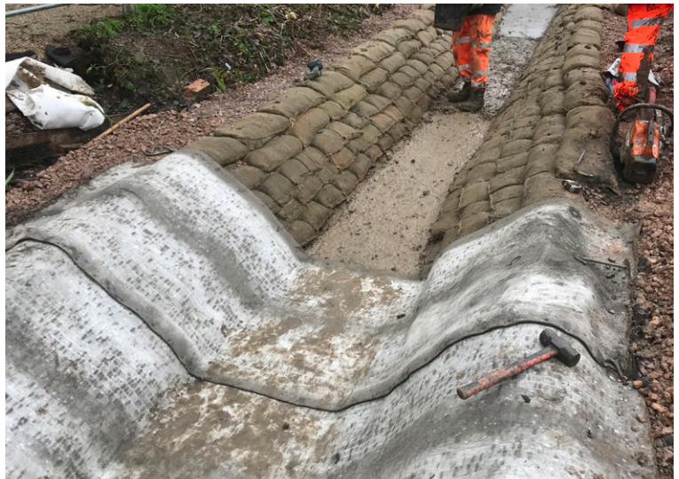
CC installed over concrete blocks and sandbags
