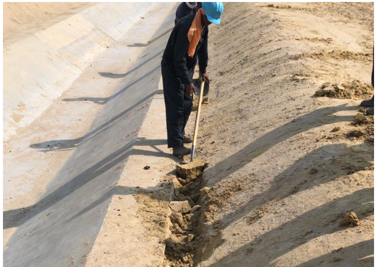
Anchor trenches dug by hand at toe of slope
