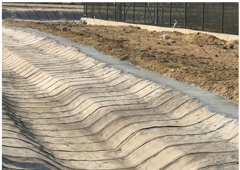
Anchor trenches backfilled with poured concrete
