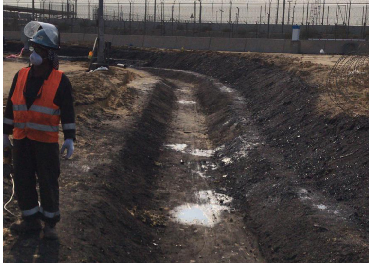
Channels were excavated and profiled prior to works
