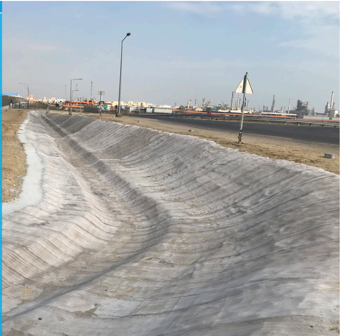
Completed channel lining installation
