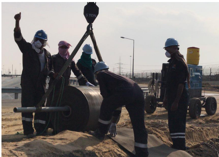
CC deployed via spreader beam
