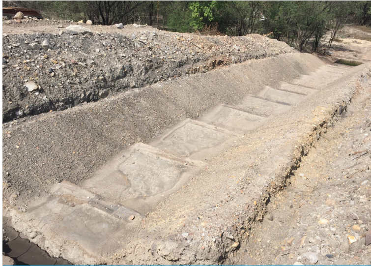
The area was graded after vegetation, loose soil and rock removal
