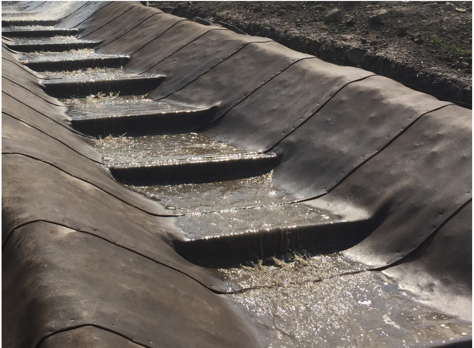
The Dissipater Channel during hydration
