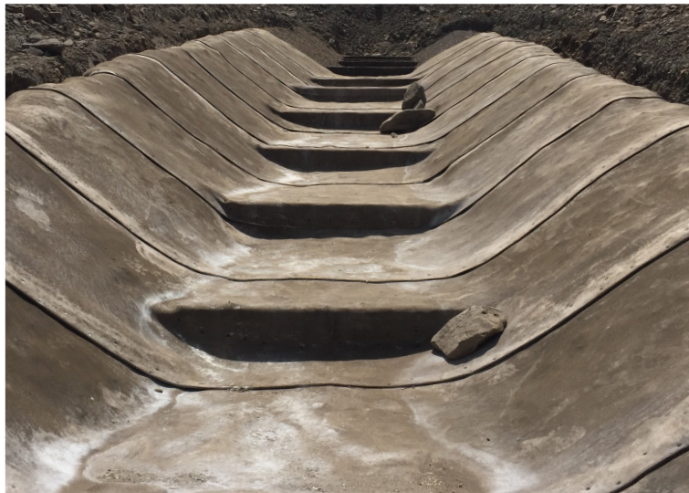
Wood screws were used to secure the CC to the wooden baffling
