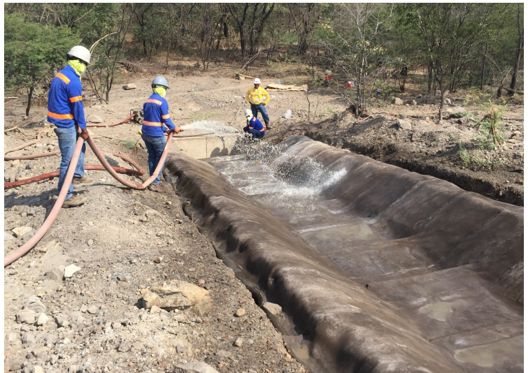
A 1000 litre on-site water tank was used for hydration
