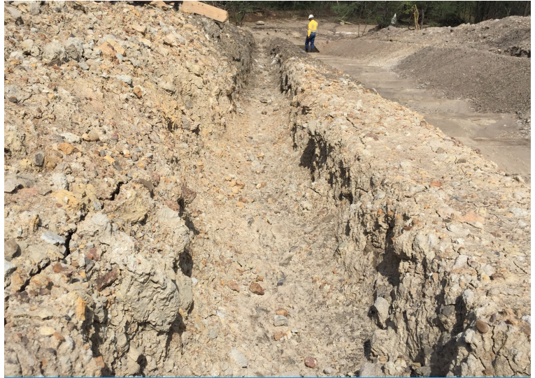
Anchor trenches were dug parallel to the channel
