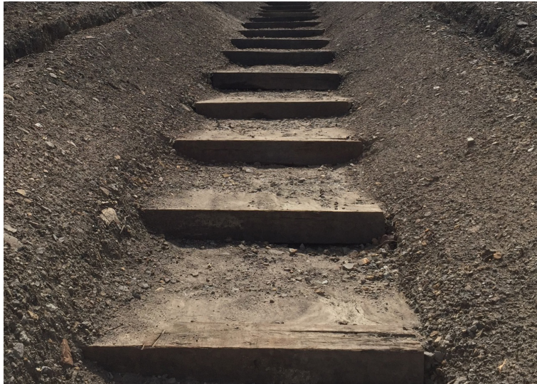
1.4m transverse wooden bafflings were inserted every 1.2m
