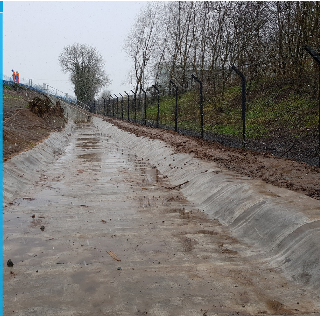
Completed CC lined channel
