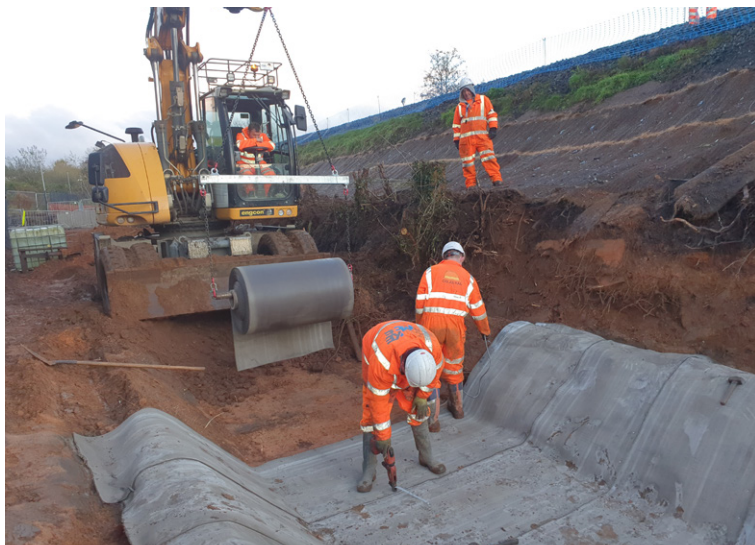
Hydrating underneath the overlap & screwing CC overlap at 200mm centres
