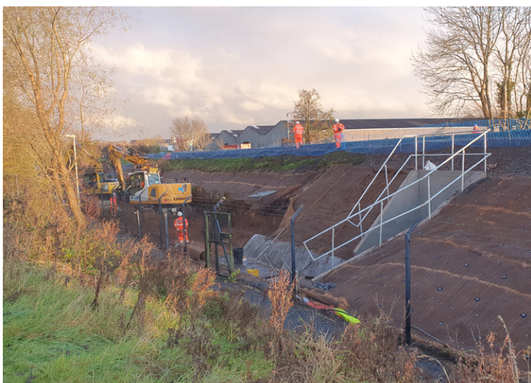
Channel excavation adjacent to railway track
