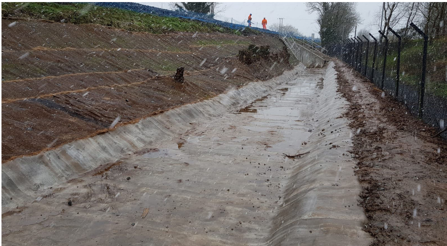
Completed CC lined channel - works were carried out despite inclement weather and restricted site access
