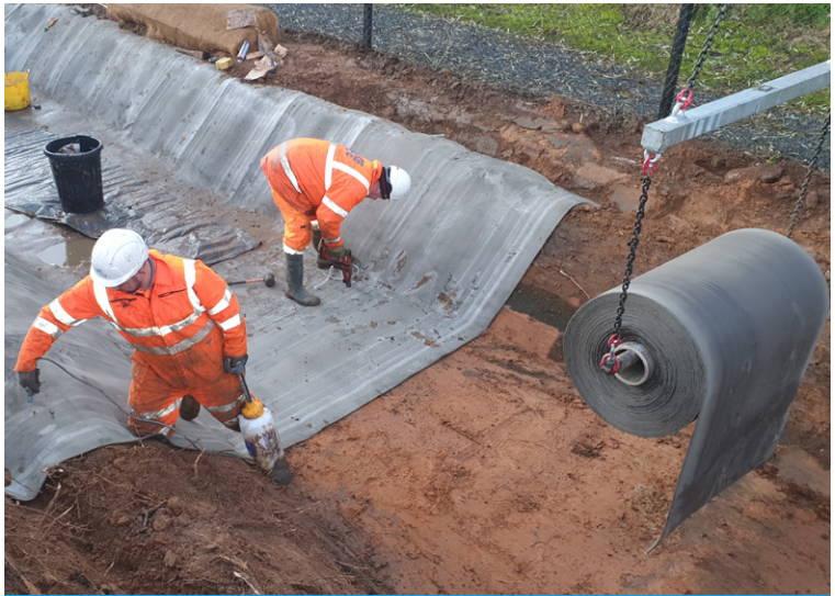
CC8 bulk roll dispensed on spreader beam
