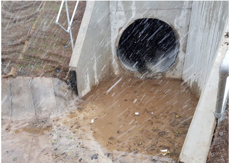
Precast headwall - CC interface
