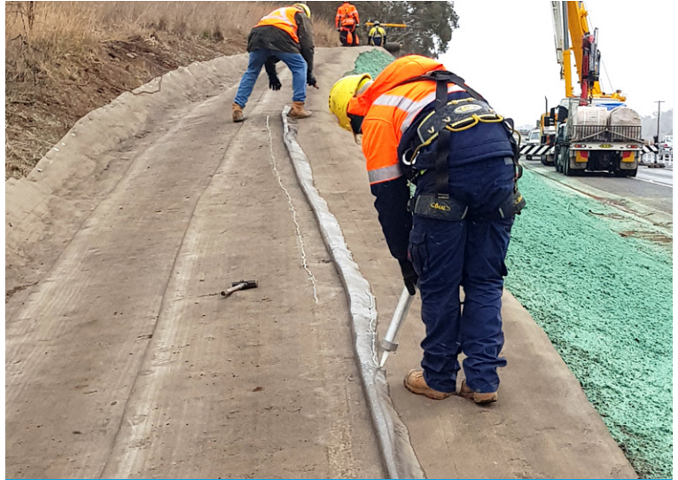
Application of sealant to joints
