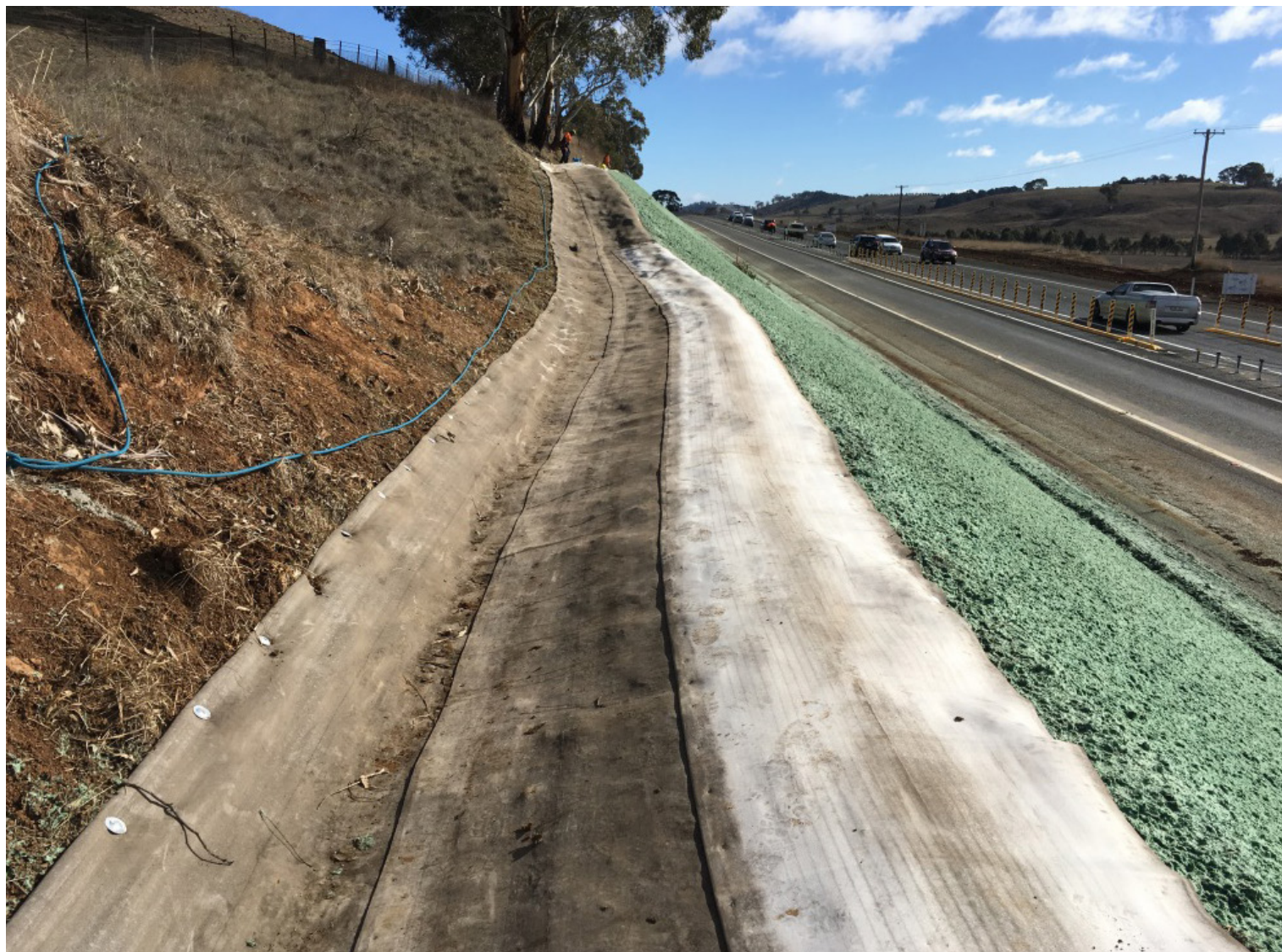
Completed section of CC lined drainage channel prior to anchor trench detailing
