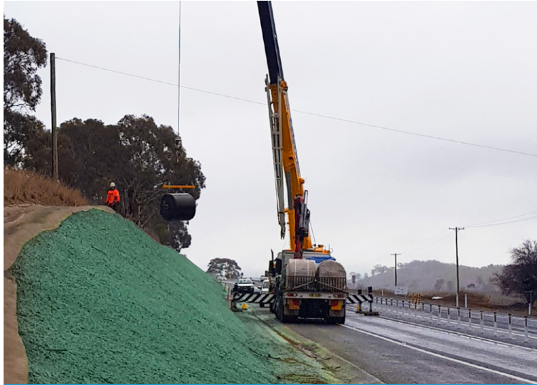
Deployment of CC5 bulk roll
