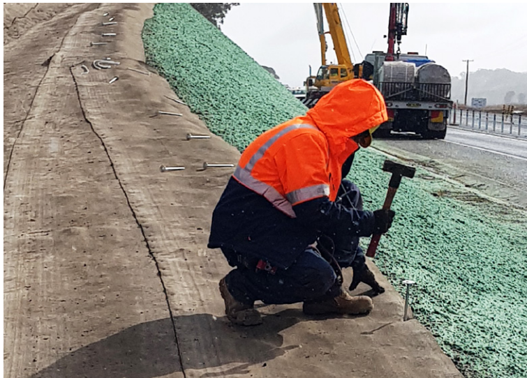
Fixing CC with pegs
