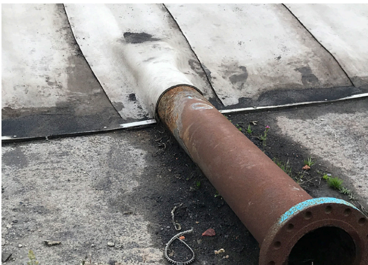
CC was able to easily accomodate existing pipes and other infrastructure
