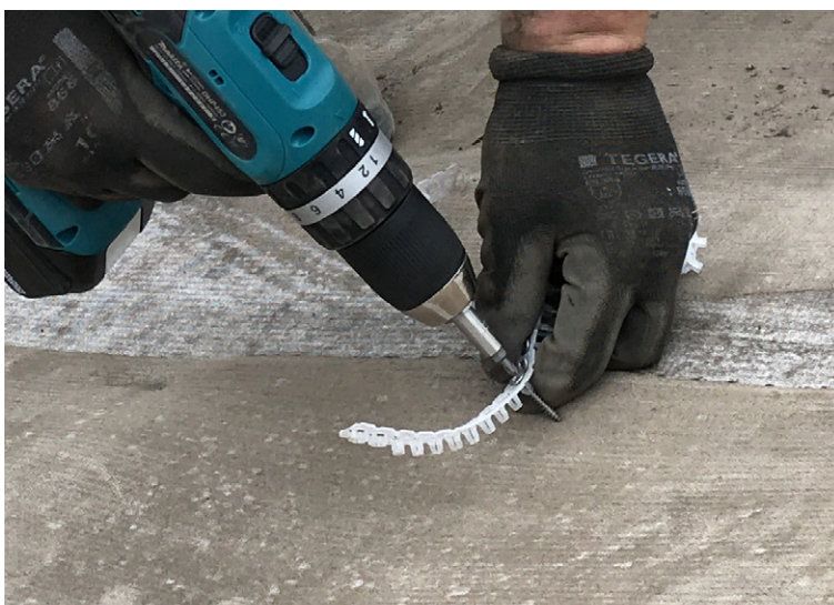
CC overlaps were jointed using stainless steel screws
