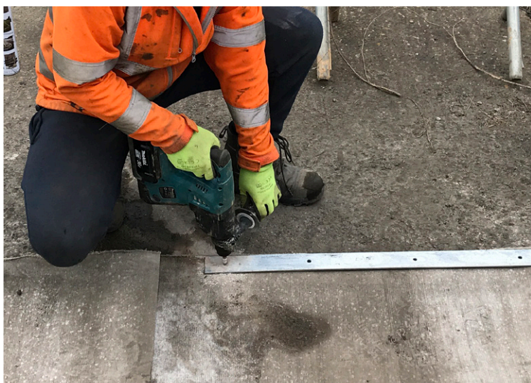
Termination of CC at existing concrete using steel bars and masonry bolts
