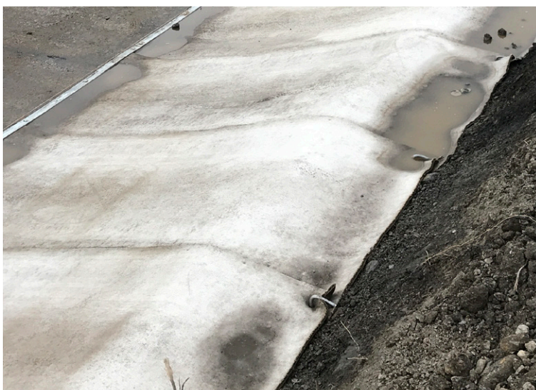
Edges secured using ground pegs
