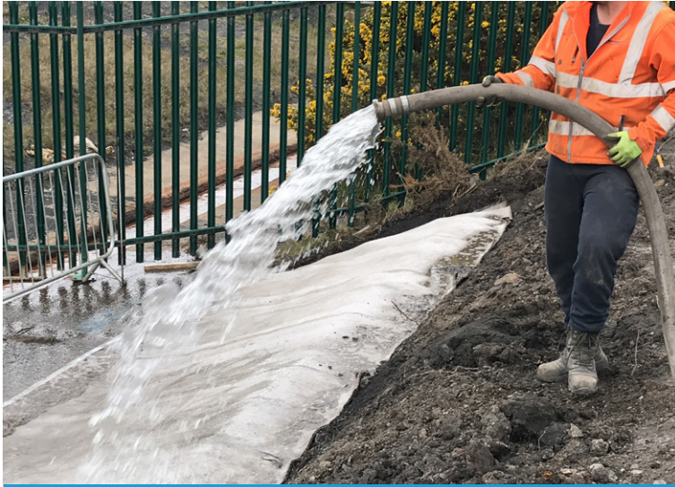
Hydration of CC following installation
