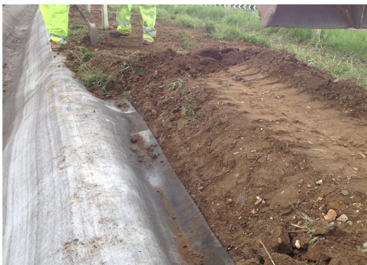
CC was pinned in anchor trench before being backfilled
