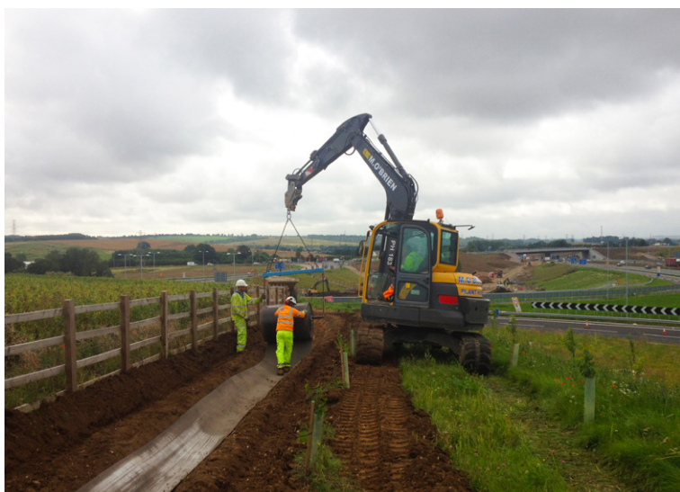
Deployment of CC via spreader beam
