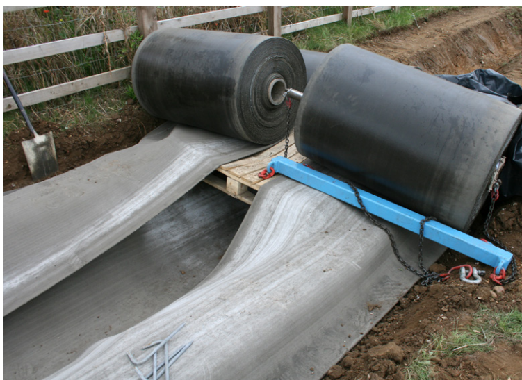
3 layers were laid longitudinally, with bottom layer laid first
