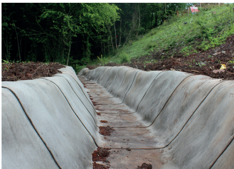
CC easily negotiated corners and changes in depth and profile
