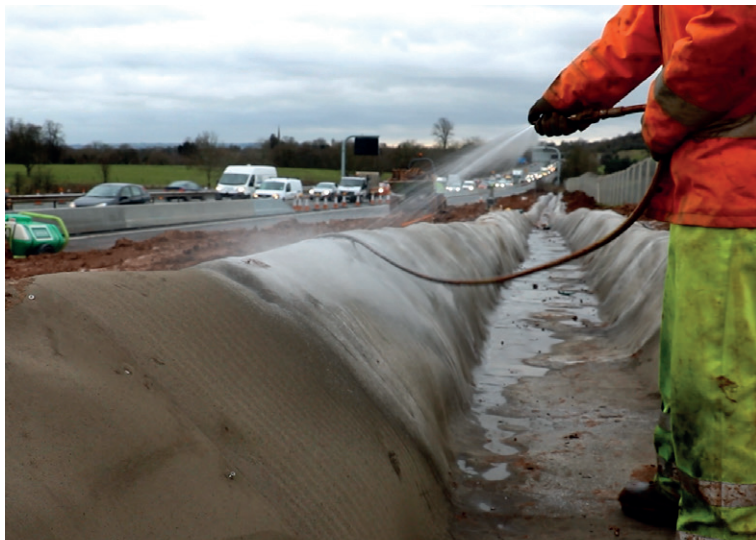
Hydration of deployed and fixed CC
