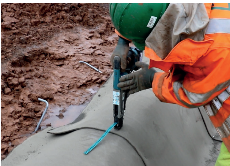
Jointing overlapped layers of CC using screws at 200mm centres
