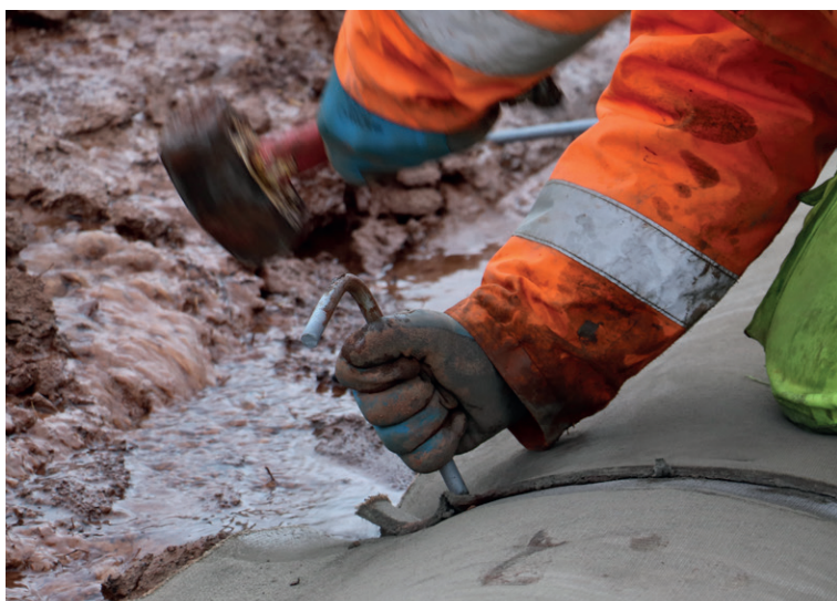
Fixing CC to substrate with 250mm ground pegs
