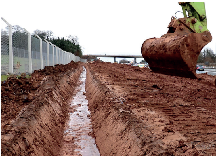
Grading of profile and deployment of type 1 aggregate
