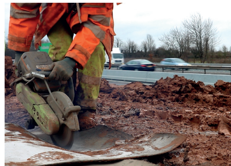
Cutting CC to length to reduce wasteage
