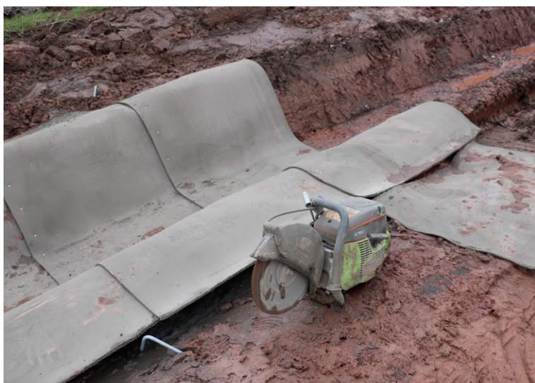
Layers of CC laid transversely to accomodate varying profile widths
