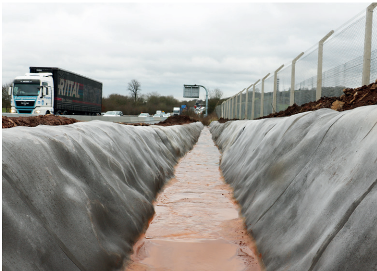
CC conforms to the substrate, greatly reducing preparation time
