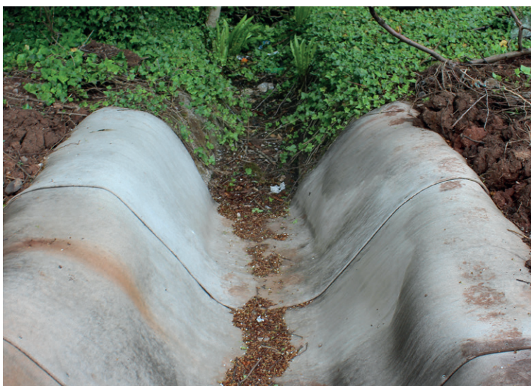
Ditch outfall collecting surface run-off from adjacent field
