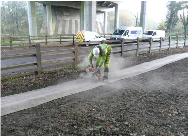
Cutting CC to length on site
