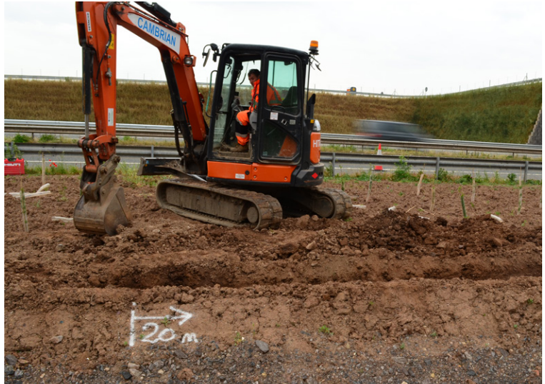
Preparation of anchor trenches
