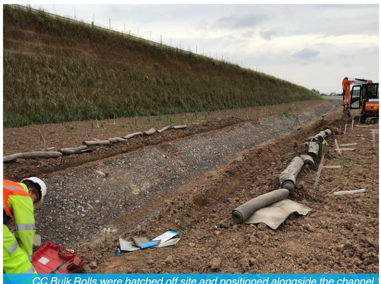
CC Bulk Rolls were batched off site and positioned alongside the channel
