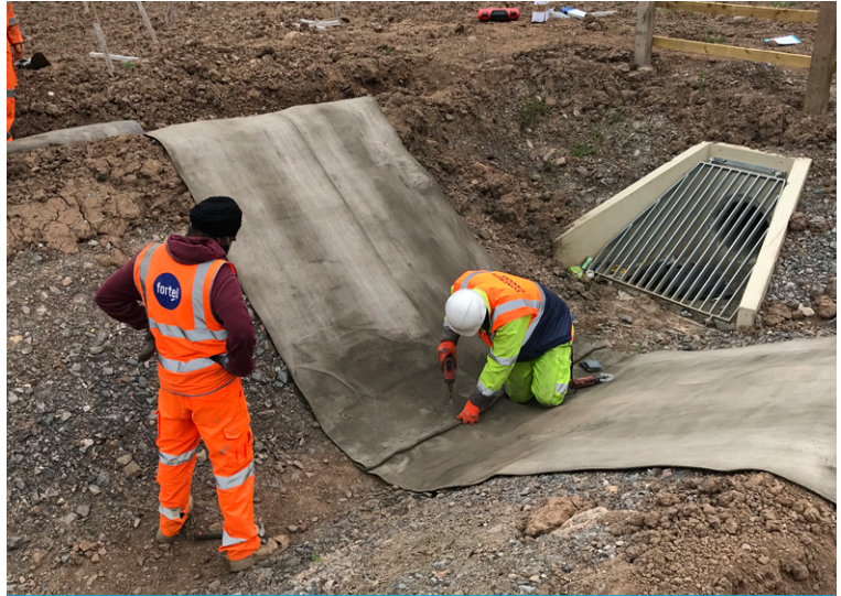
Joining the invert overlap
