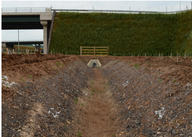
Channel profile excavated and graded
