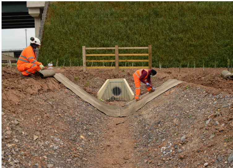
Subsequent lengths were overlapped and jointed with stainless steel screws
