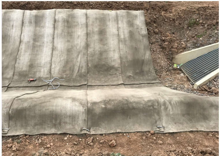
CC edges captured in the anchor trenches with ground pegs
