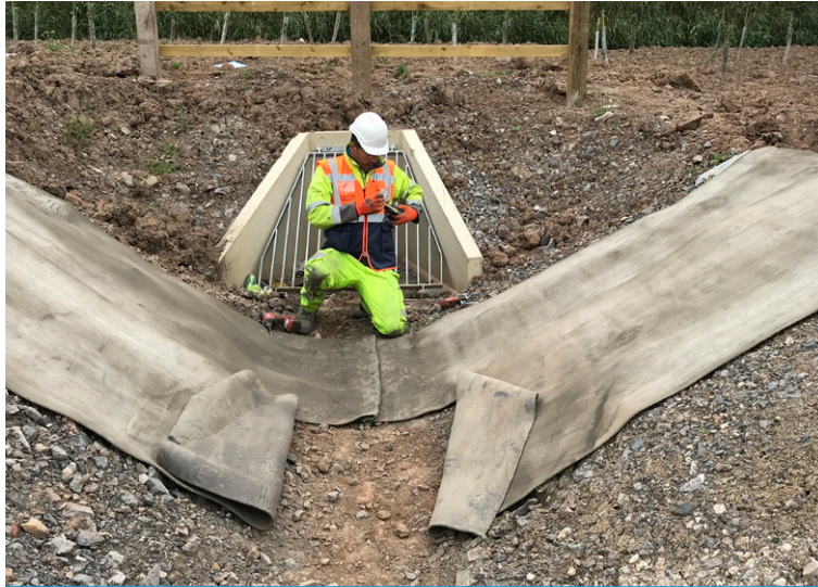
3 and 3.5m lengths of CC deployed down each channel side slope
