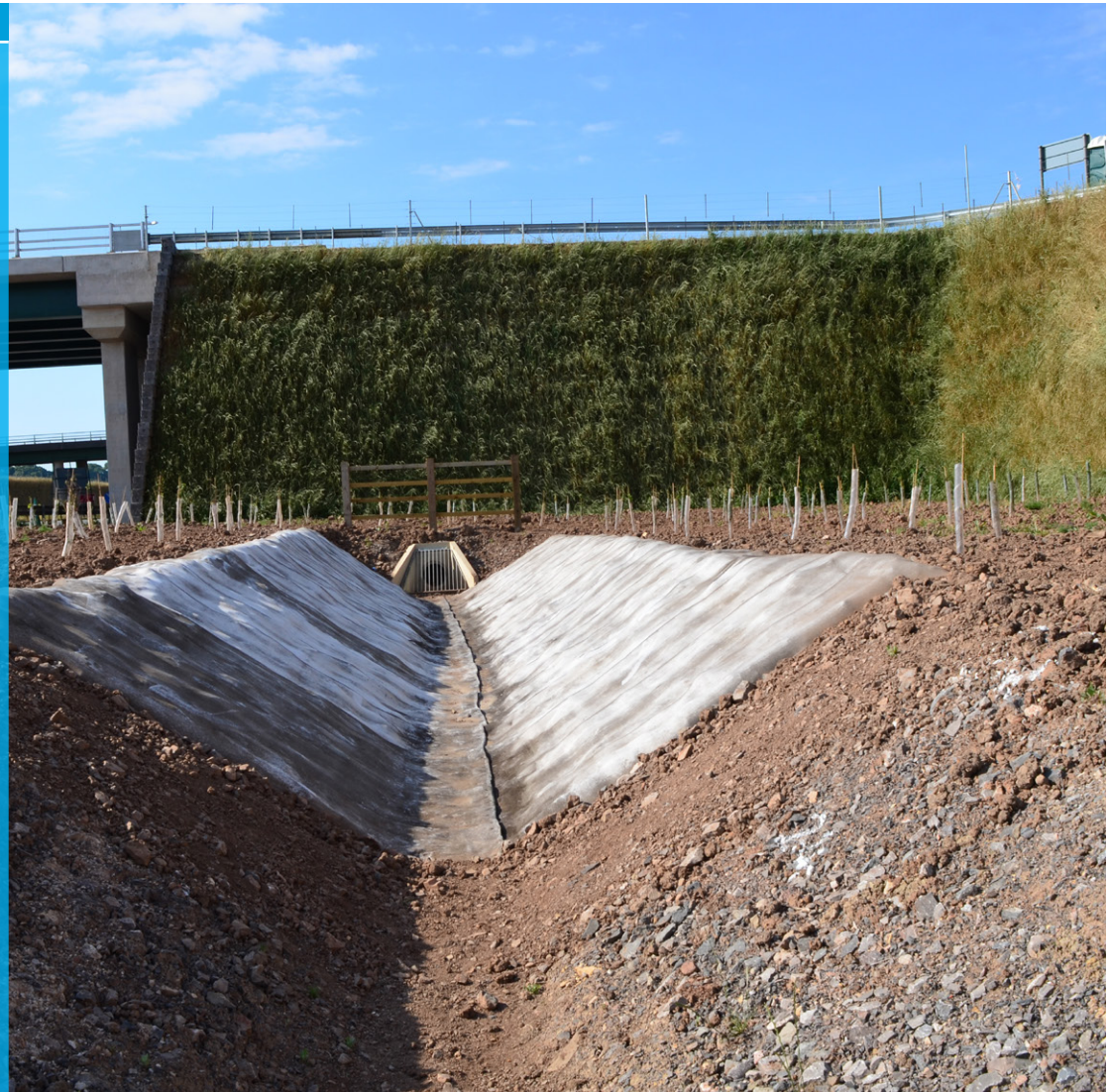
Completed CC lined drainage channel section alongside the new A49 Junction in Avonmouth
