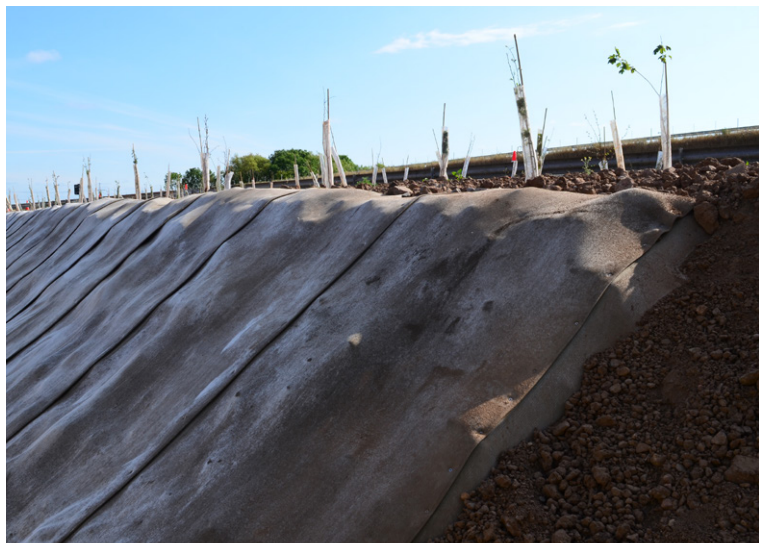
Termination detail at either end of the channel
