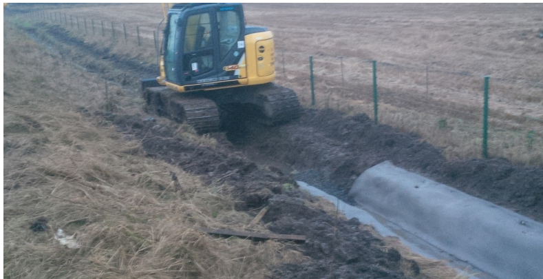
Excavation and laying CC
