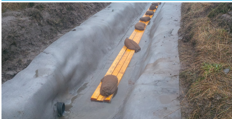
Weighing down joints and a pipe penetration
