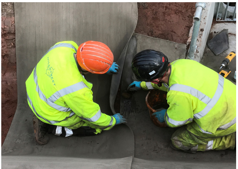
CC material hydrated under overlaps prior to jointing
