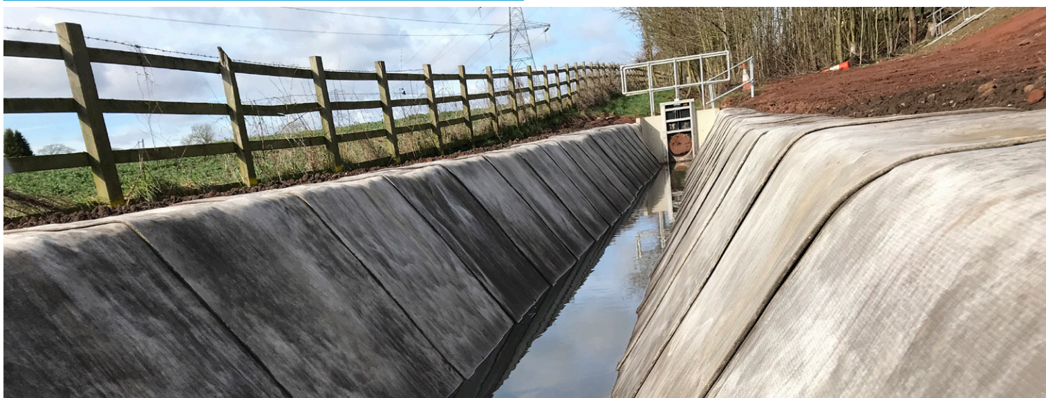
Completed ASC following backfilling of anchor trenches
