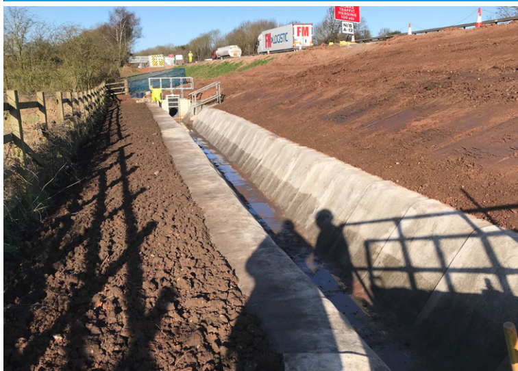
Completed ASC following backfilling of anchor trenches
