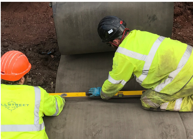
CC cut to length in-situ to minimise waste
