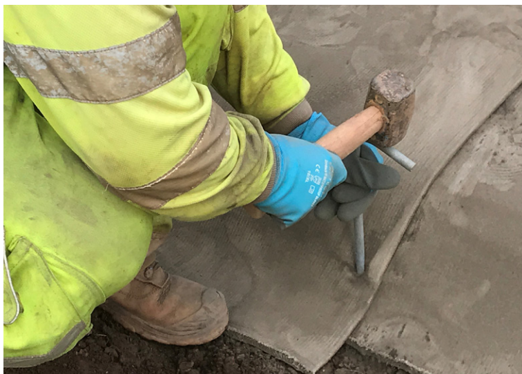
CC edges secured in anchor trenches using ground pegs
