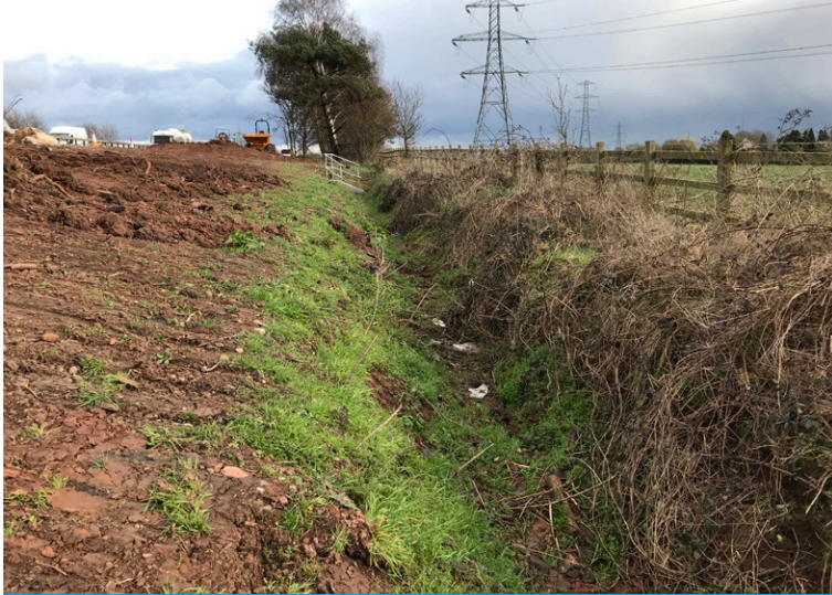
Original channel had suffered erosion and was overgrown
