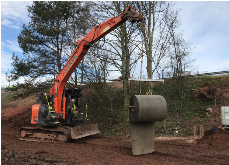
CC bulk rolls deployed from plant mounted spreader beam
