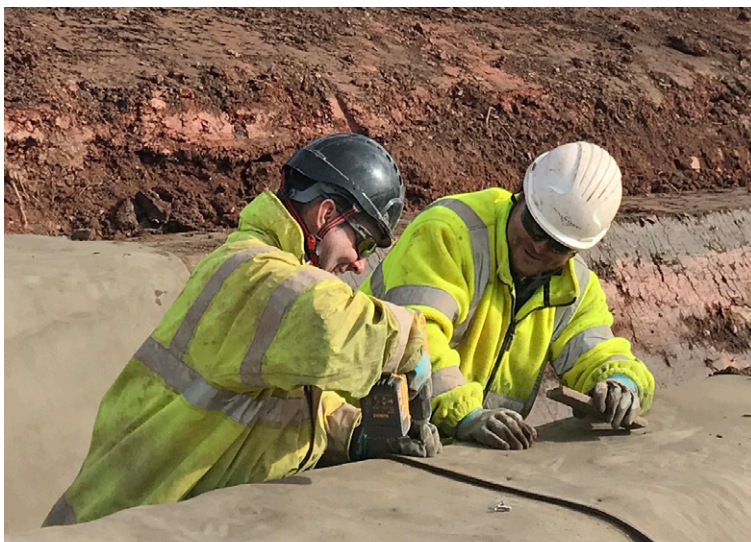
Joining overlaps using stainless steel screws
